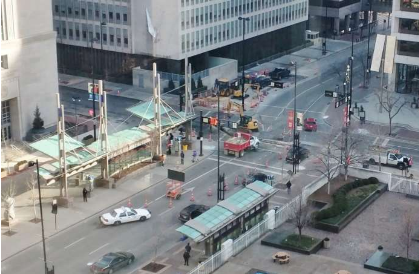
Duke completing manhole construction at 5th and Main Streets
