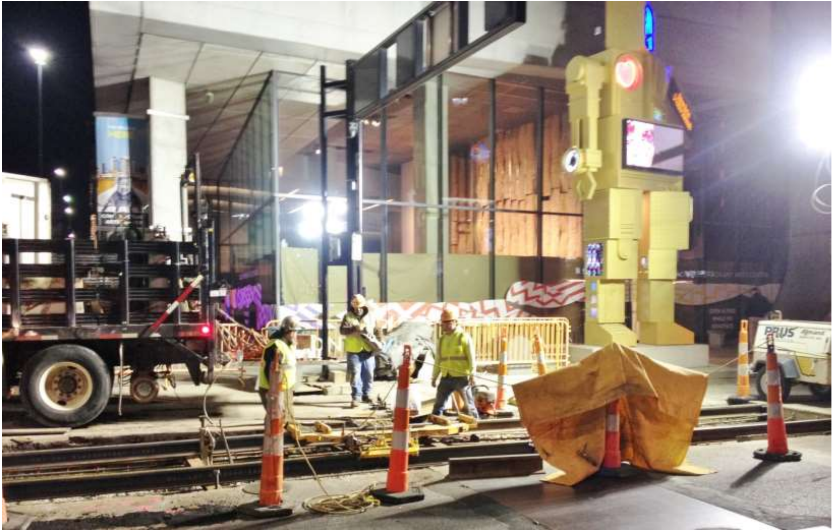
Rail welding for trackwork on Walnut Street adjacent to Metrobot
