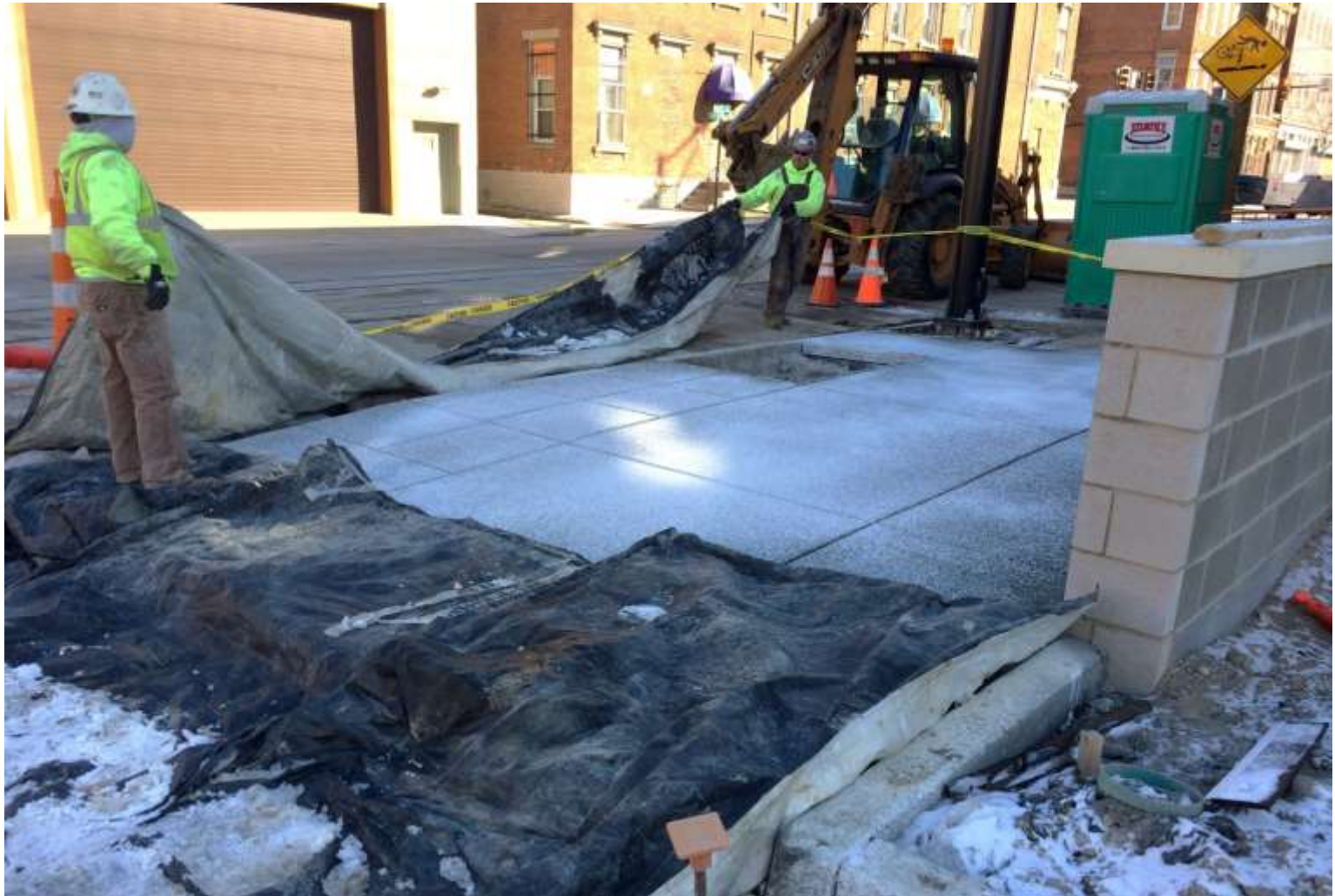
Covering fresh MOF sidewalk concrete with blankets during curing
