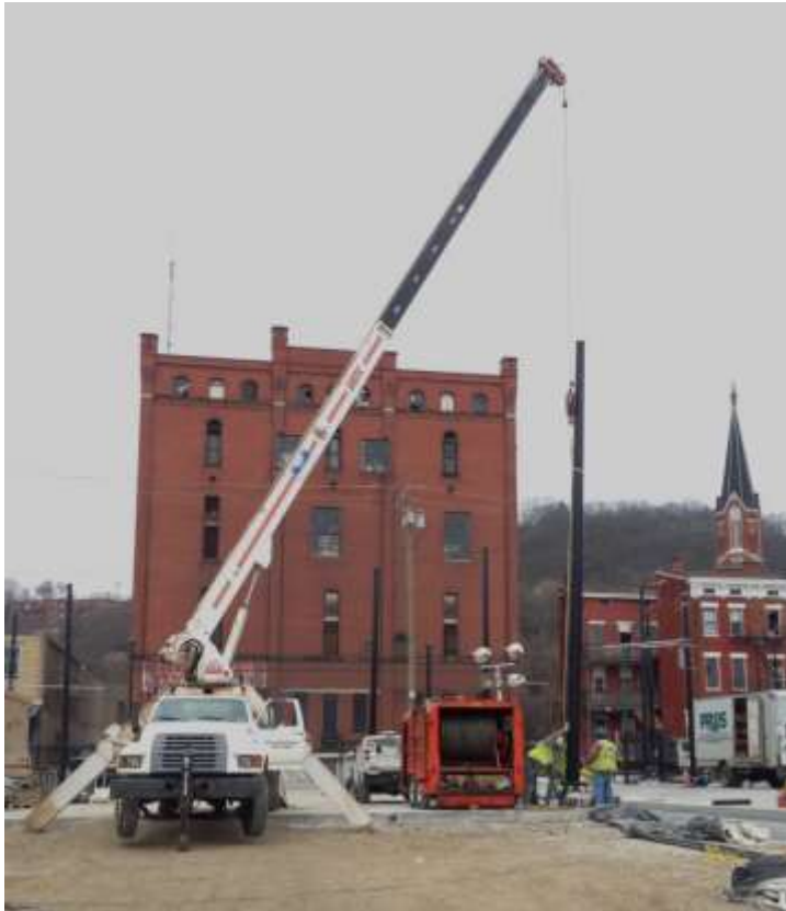
Setting an OCS Pole at the MOF Yard
