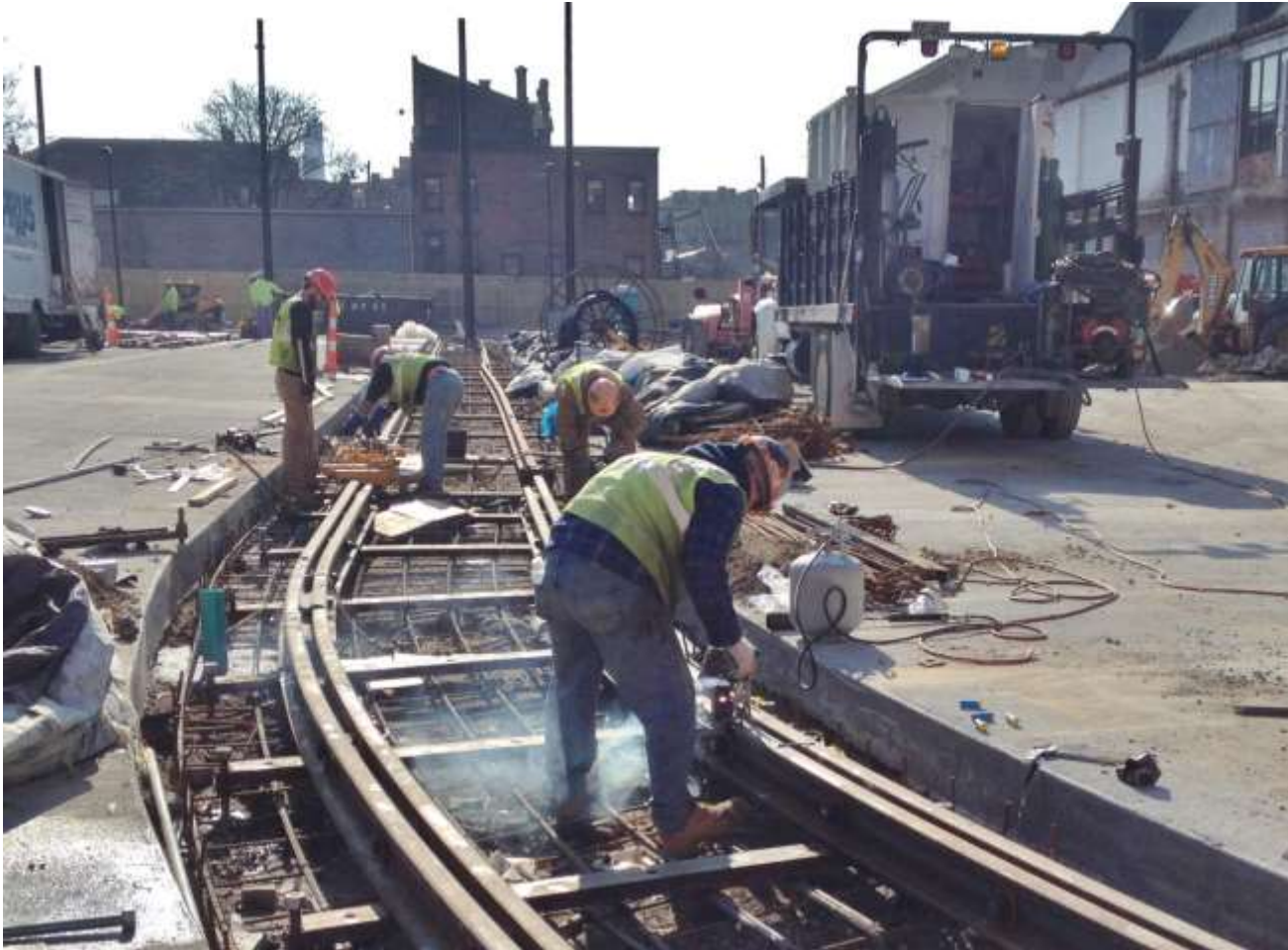
Trackwork at the MOF, thermite welding electrical continuity jumper
