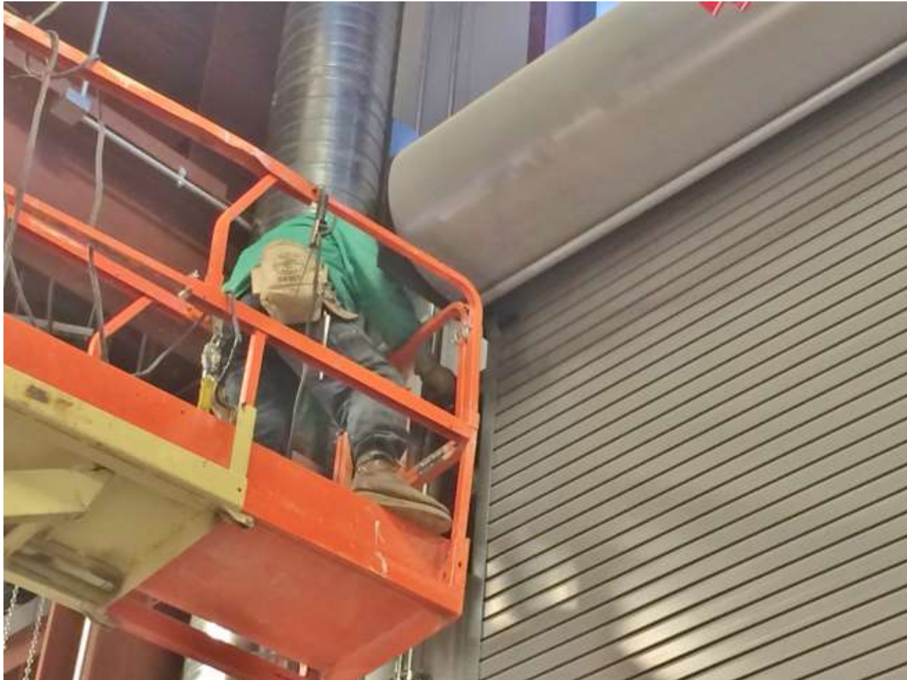
Installing bracket for MOF OCS support
