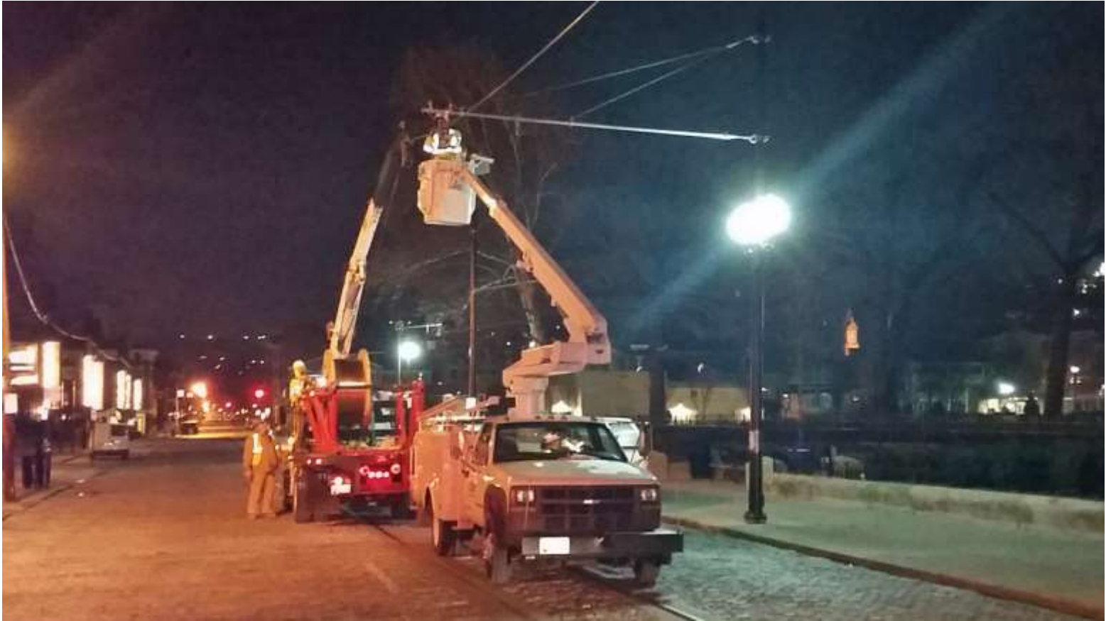
Late night contact wire pull on Elm Street
