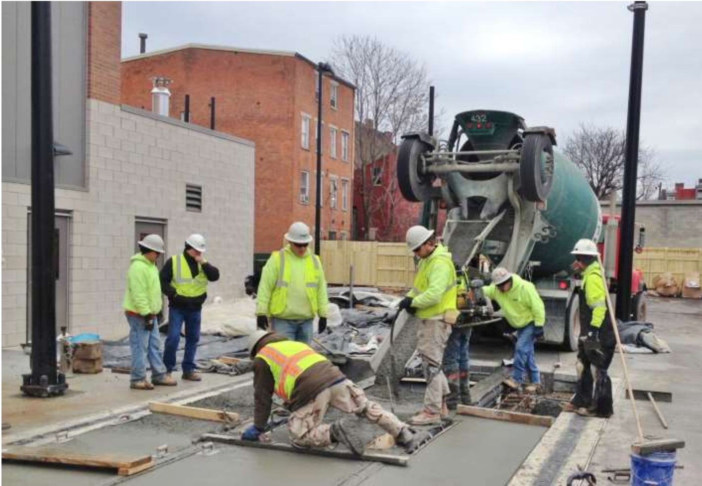
Trackslab concrete placement at the MOF
