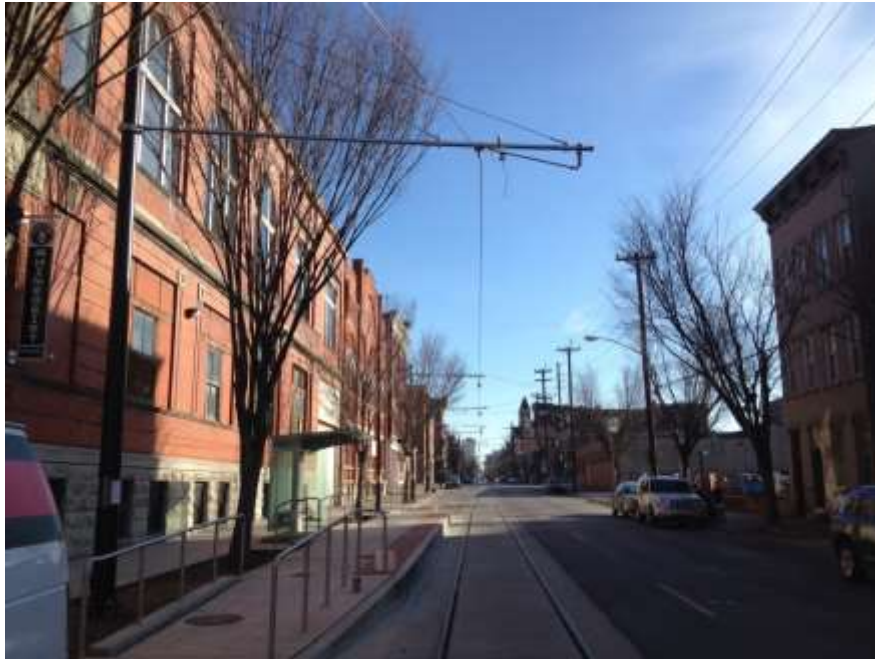
Contact wire on Elm Street after initially 1500 lbs. of tensioning
