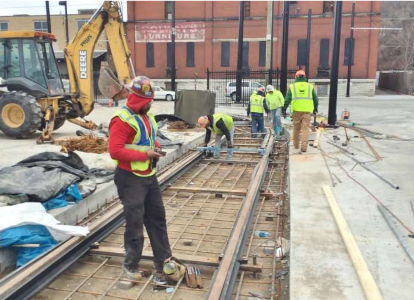
Trackwork at the MOF
