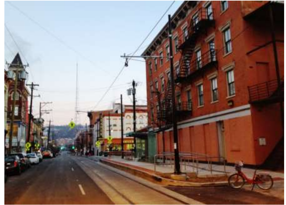
Contact wire on Elm Street after initially 1500 lbs. of tensioning
