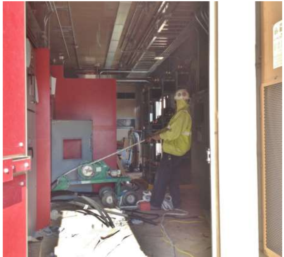
Pulling power cable into TPSS #4 at the MOF Yard
