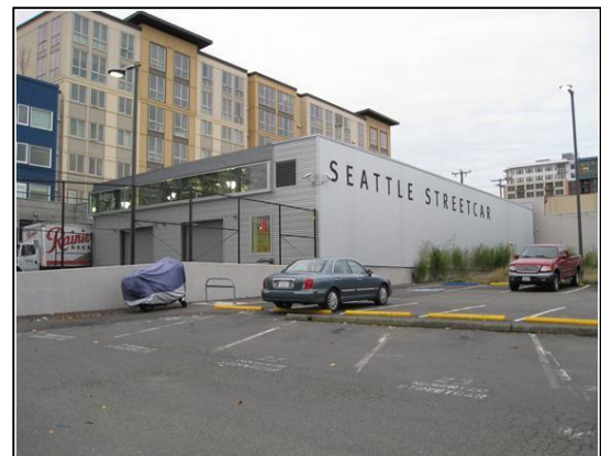
Example of Existing Maintenance and Storage Facility in Seattle, WA
