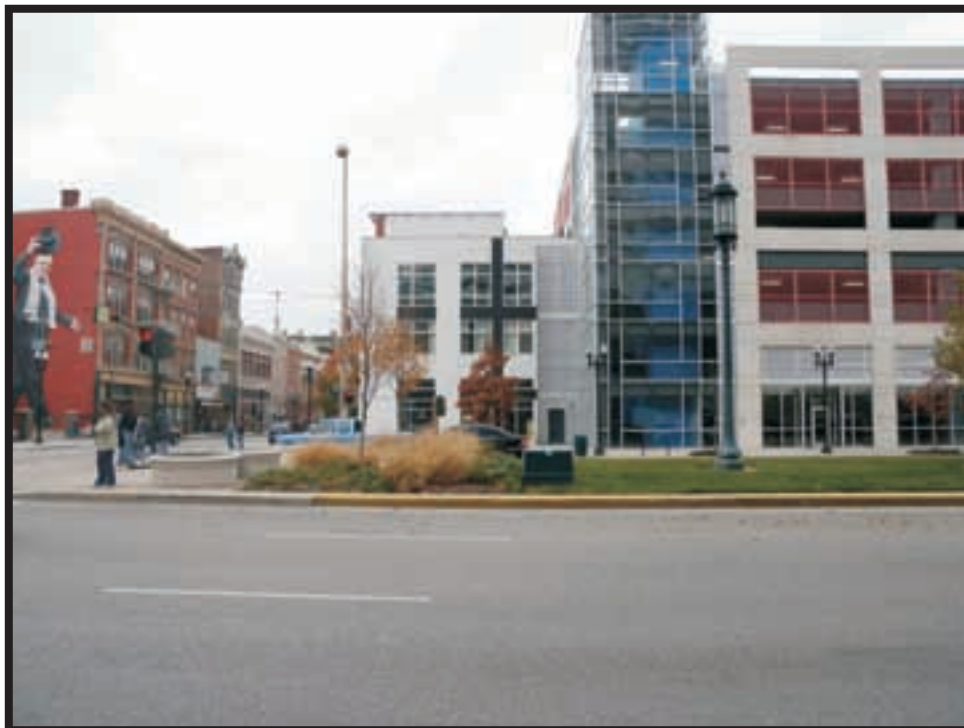
Plate A44. View of Proposed Streetcar Stop Location 14 within the Central Parkway grassy median at Vine Street, facing north.
