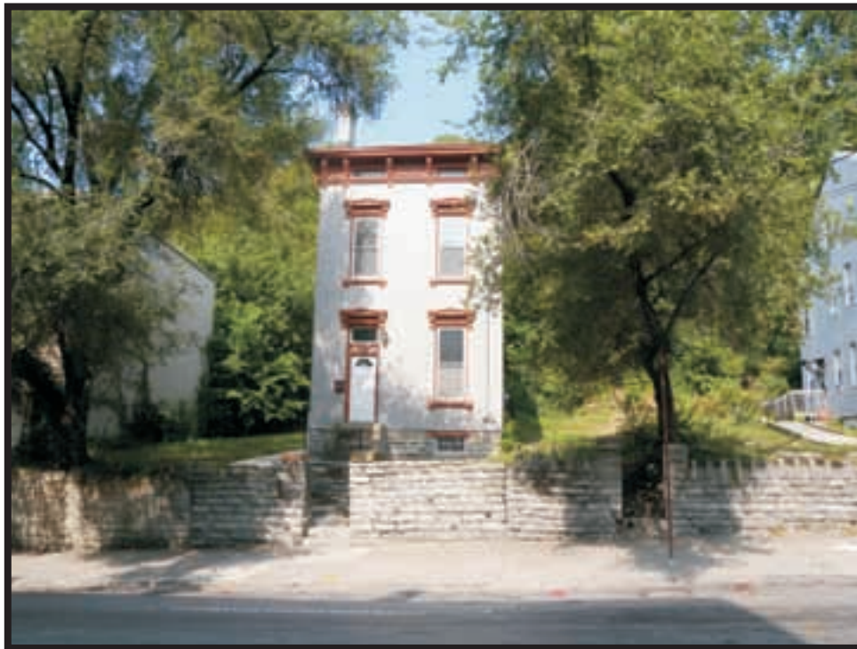
Plate A1. View of 2287 Vine Street, facing west.
