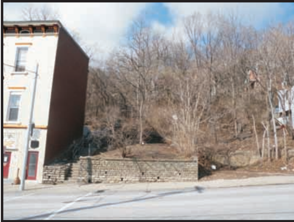
Plate A55. View of the Proposed Substation Location on the north side of Vine Street between Mulberry Street and St. Joe Street.
