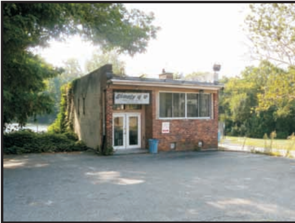
Plate A24. View of 2436 Vine Street, facing southeast.
