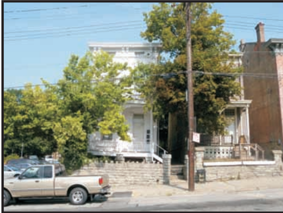
Plate A19. View of 2425 Vine Street, facing west.
