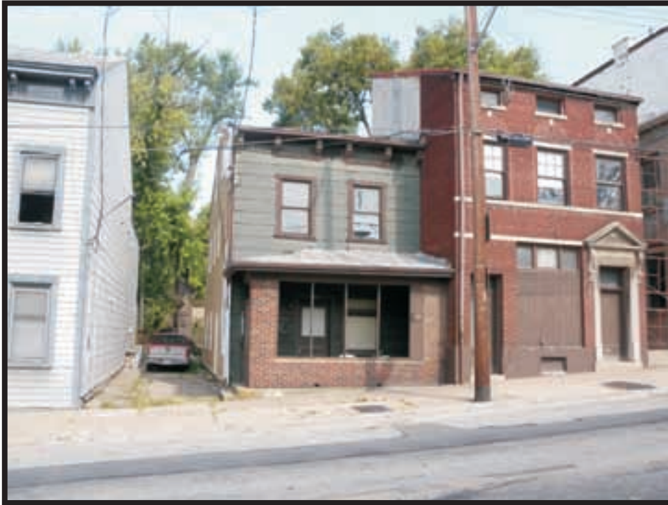
Plate A15. View of 2413 Vine Street, facing west.
