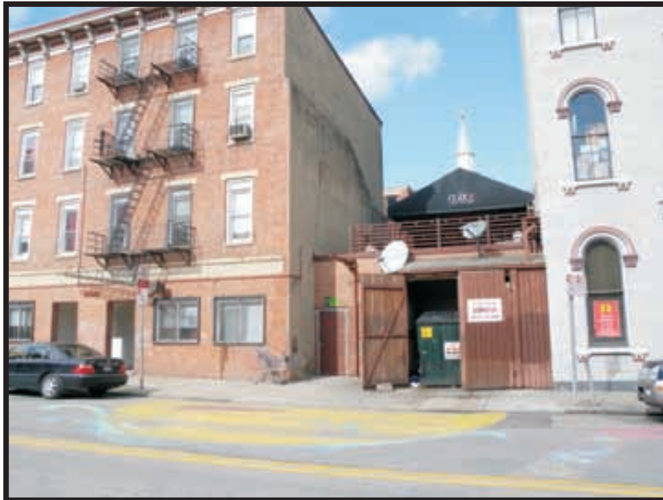
Plate A35. View of Proposed Streetcar Stop Location 5a on 12th Street between Main Street and Clay Street, facing north
