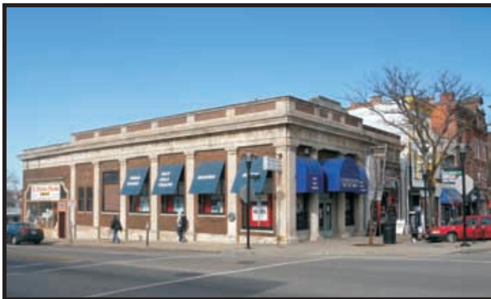
Plate A28. View of 2601 Vine Street, facing northwest.
