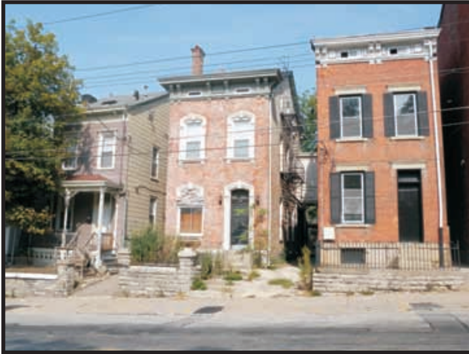
Plate A21. View of 2429 Vine Street, facing northwest.
