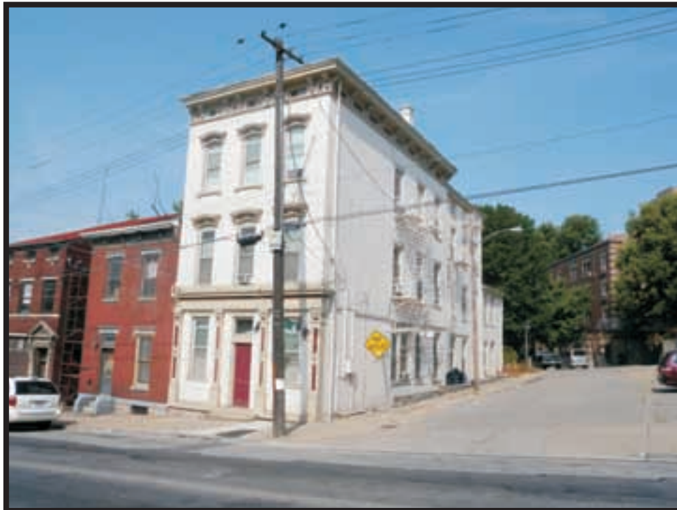
Plate A18. View of 2419 Vine Street, facing west.
