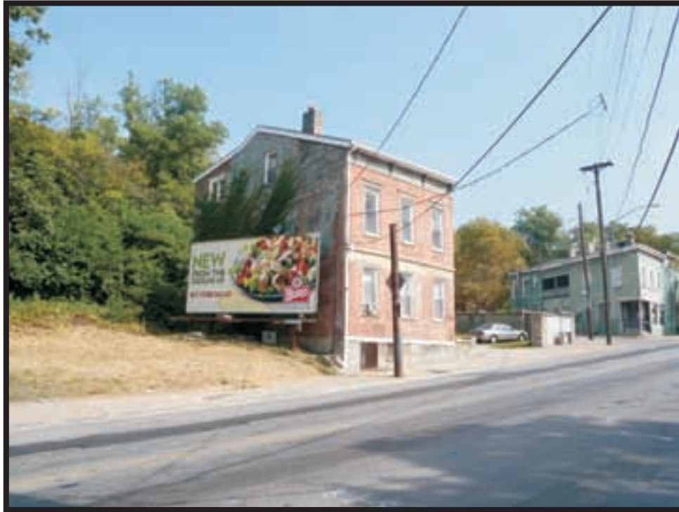
Plate A11. View of 2385 Vine Street, facing northwest.
