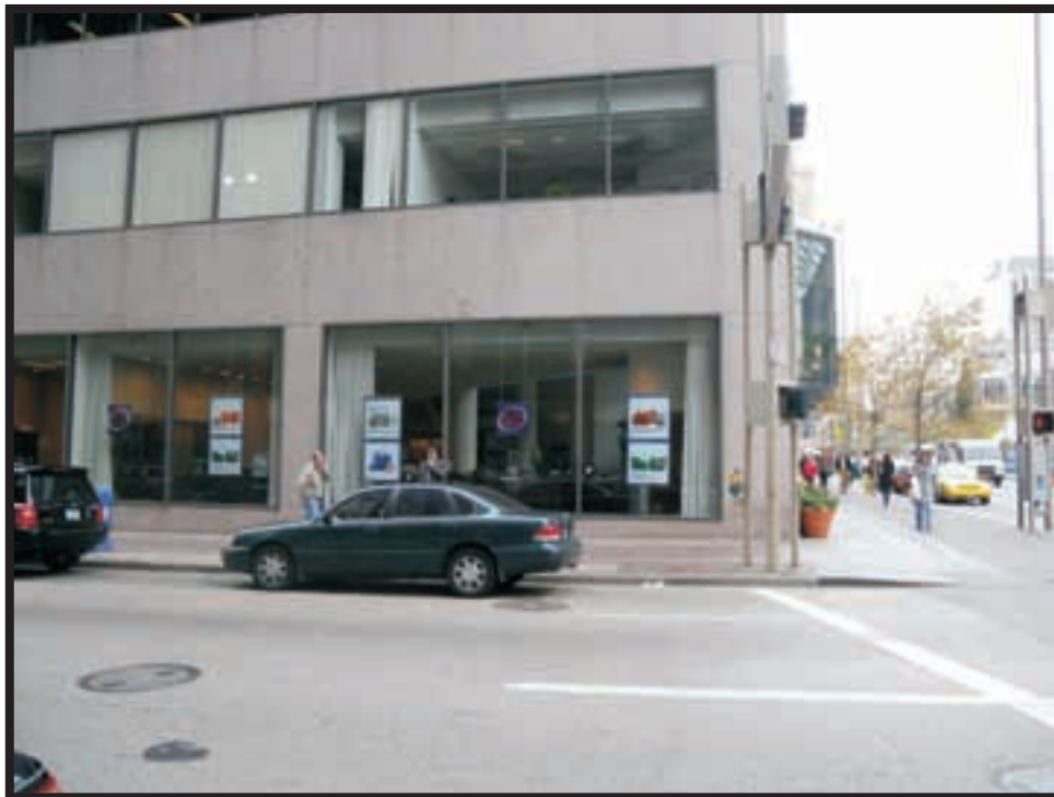
Plate A47. View of the Proposed Streetcar Stop Location 17 at the northwest corner of the Walnut and Fifth Street intersection, facing west.
