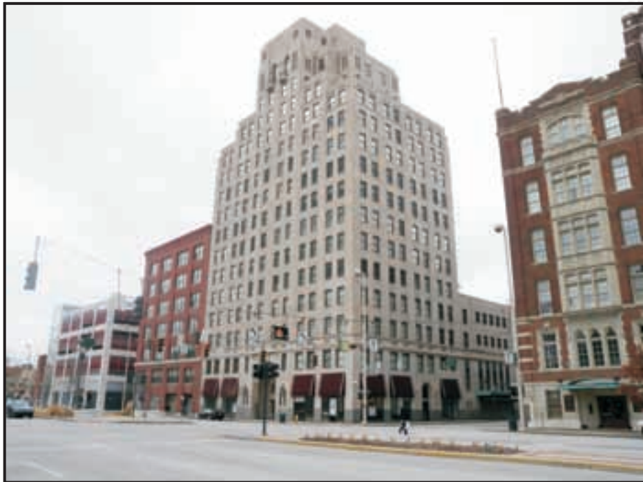
Figure 20. 2011 View of Central Parkway at Walnut Street
