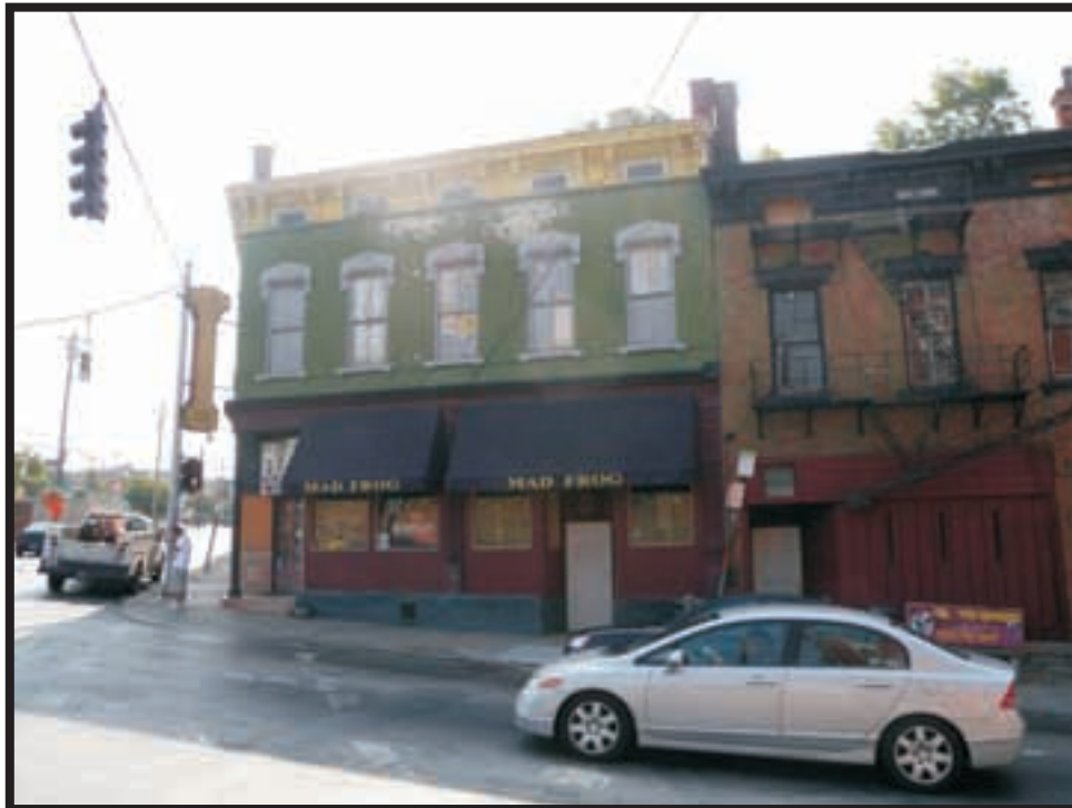
Plate A26. View of 1 McMillan Street, facing southeast.
