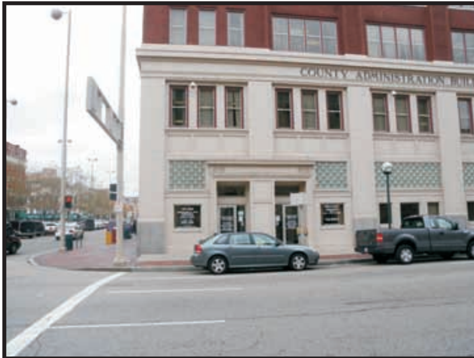
Plate A34. View of Proposed Streetcar Stop Location 5 at the northwest corner of the Court and Main Street intersection, facing west.
