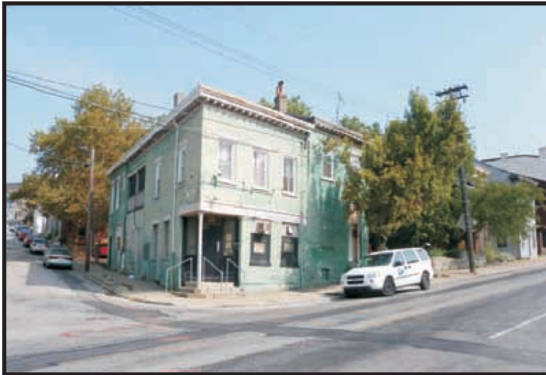
Plate A12. View of 2401 Vine Street, facing northwest.
