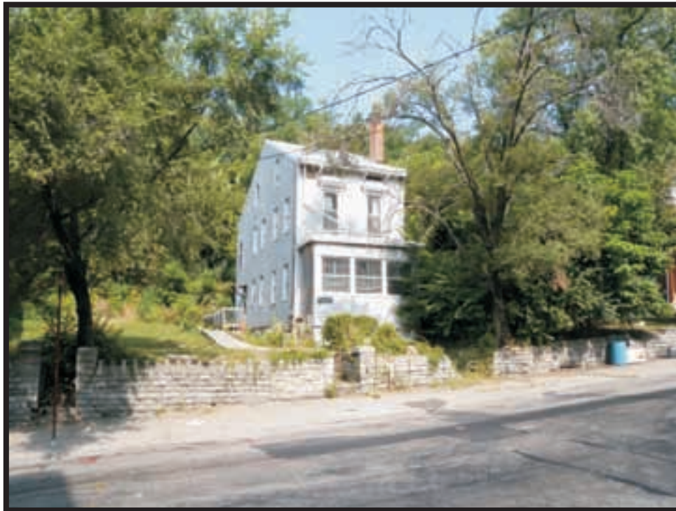
Plate A2. View of 2301 Vine Street, facing northwest.
