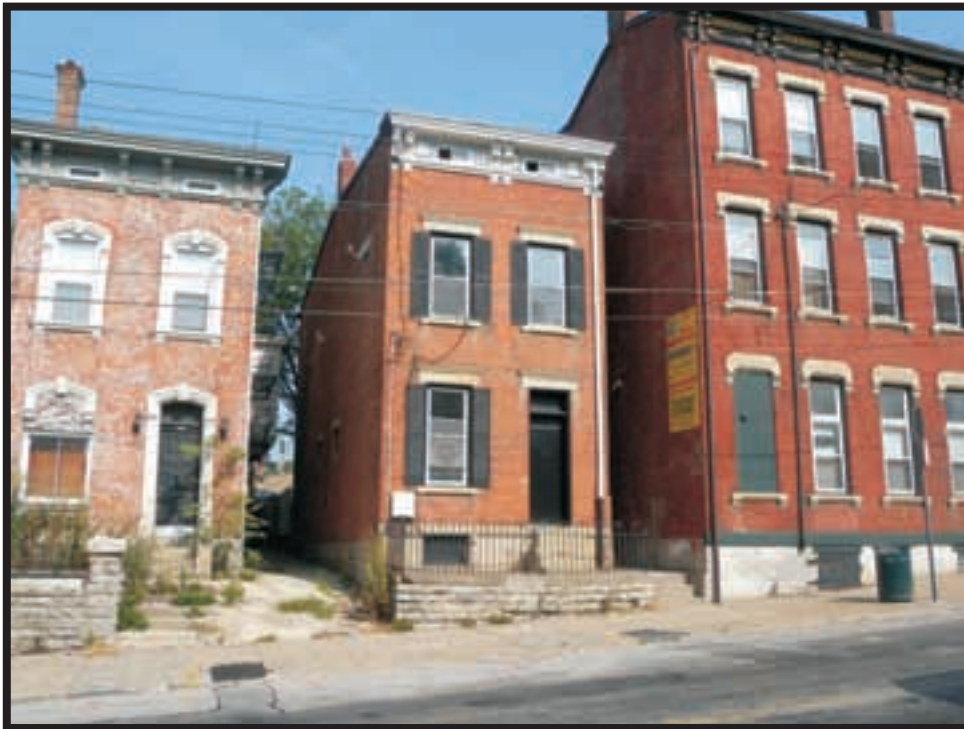
Plate A22. View of 2431 Vine Street, facing northwest.
