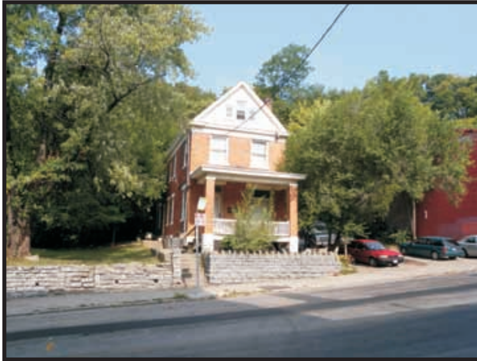
Plate A3. View of 2307 Vine Street, facing west.
