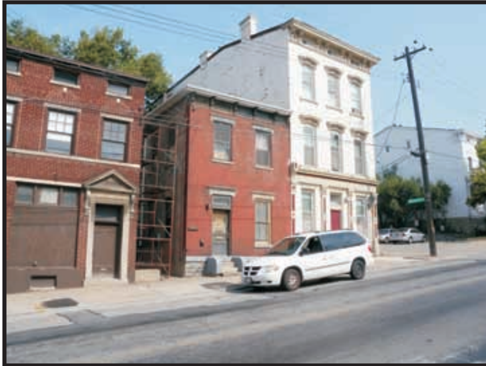
Plate A17. View of 2417 Vine Street, facing northwest.
