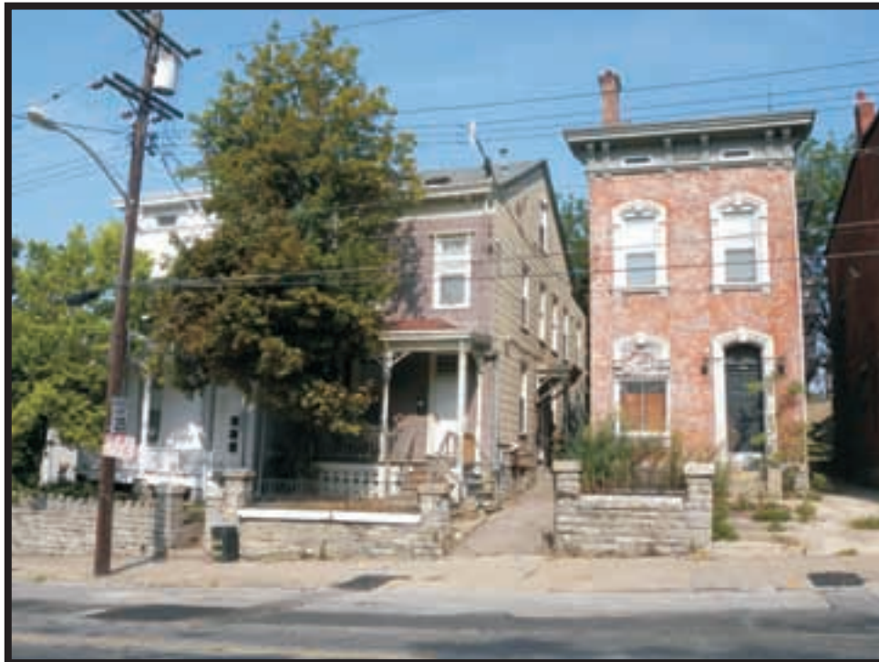
Plate A20. View of 2427 Vine Street, facing west.
