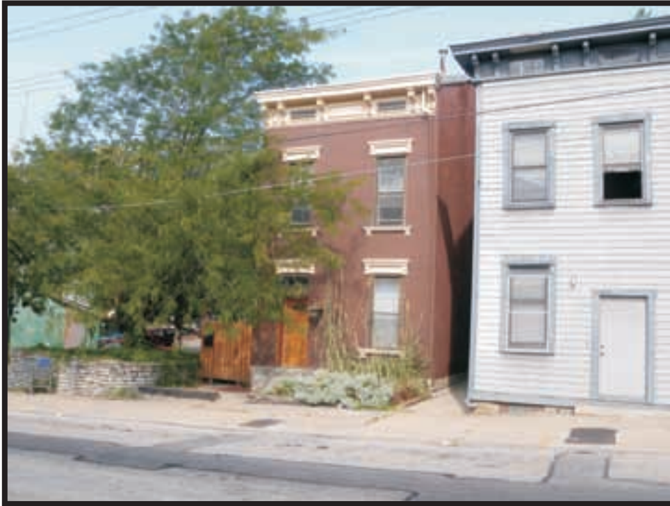
Plate A13. View of 2409 Vine Street, facing west.
