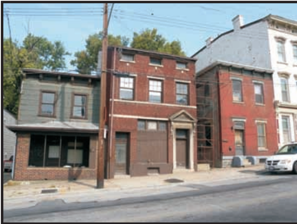
Plate A16. View of 2415 Vine Street, facing northwest.
