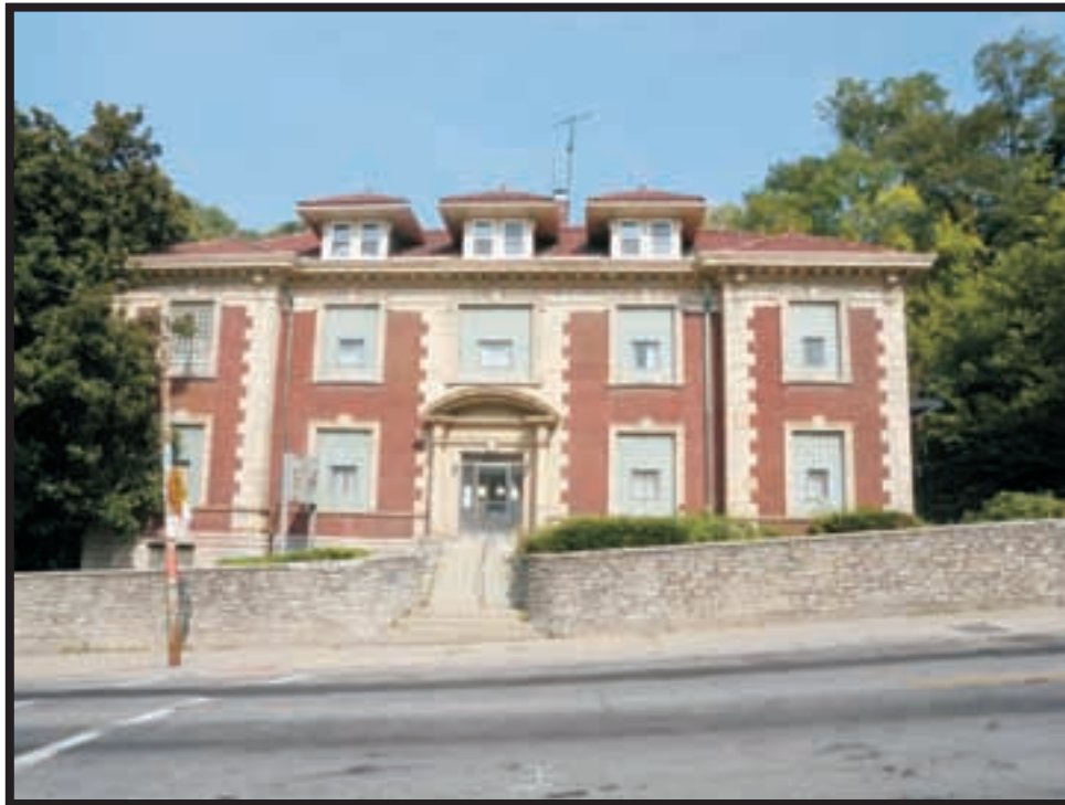
Plate A10. View of 2347-2351 Vine Street, facing west.
