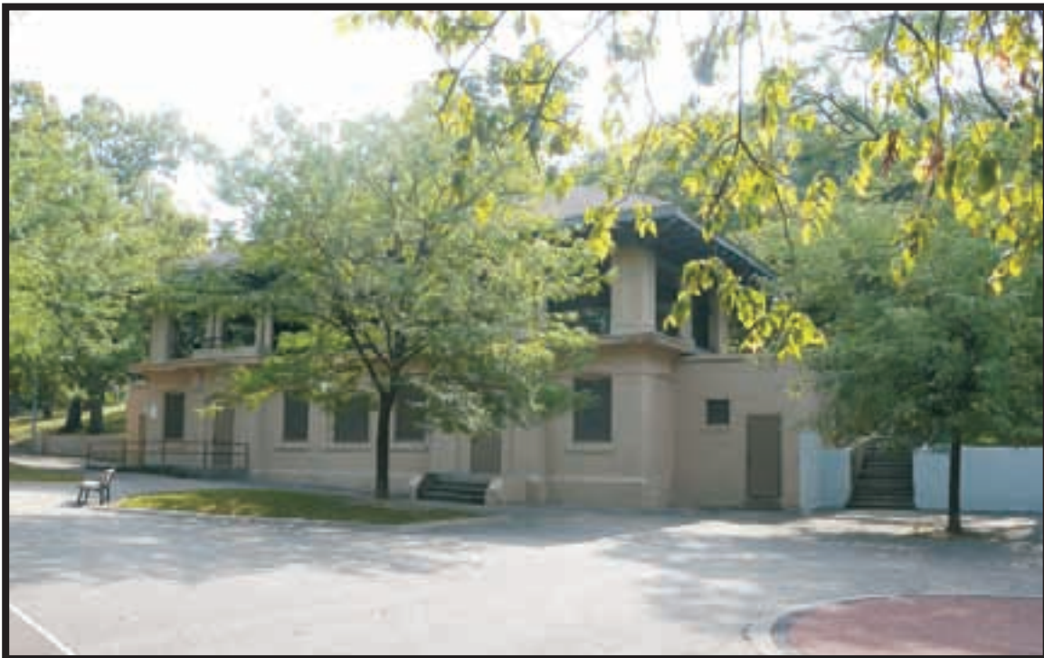
Plate A7. View of 2326 Vine Street, Inwood Park Pavilion, facing northeast.
