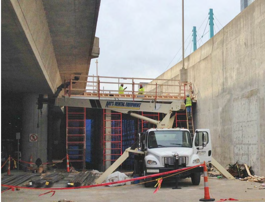
Photo 16: TPSS #2 platform under construction in the Riverfront Transit Center
