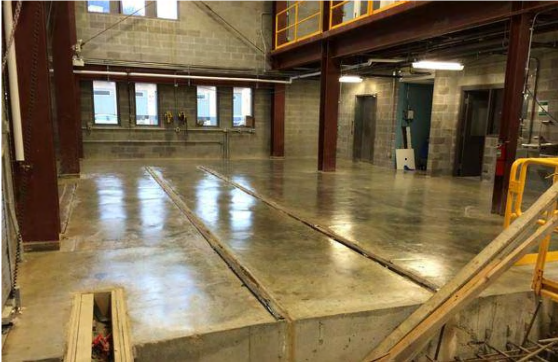
Photo 10: Freshly sealed floor at the MOF truck storage area
