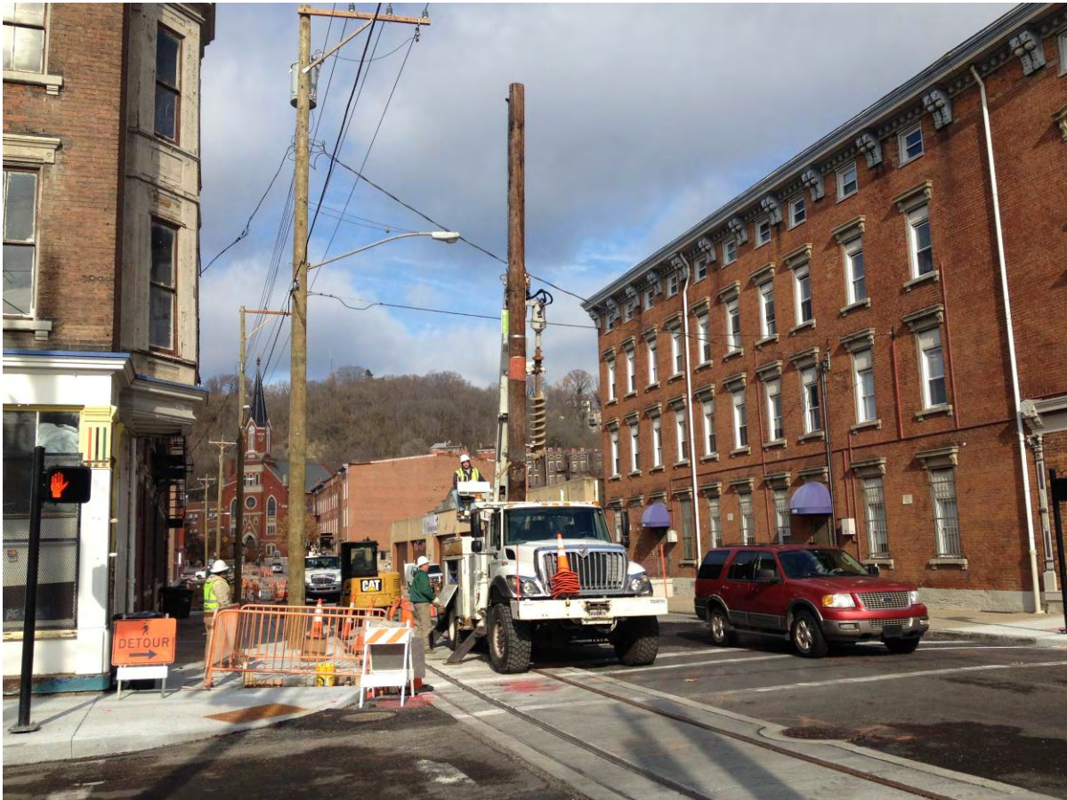
Photo 223: Cincinnati Bell removing old utility pole on Race at Findlay after installing their system underground
