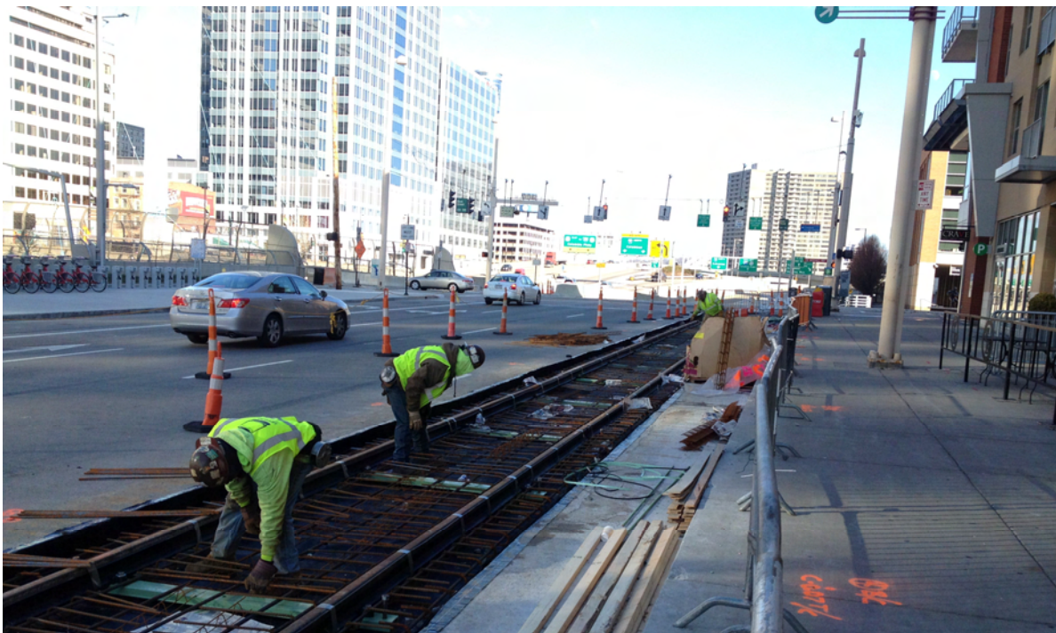
Photo 8: Top mat of rebar goes in prior to concrete on 2nd Street tangent track
