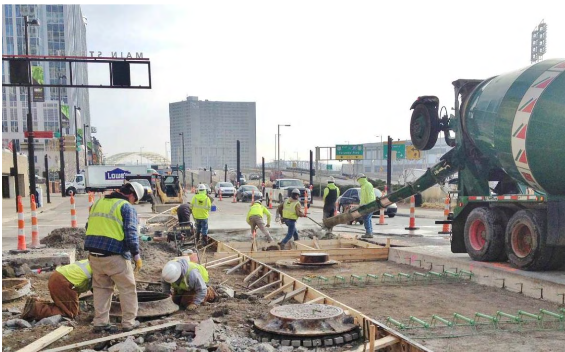
Photo 6: Main St intersection with Third gets new pavement to accommodate track geometry while Duke adjusts manhole for next concrete
