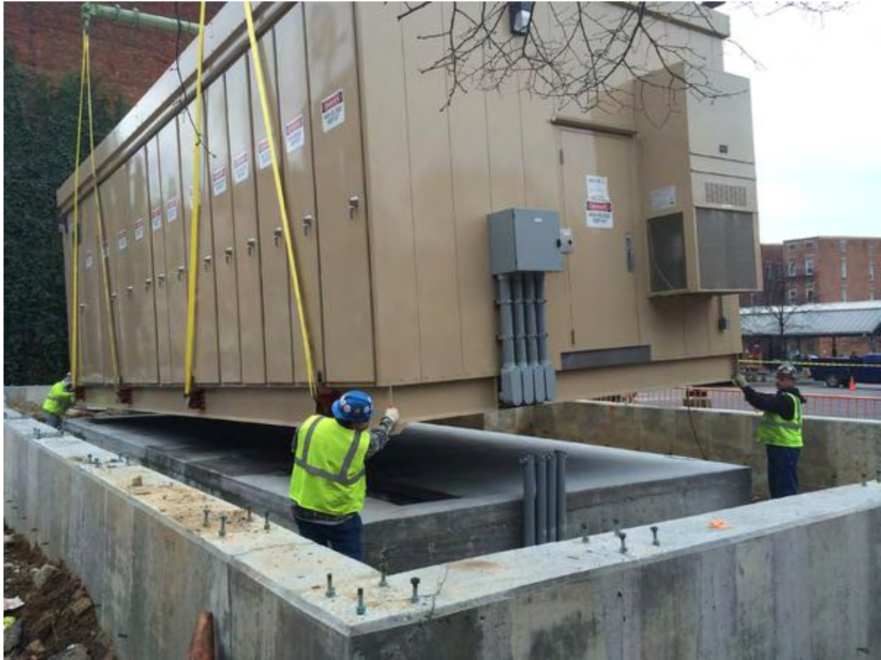
Photo 21: Setting TPSS #2 into final position
