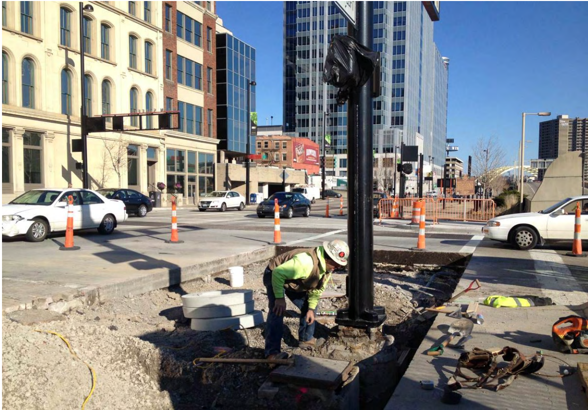
Photo 7: Adjusting pull boxes and manholes in approach slab and sidewalk
