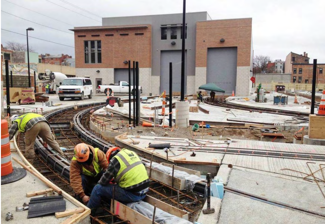
Photo 12: Trackwork at the MOF
