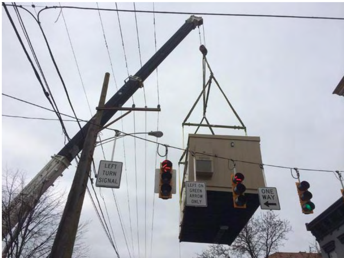
Photo 20: Lifting TPSS #3 over the de-energized Duke overhead electric lines
