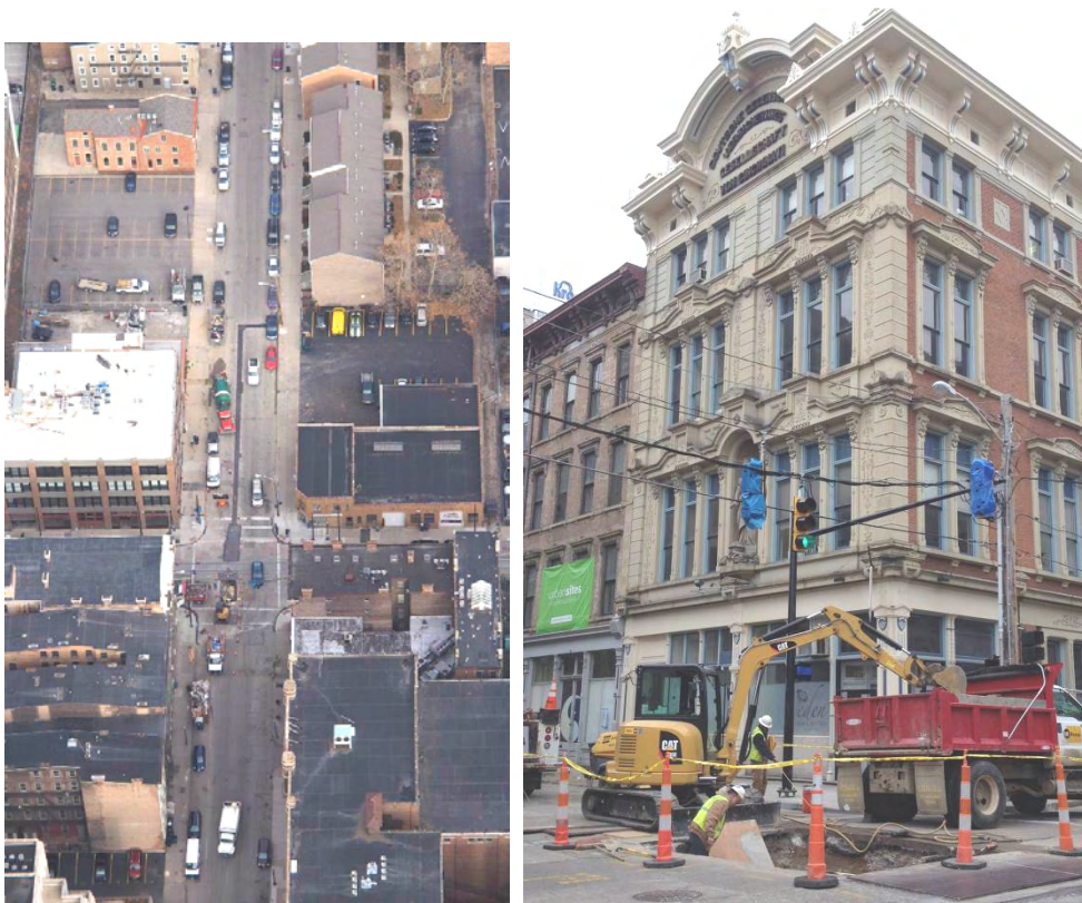
Photo 14 and 15: Conduit tie-in to power TPSS #2 between transmission line to duke Manhole at 12th and Walnut
