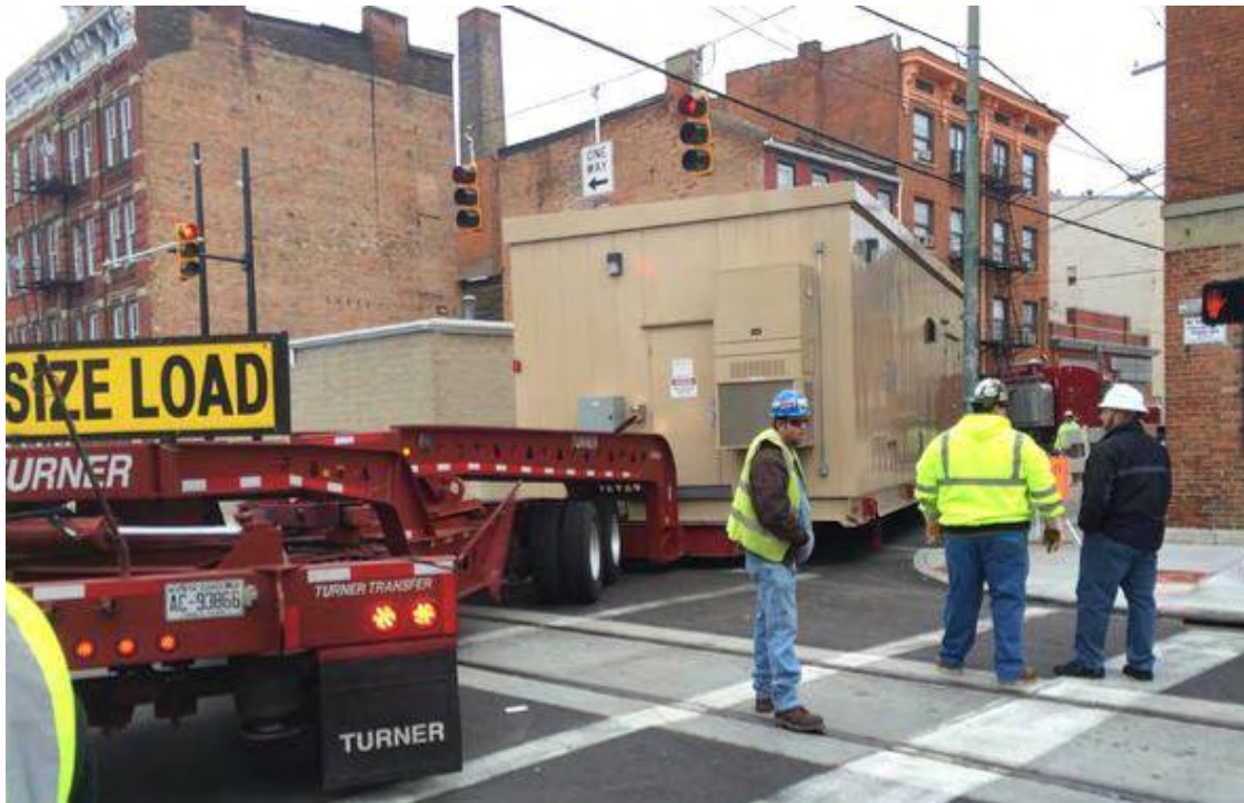
Photo 29: Positioning TPSS 3 to lift into position on Race at Findlay
