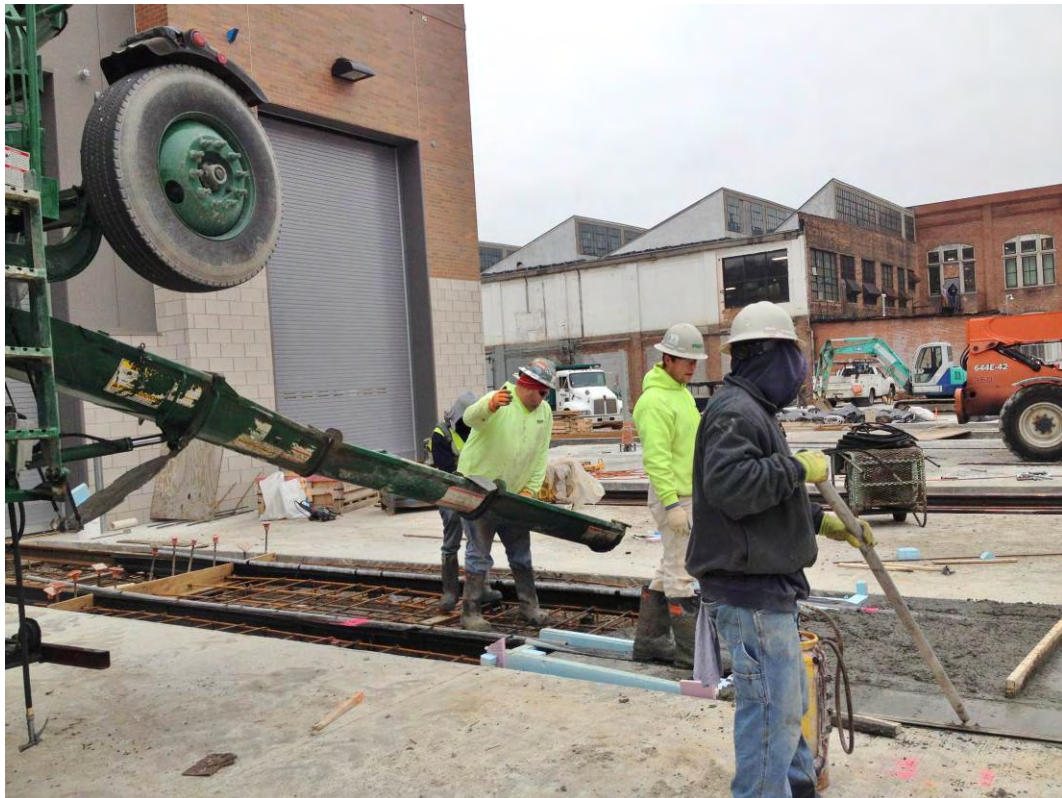
Photo 13: Trackslab concrete at the MOF
