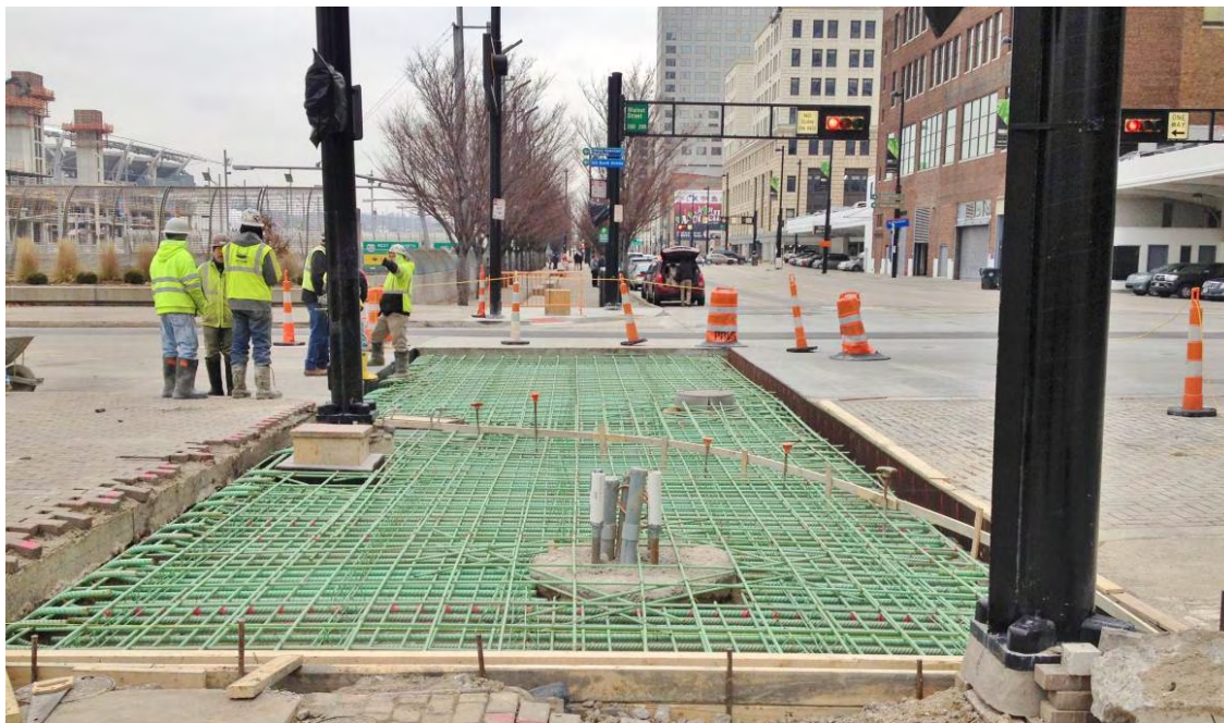
Photo 5: Heavily reinforced approach slab ready for concrete
