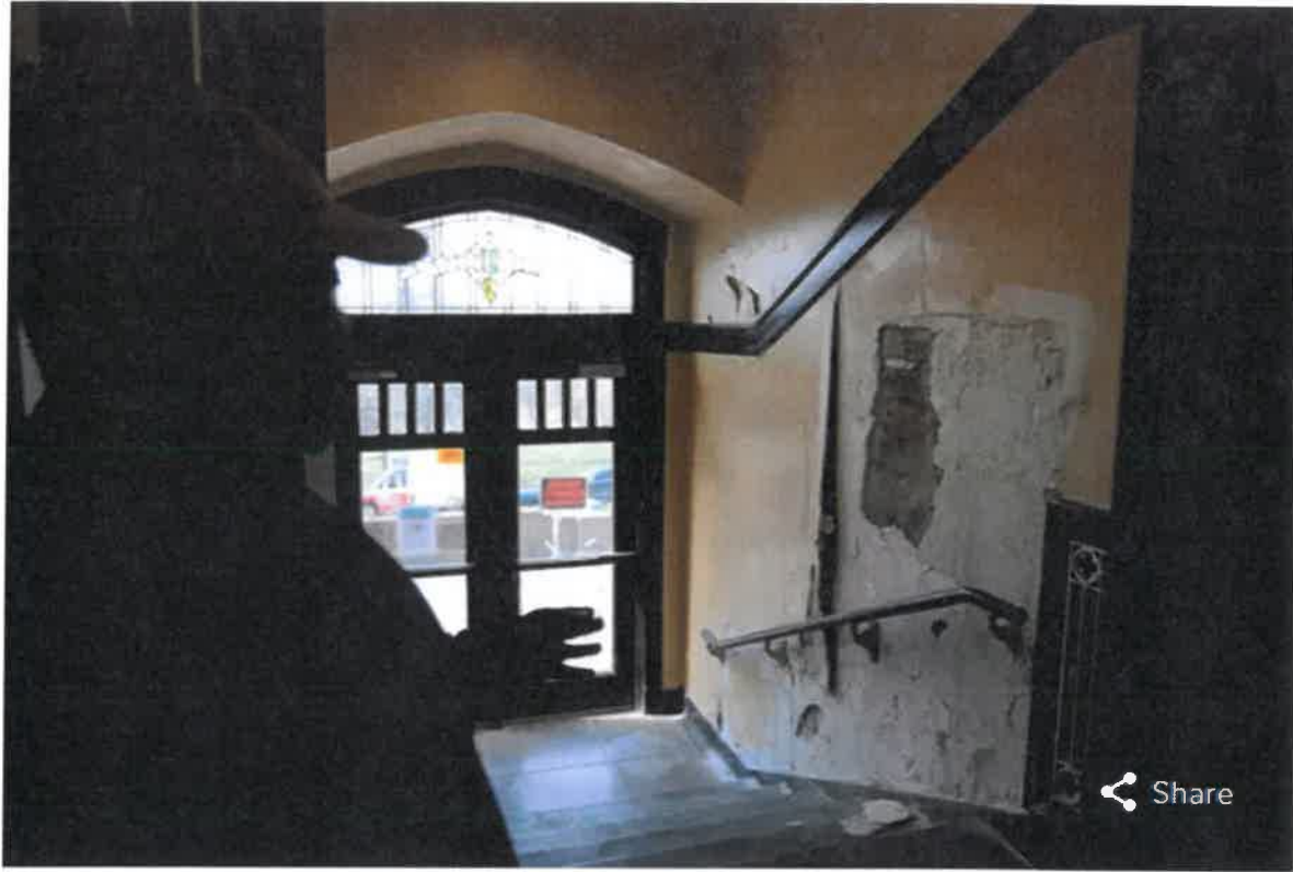
Figure 3: Significant water damage to a hallway within the Hoffman School.
