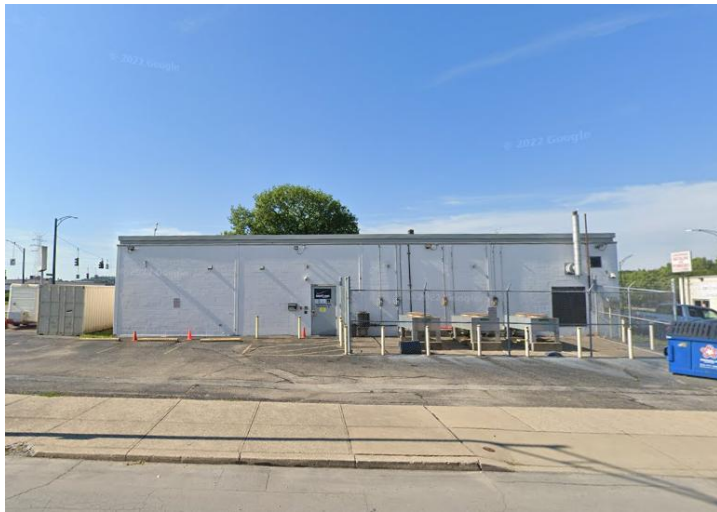
Verizon facility in Cincinnati, OH Total capacity <1 MW
