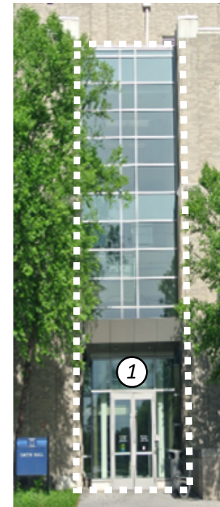
Smith Hall ① Entries with vertical glazing elements above.
