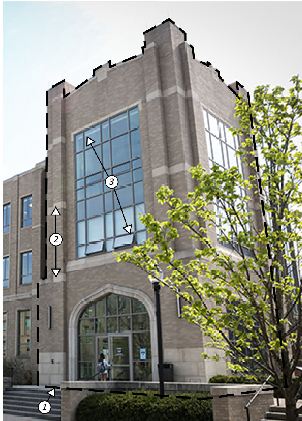
Alter Hall ① Strong tower elements. ② Decorative cast stone banding. ③ Expansive glazing.
