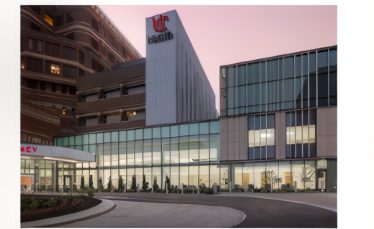
UC Health Surgical Infill, Emergency Department and Tower
