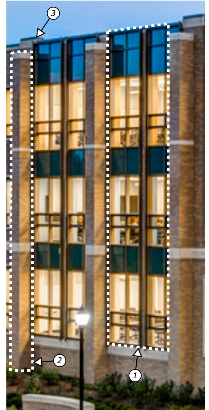
Alter Hall ① Strong vertical elements. ② Vertical fenestration with spandrel glass. ③ Elements projecting above the line of roof coping.
