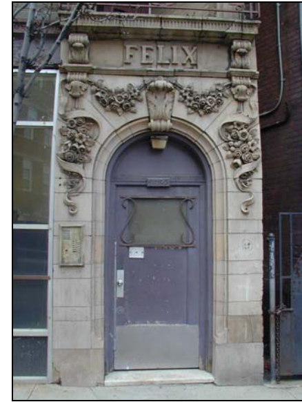
Plate 14: Detail of the Felix Flats Entrance
