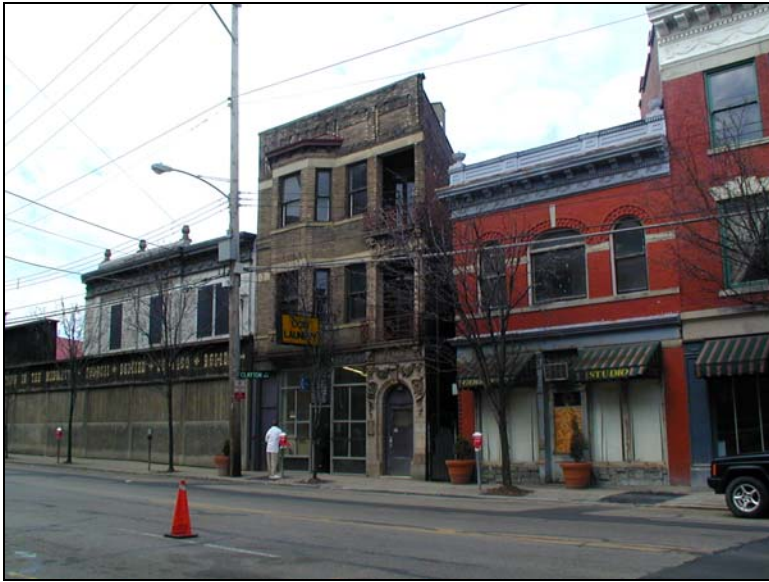
Plate 13: View of 2725, 2723 (Felix Flats) and 2721 Woodburn Avenue
