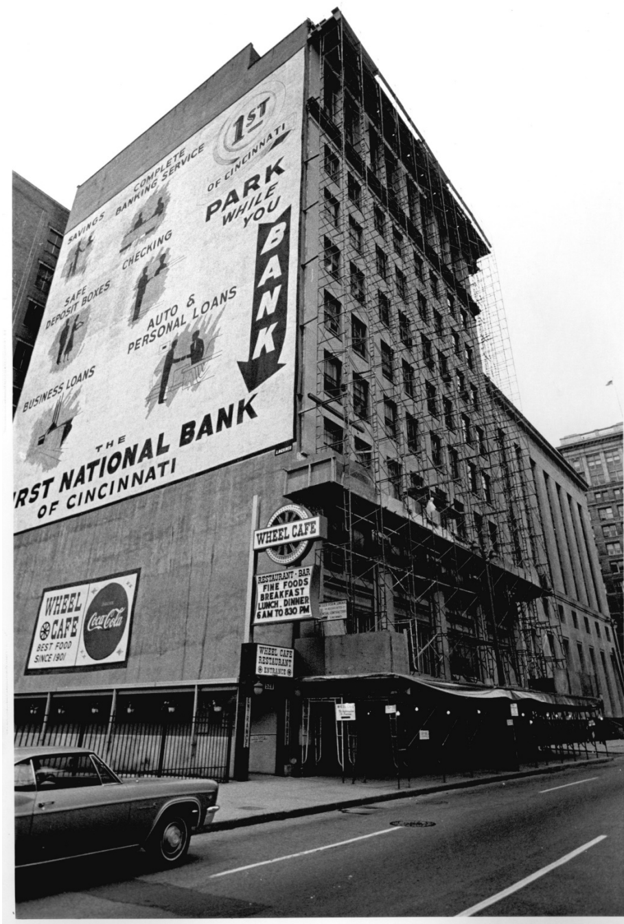
Figure 17. Atlas Bank Building undergoing renovation, 1968
