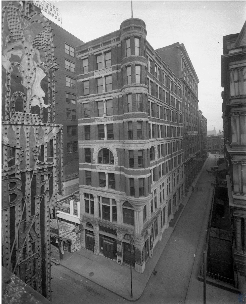
Figure 10. Smith Building/Atlas Bank Building, demolished for present building Lawrence Brand Collection, Kenton County Library
