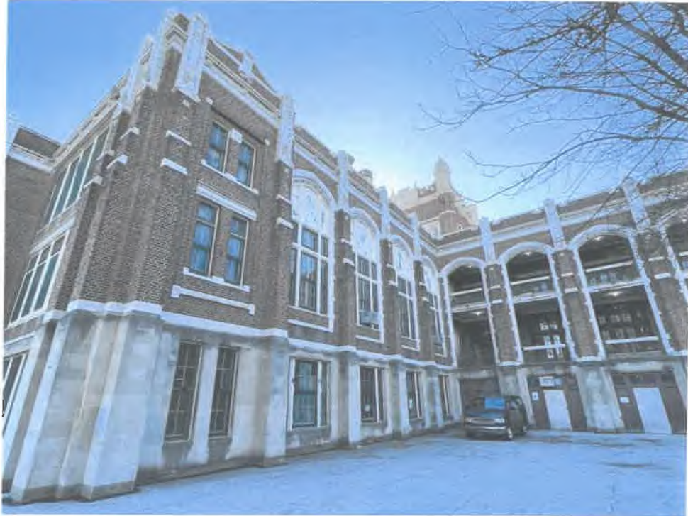
Rear elevations of the school
