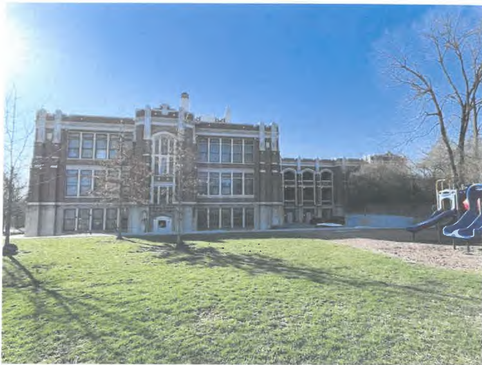
South elevation of the school
