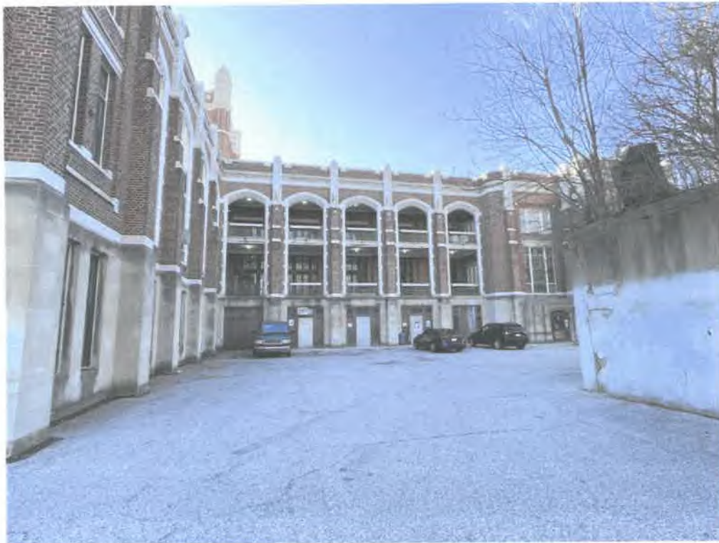
South elevation of the school
