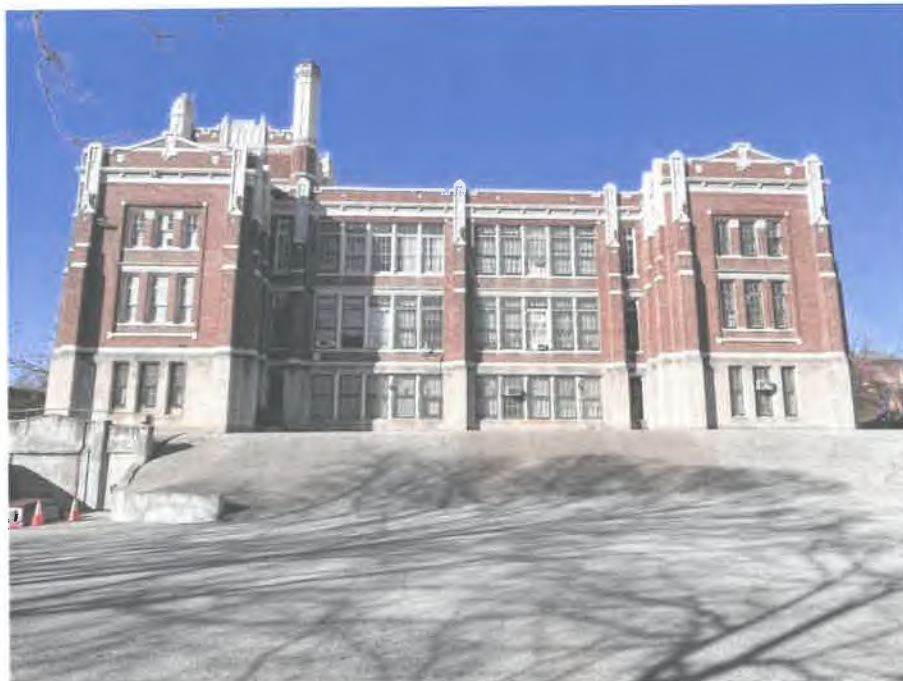
South elevation of the school
