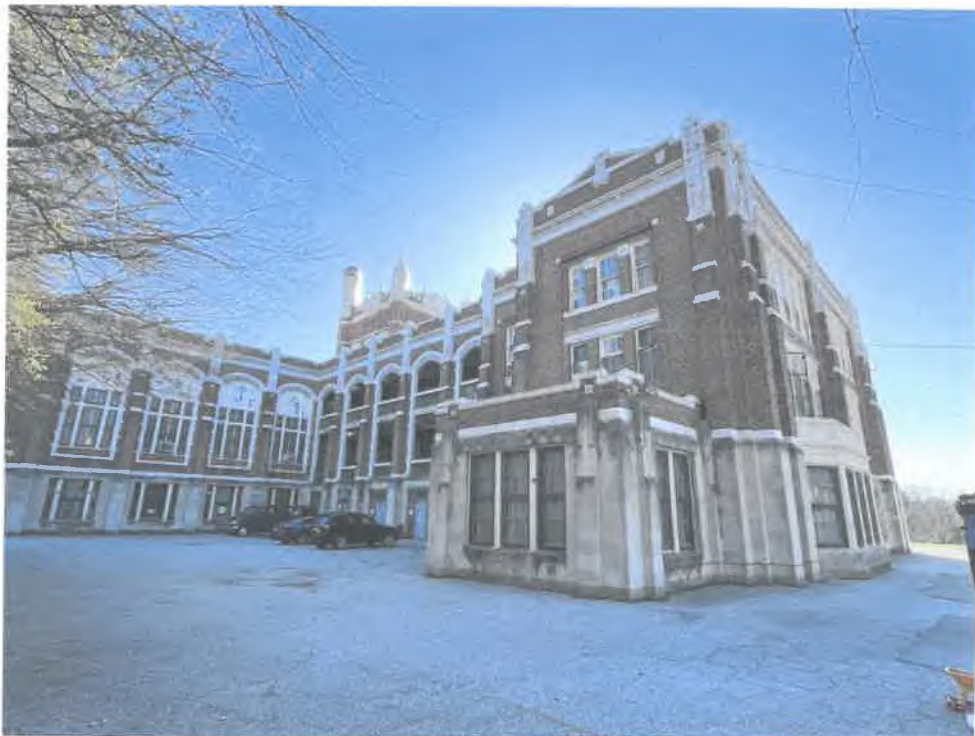
North and rear elevations of the school
