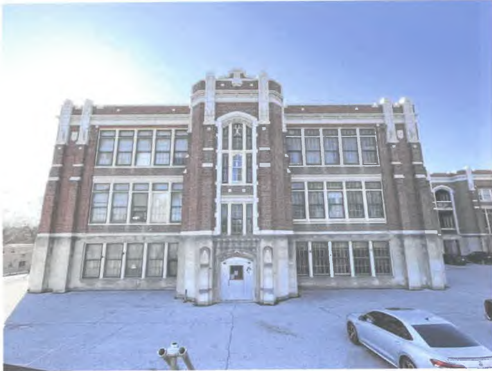
South elevation of the school
