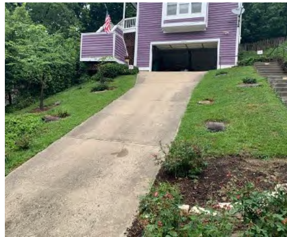
Photo 2: Additional view of existing driveway
