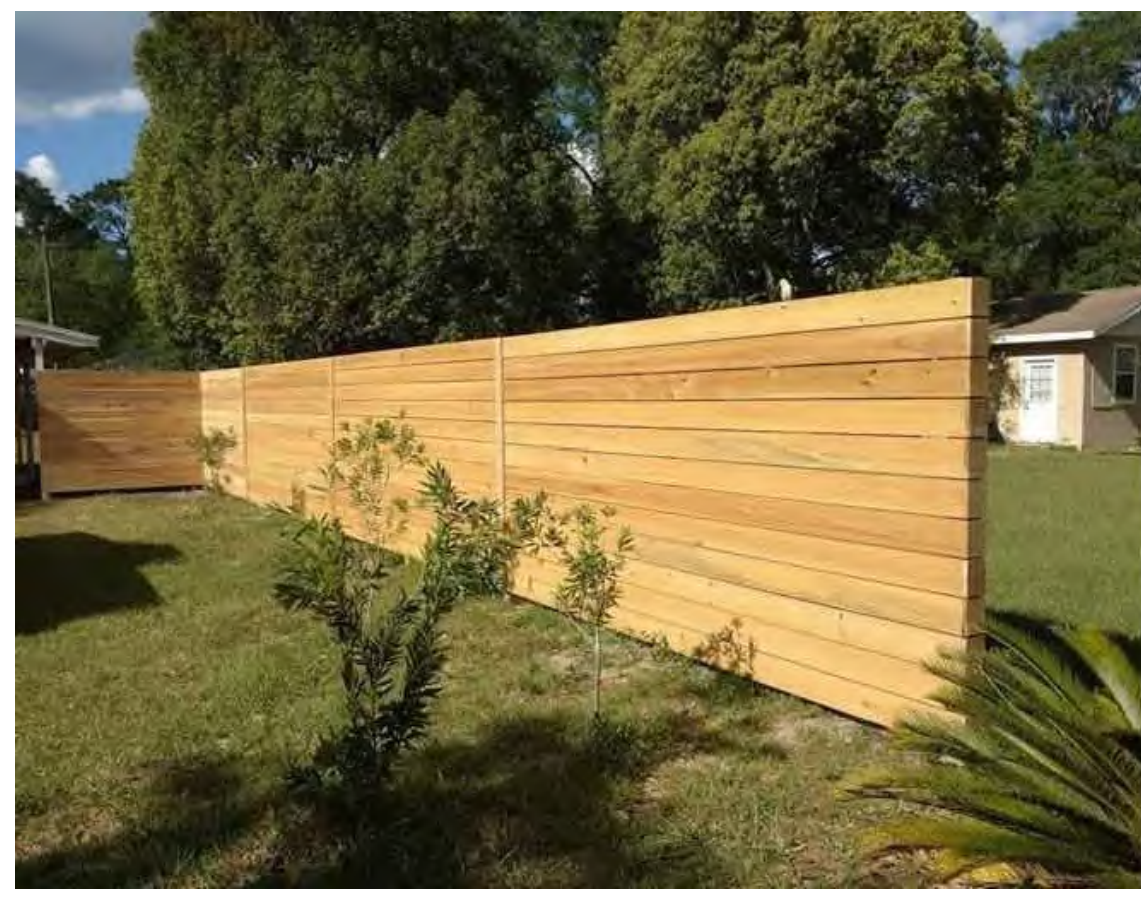
EXAMPLE OF SLAT CONFIGURATION / SPACING (UNFINISHED)
