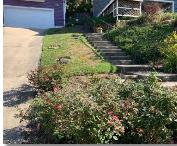
Photo 4: View of gas and sewer utilities in side yard
