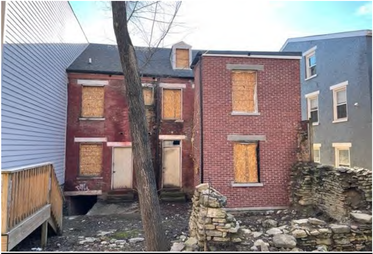
Figure 3. 226 Mohawk Street, rear elevation, ca. 2024, facing south. Image provided by applicant.
