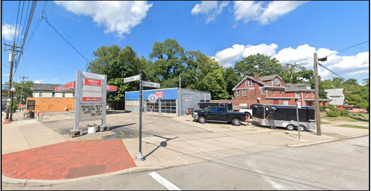
Figure 2: Image of subject property from August 2022. Image from Google.
