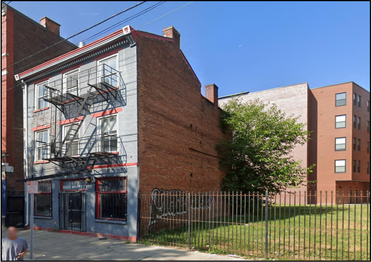
Figure 2. Front (east) and side (north) view of 1607 Race St. Image from Google.
