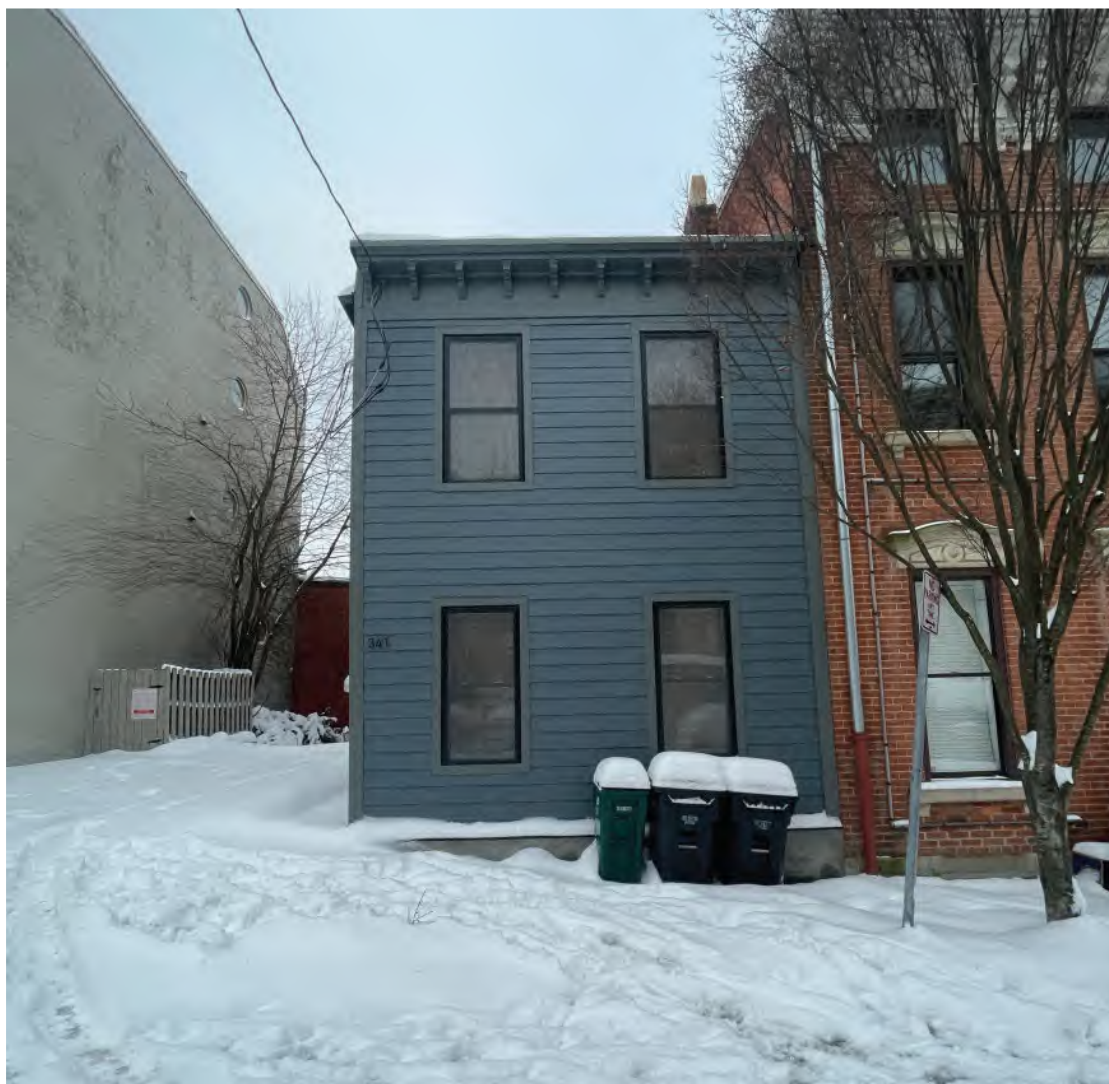
Figure 9: Current Front facade of 341 Milton St.
