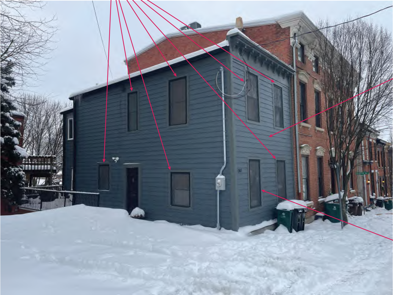
Figure 8: Current Front and Side facade of 341 Milton St.
