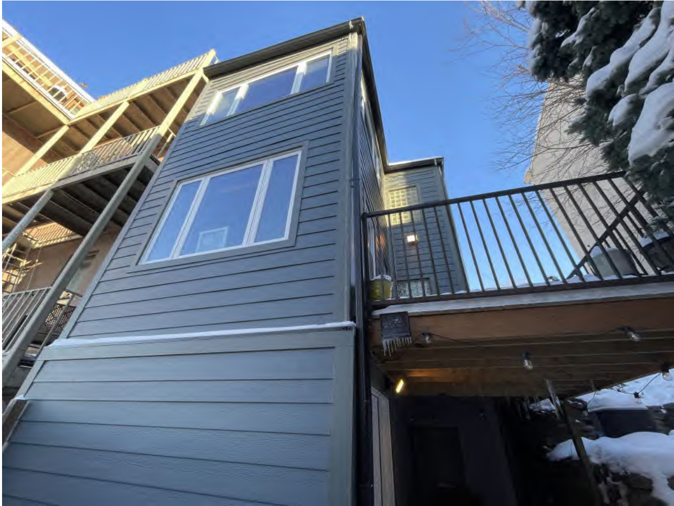
Figure 10: Only new work is siding. Old windows shown.
