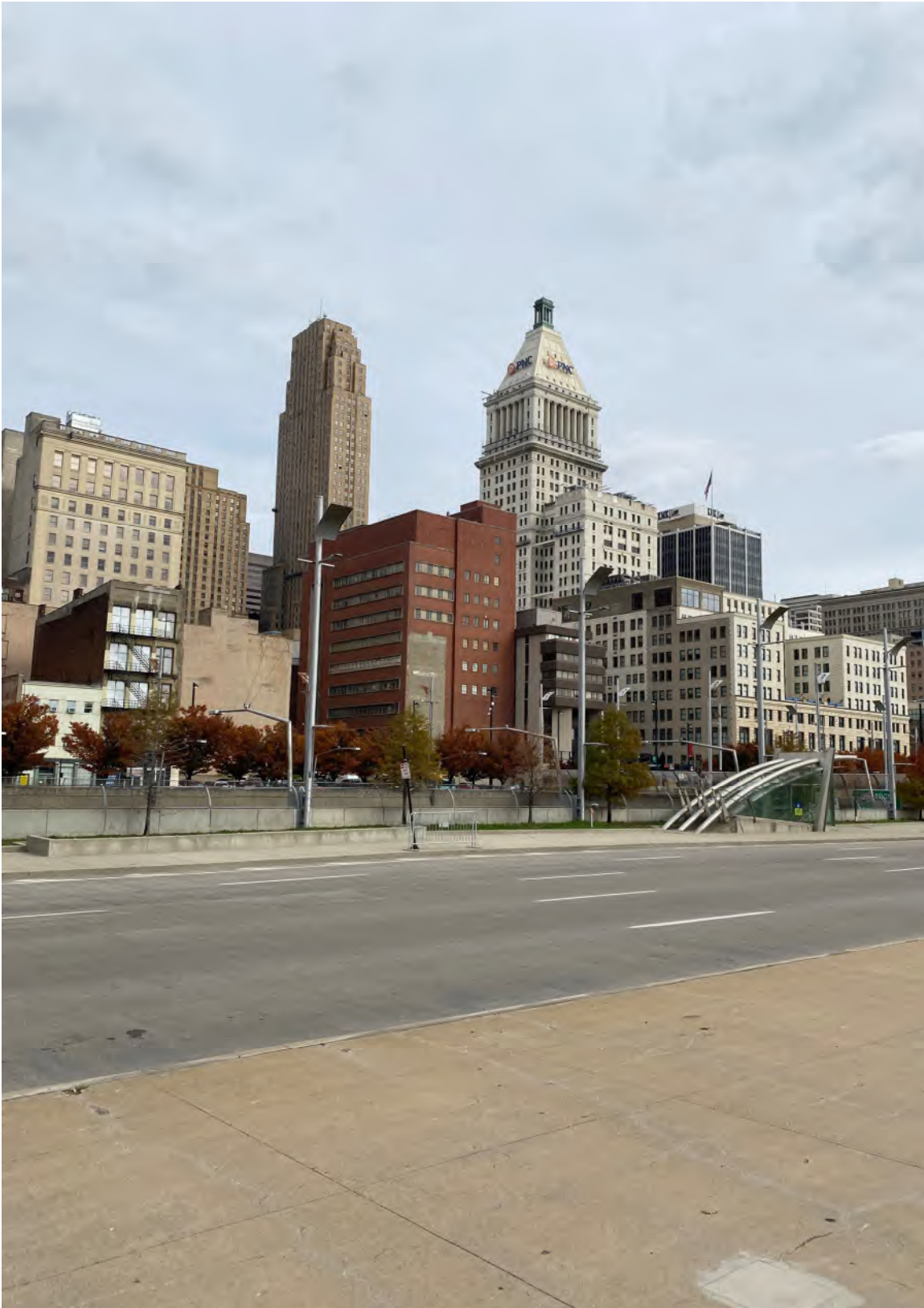
11. Exterior, West and South Elevations, perspective view looking northeast across 2nd Street.
