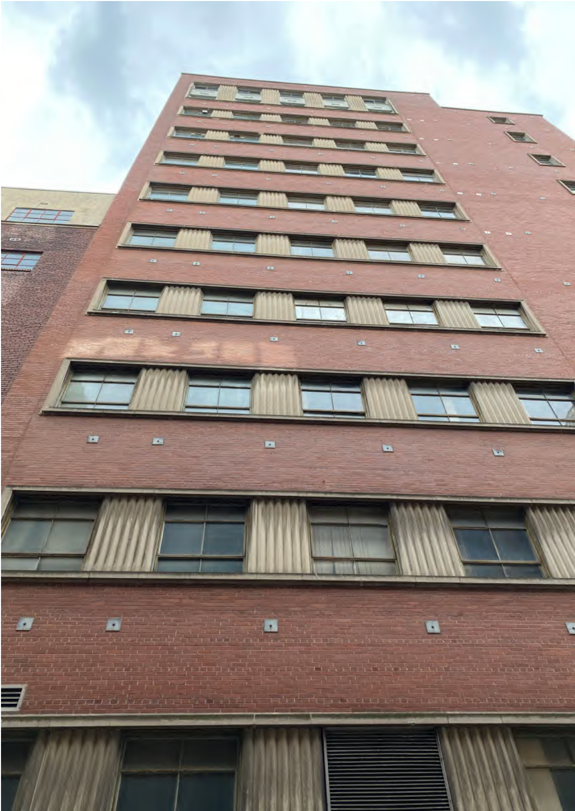
9. Exterior, North Elevation, view looking south.
