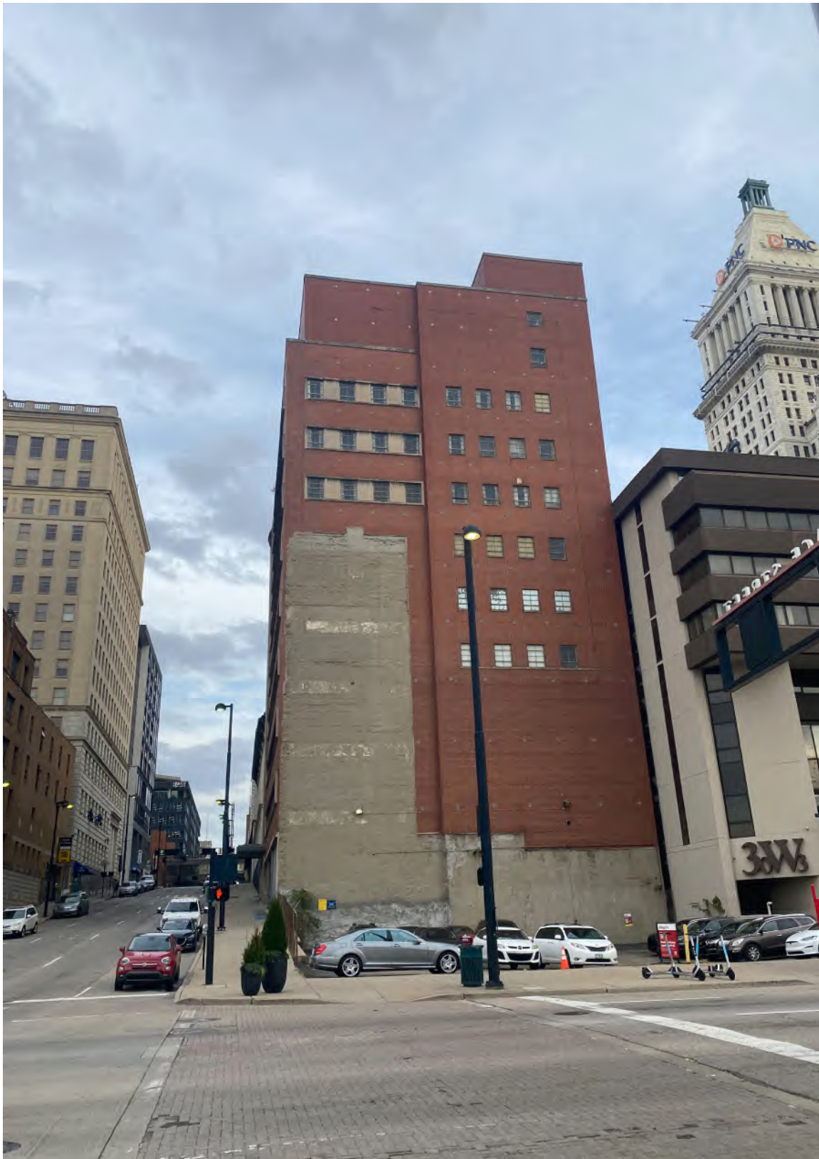
7. Exterior, South Elevation, view looking north.
