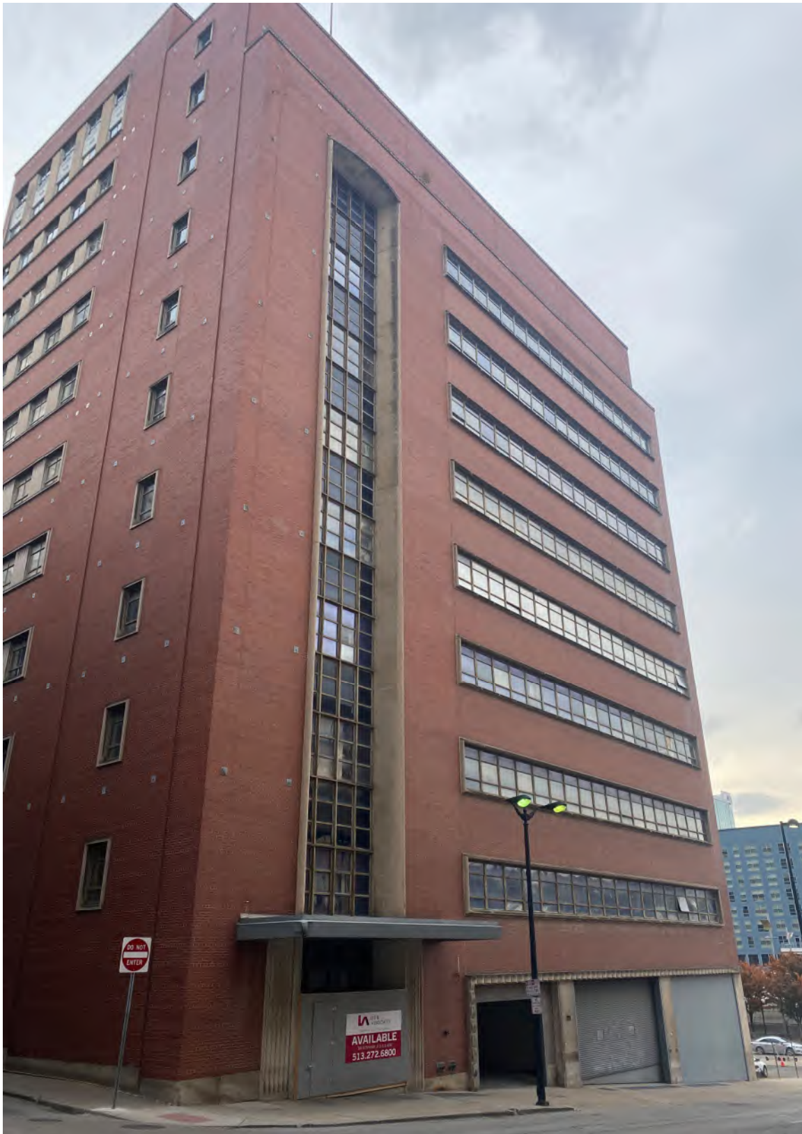
3. Exterior, West Elevation, perspective view looking southeast.
