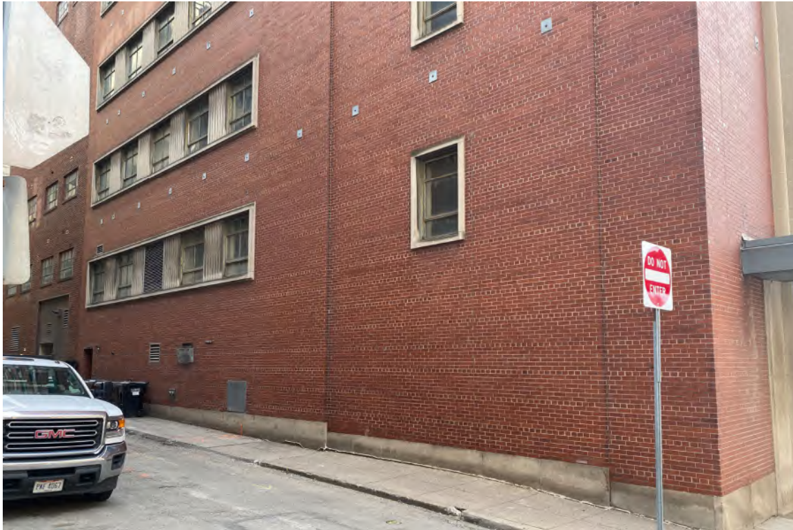
8. Exterior, North Elevation, perspective view looking southeast.
