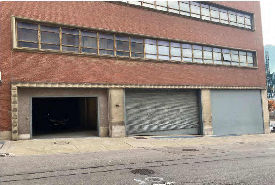
5. Exterior, West Elevation, view looking east.
