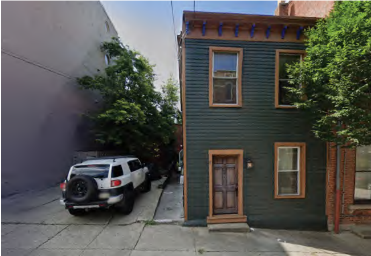
Figure 7: Previous Front facade of 341 Milton St. 2022 Google Street Views
