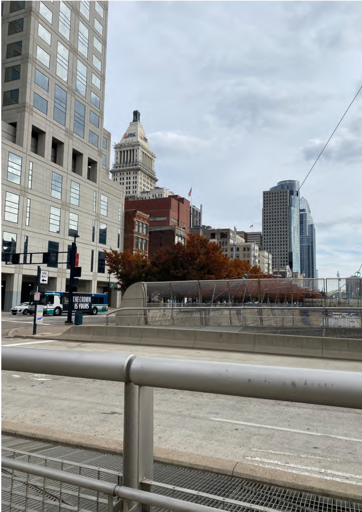
10. Exterior, West and South Elevations, perspective view looking northeast across 3rd Street.
