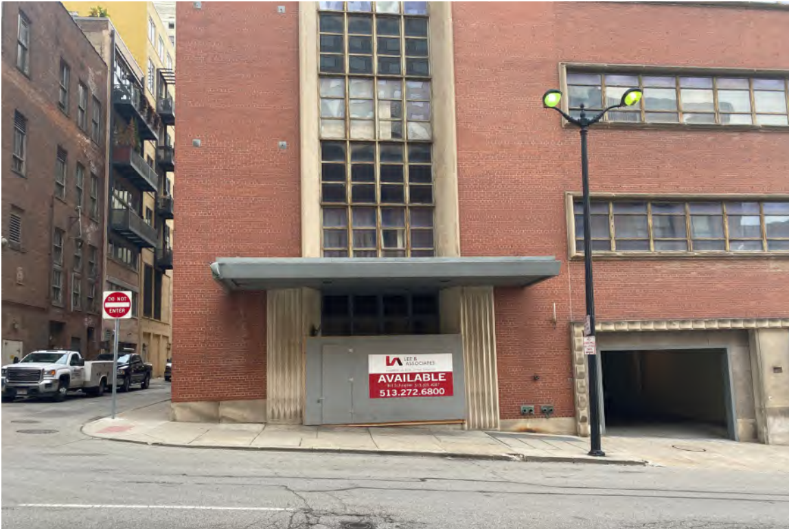
4. Exterior, West Elevation, view looking east.
