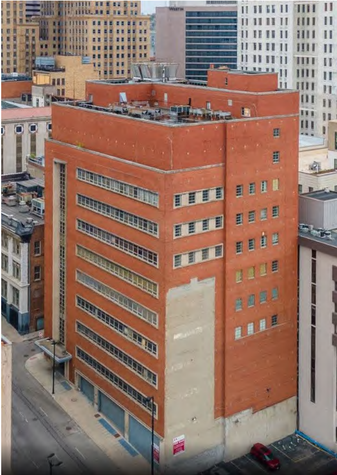
1. Exterior, West and South Elevations, perspective view looking northeast.
