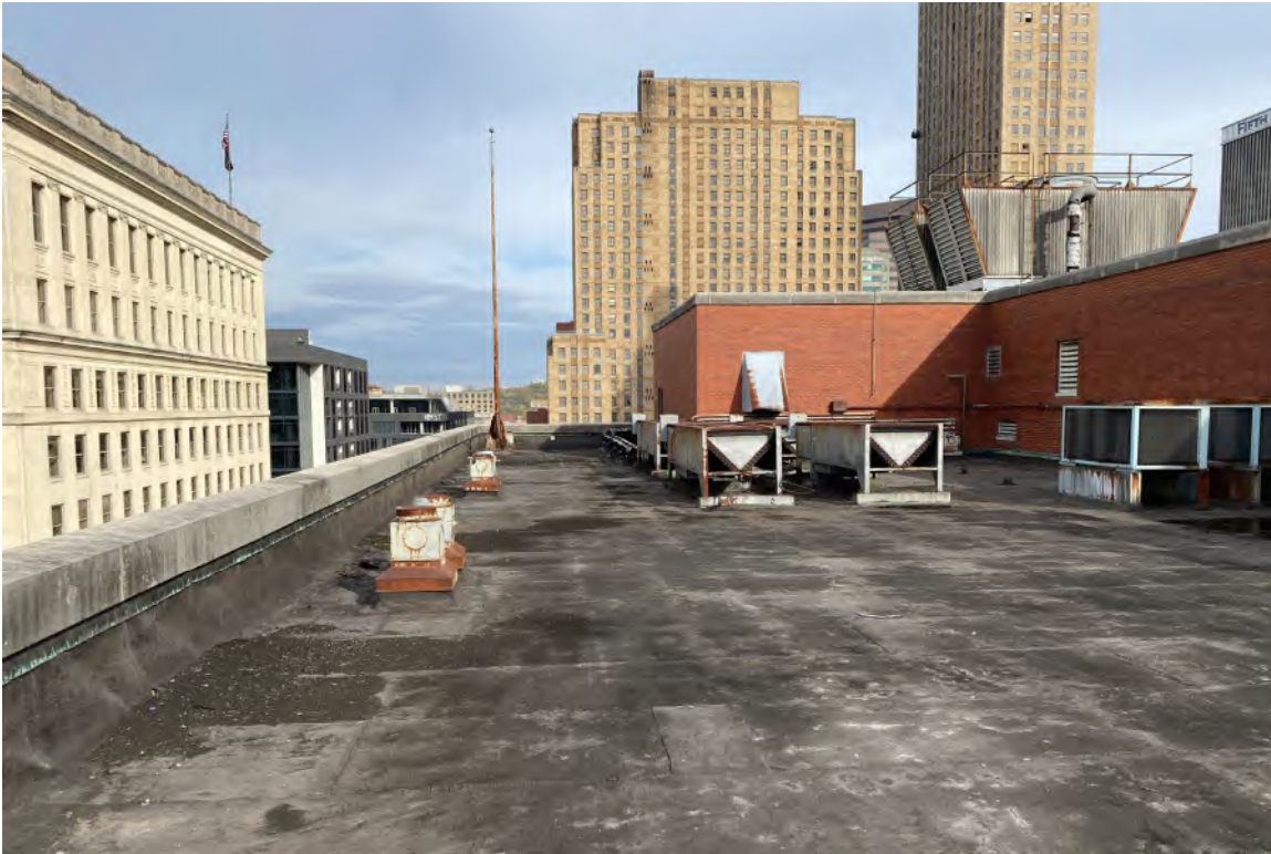
15. Exterior, Roof, view looking northeast.
