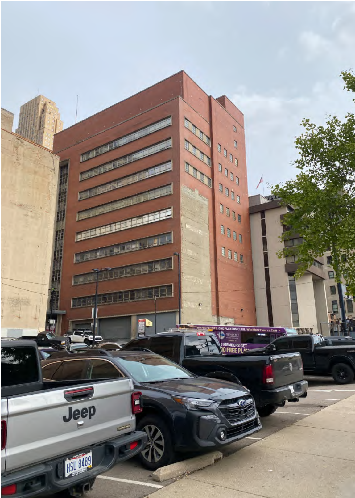
6. Exterior, West and South Elevations, view looking northeast.
