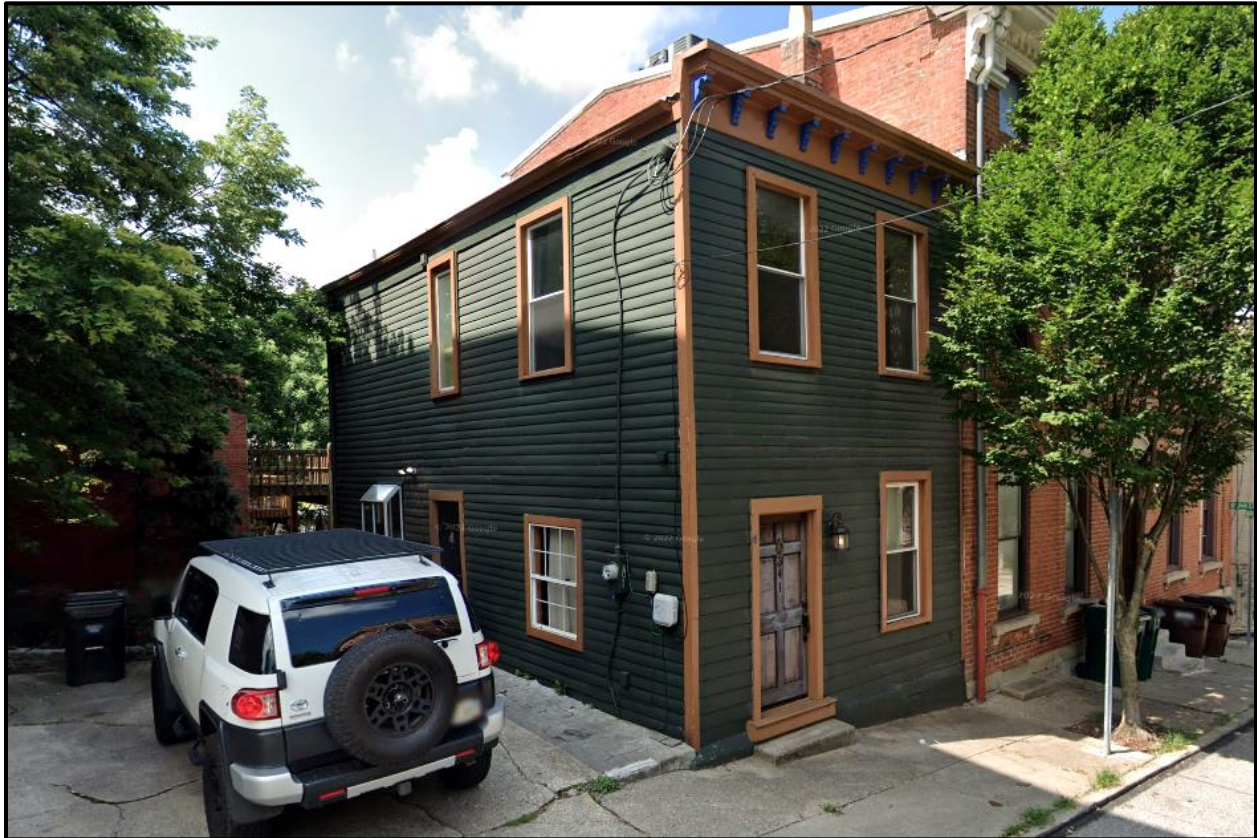
Figure 2. Image of subject property from July 2022 prior to alterations. Image from Google.
