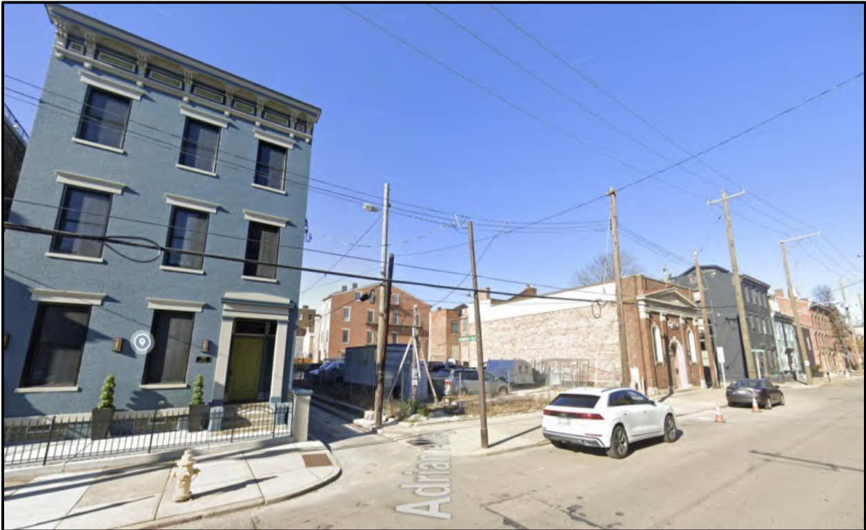
Figure 2: Street view of 1413-1415 Elm Street. Image from Google Street views.
