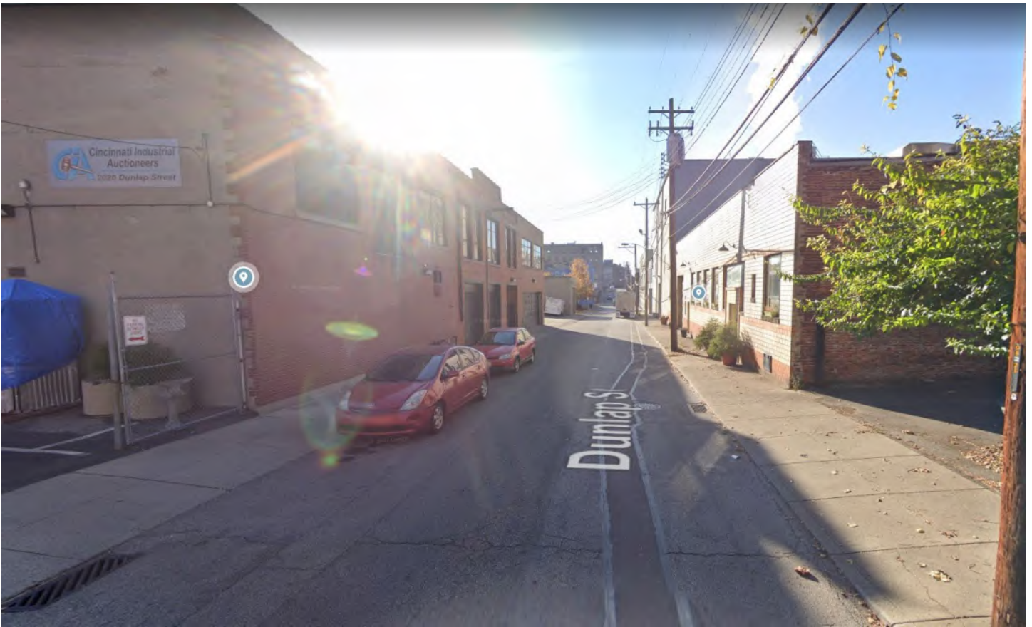
Dunlap Street north of the subject property, facing south toward the subject property: F.L. Emmert Company’s building at 2077 Dunlap on the right and Cincinnati Industrial Auctioneers, Inc.’s building at 2020 Dunlap on the left.
