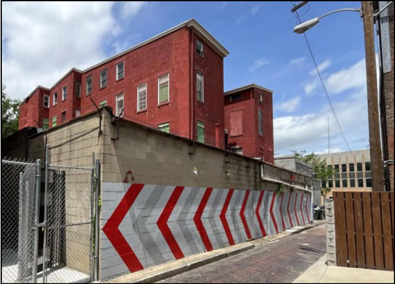
Figure 3. Image of rear of 1530-1534 Race Street. Image from applicant.
