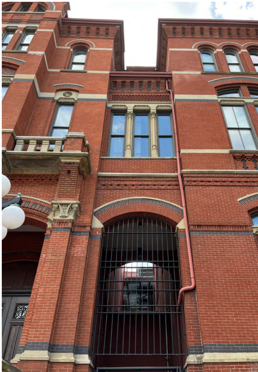
CORBELED BRICK PRECEDENT Cincinnati Music Hall 1241 Elm Street
