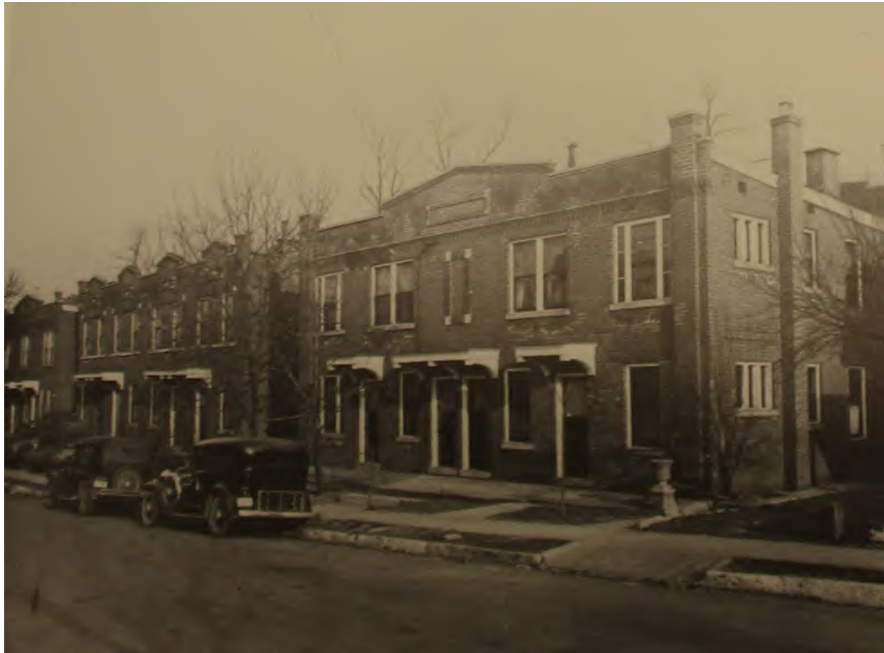
Figure 10. (R-L) 3066-3068 Kerper Avenue, 3070-3076 Kerper Avenue, and 3078-3083 Kerper Avenue in the 1920s before the front parapet reconstruction.
