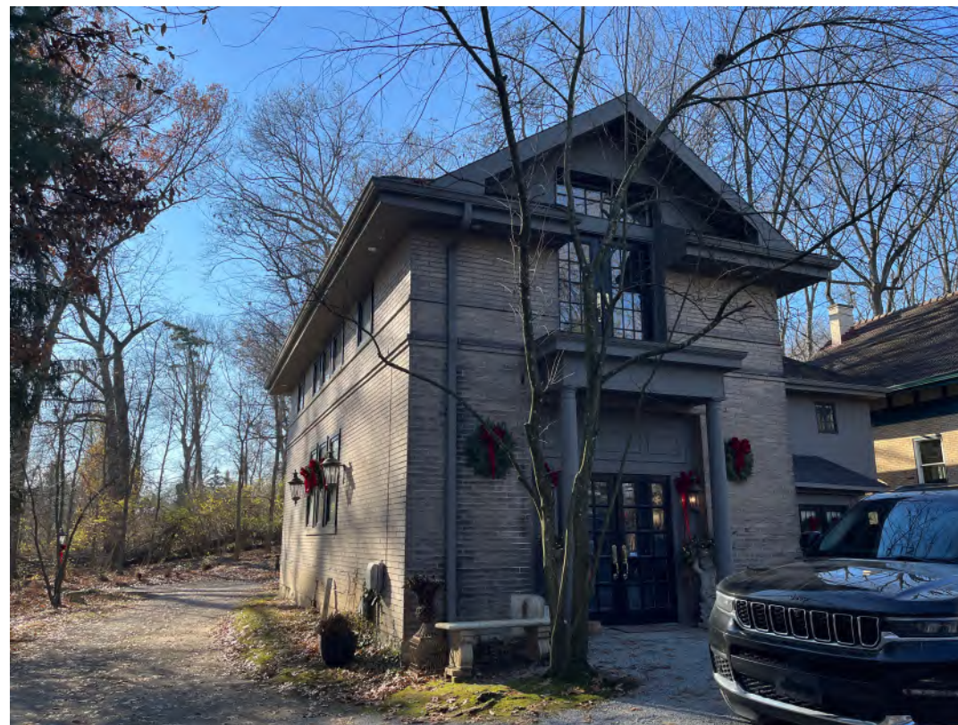
2. Existing Side View - where Addition will connect
