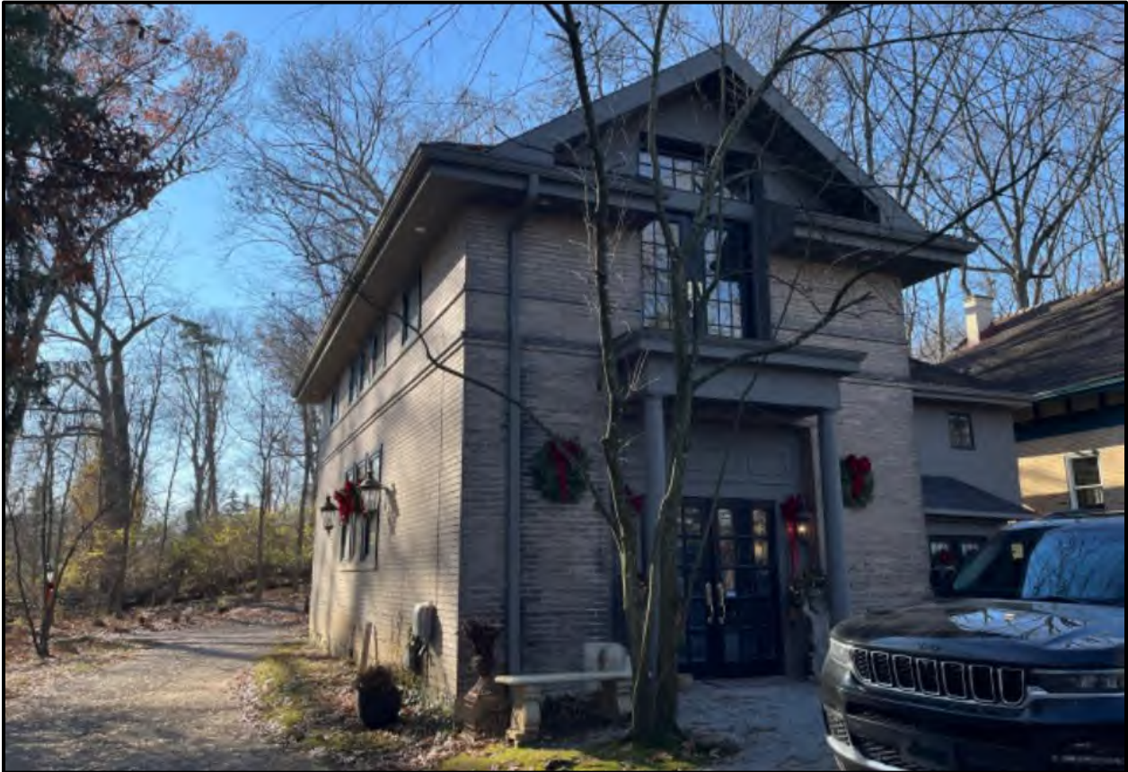
Figure 3: Image of north elevation at location of proposed addition, facing south. Image from applicant.
