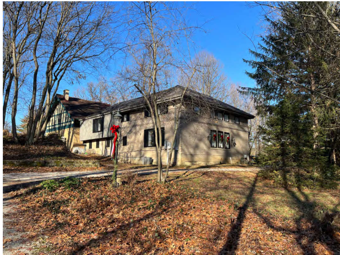
1. View of Existing Carriage House from Driveway
