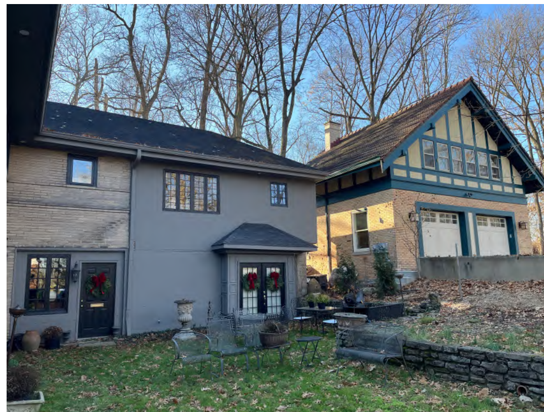
4. Existing Rear View - (neighboring property Garage on Right)
