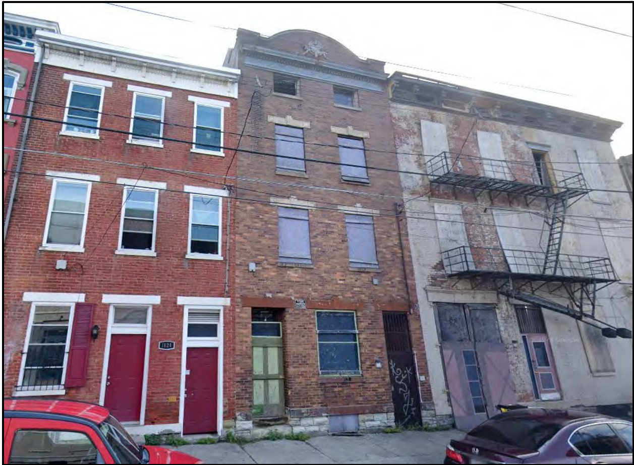
Figure 2: 1618 Walnut Street at center, ca. July 2022, facing east. Image from Google.
