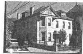
Rectory, view NW
