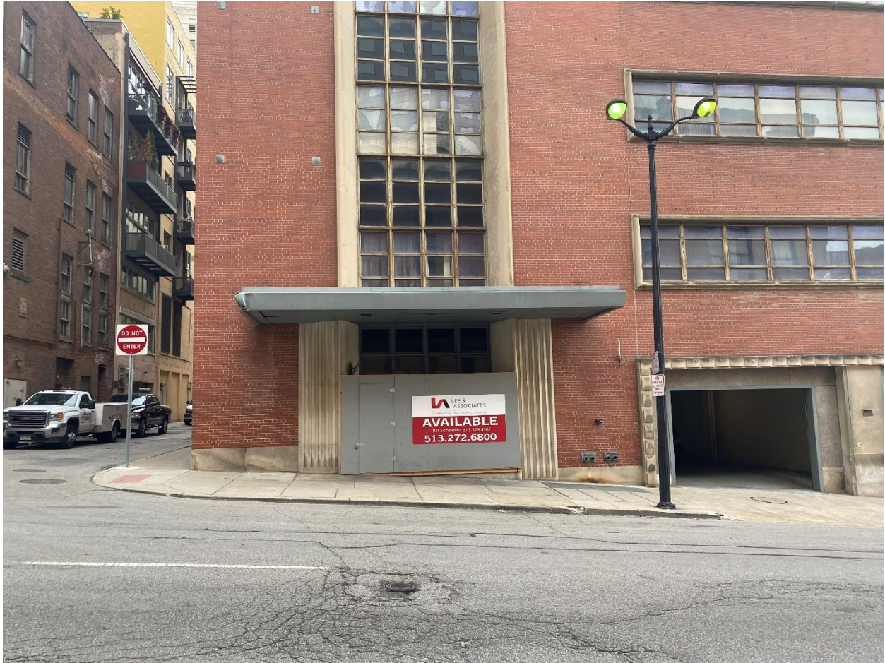
Photograph 4: West elevation looking east at entrance.
