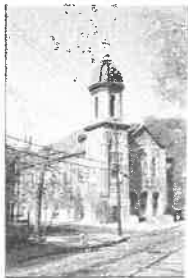
Church, view SW
