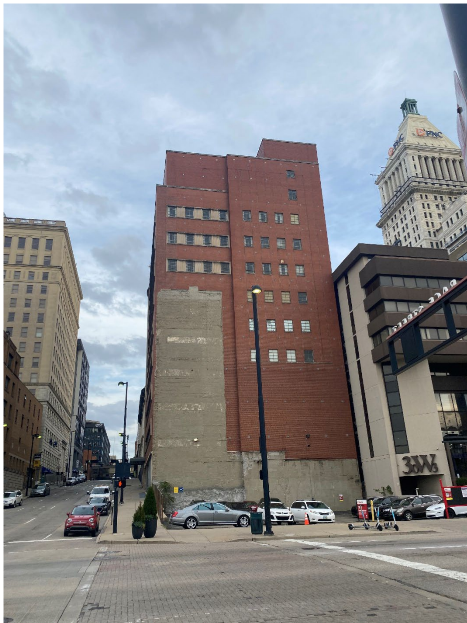
Photograph 8: South elevation looking north.
