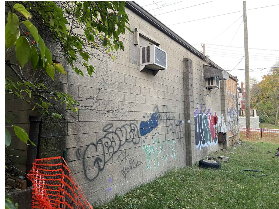
5 EXIST. ELEVATION D200 PHOTO SOUTH WEST CORNER
