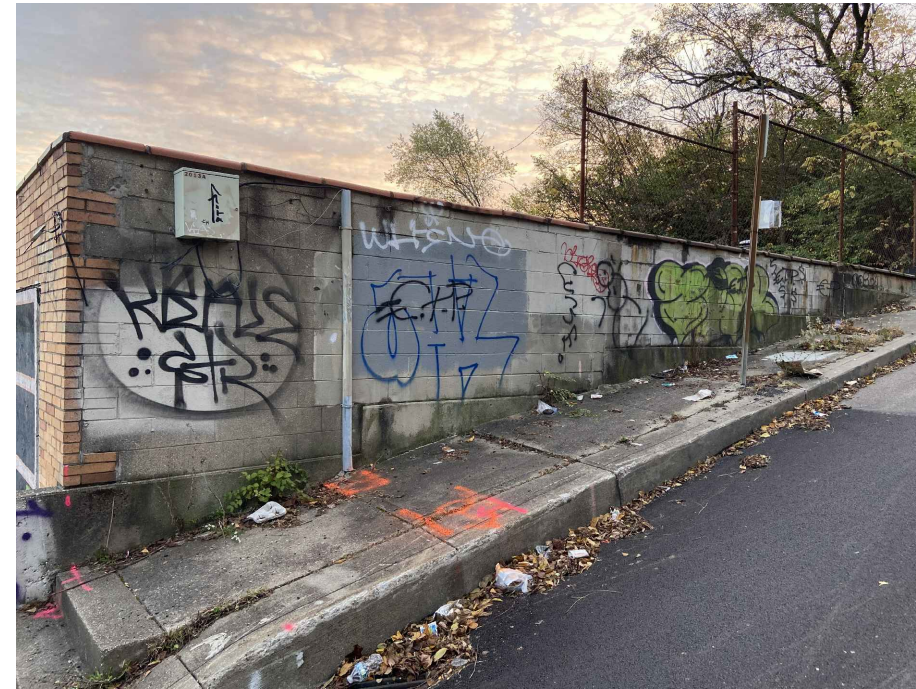
2 EXIST. ELEVATION D200 PHOTO NORTH EAST CORNER
