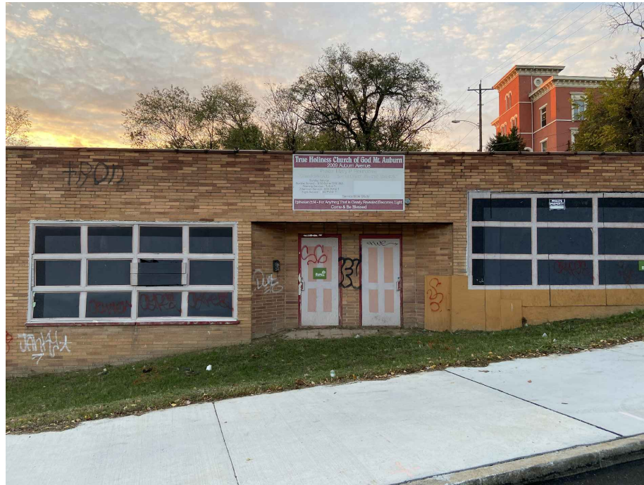
1 EXIST. ELEVATION D200 PHOTO EAST SIDE (FRONT)
