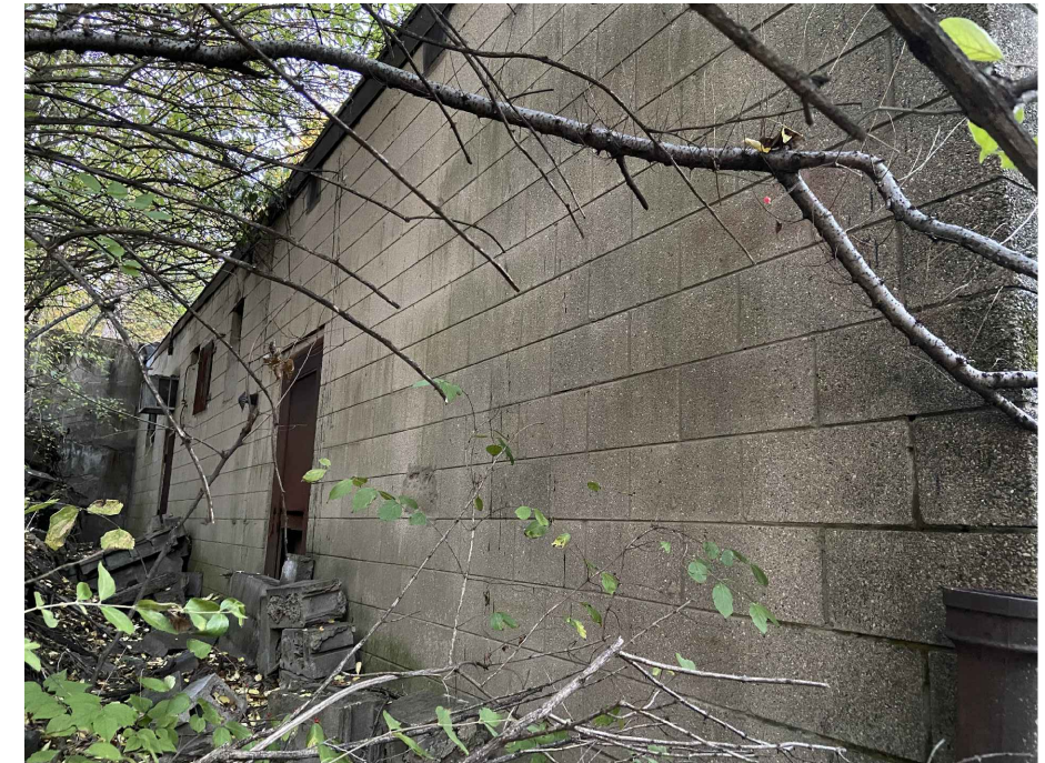
6 EXIST. ELEVATION D200 PHOTO WEST SIDE (REAR)
