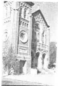
Church detail, view SW
