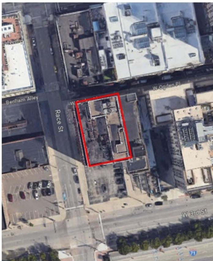
Figure 1: The H. & S. Pogue Service Building, with boundary shown in red.
