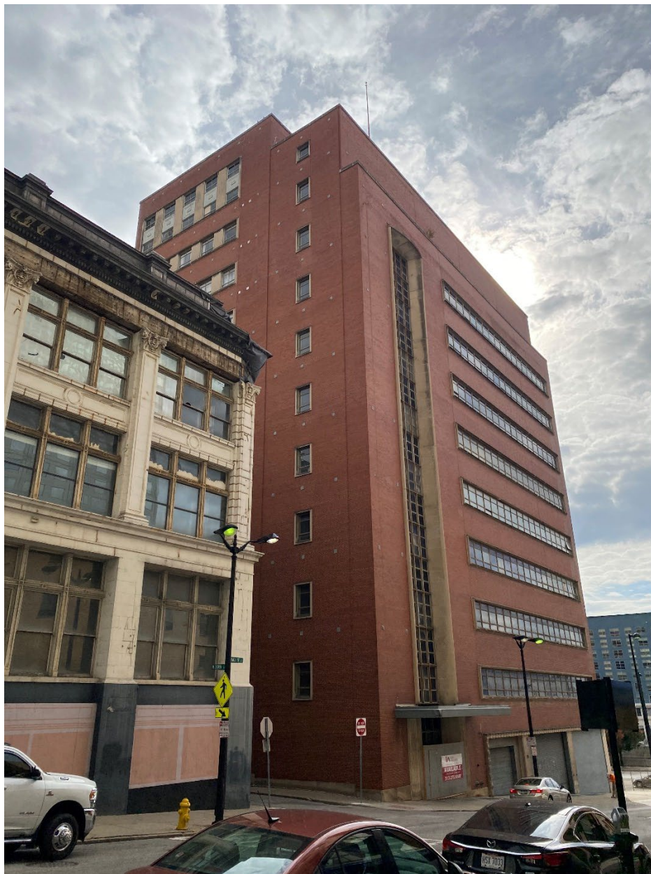
Photograph 1: West and north elevations looking southeast.
