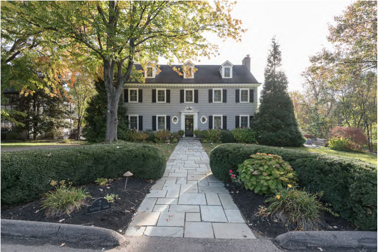
7 Annwood Ln, Front (West) Side
