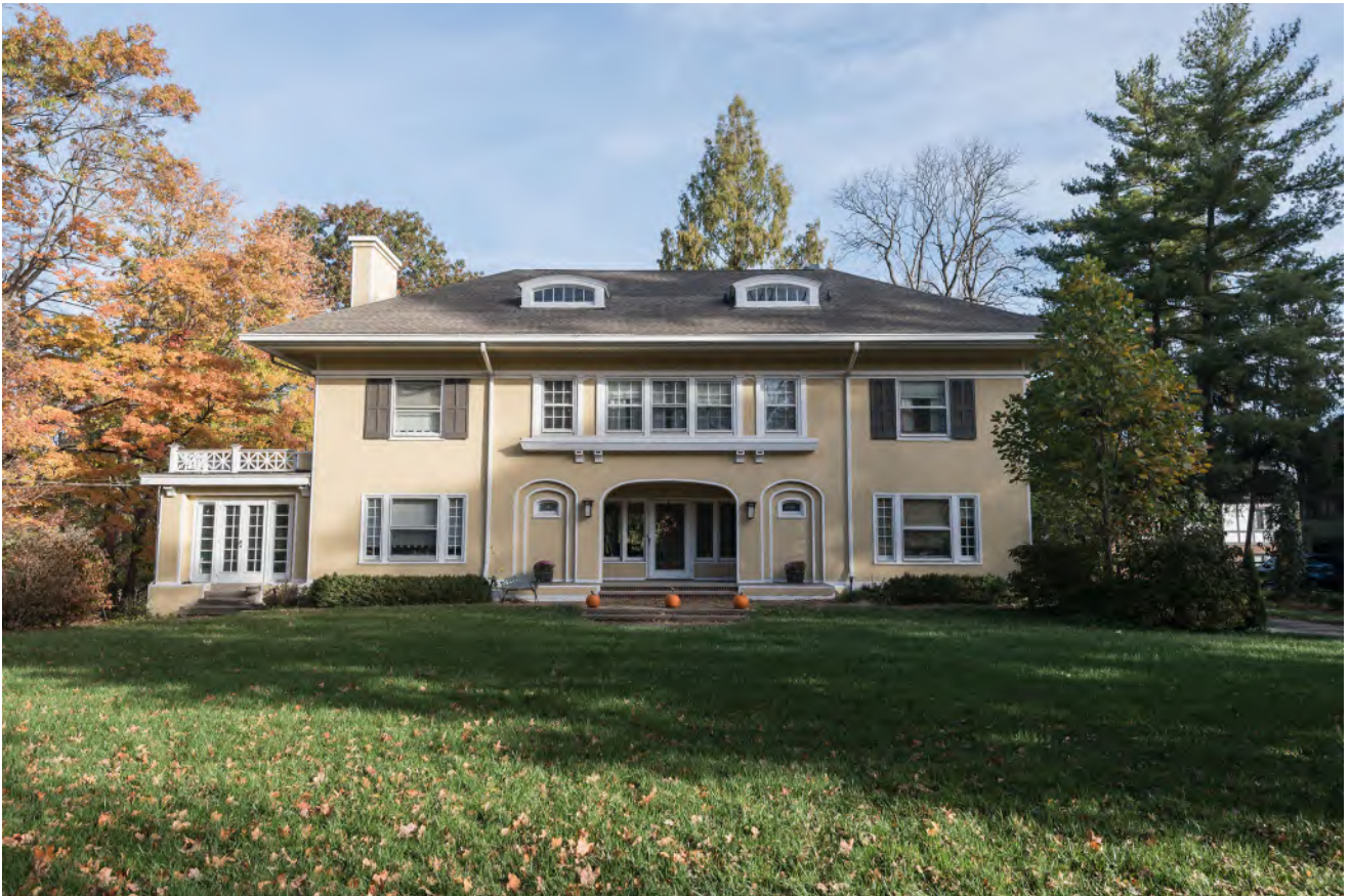
1 Annwood Ln, Front (South) Side
