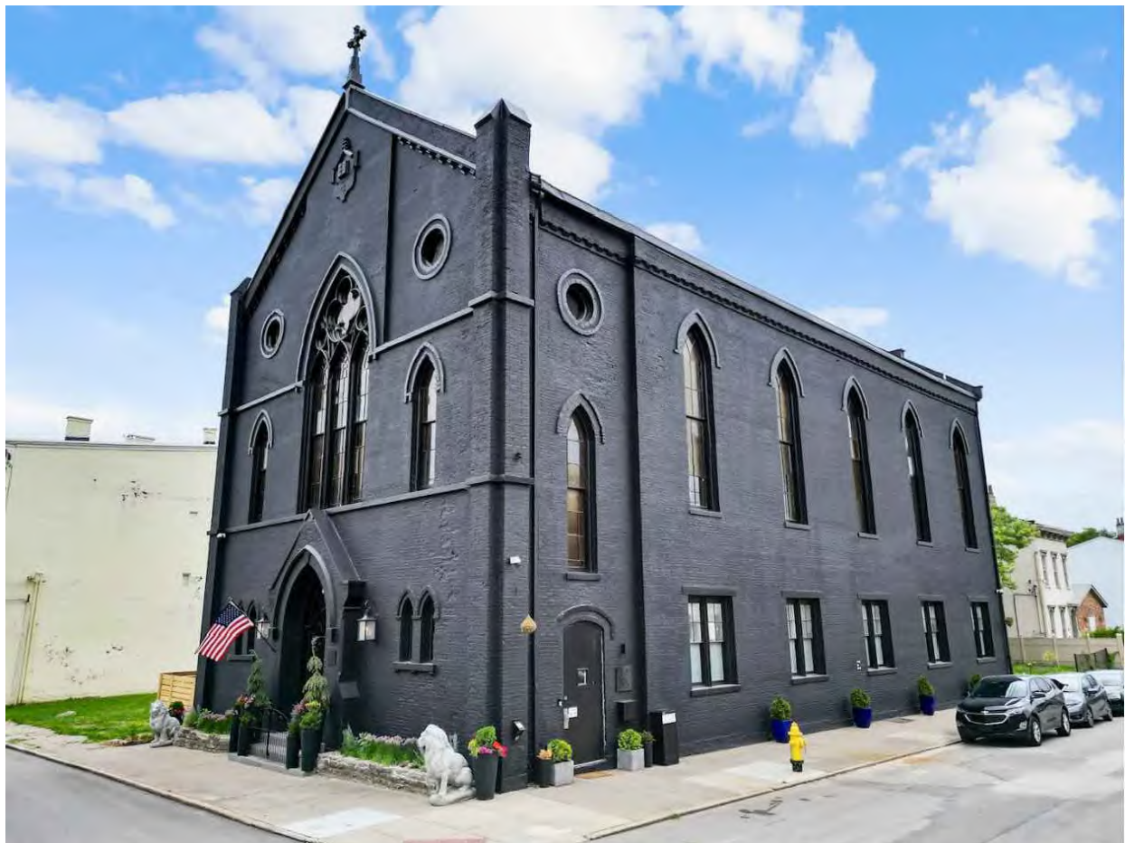
4. LOOKING SOUTH WEST FROM INTERSECTION OF BAYMILLER ST AND YORK ST
