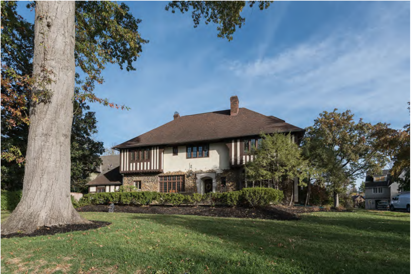
6 Annwood Ln, Front (South) Side
