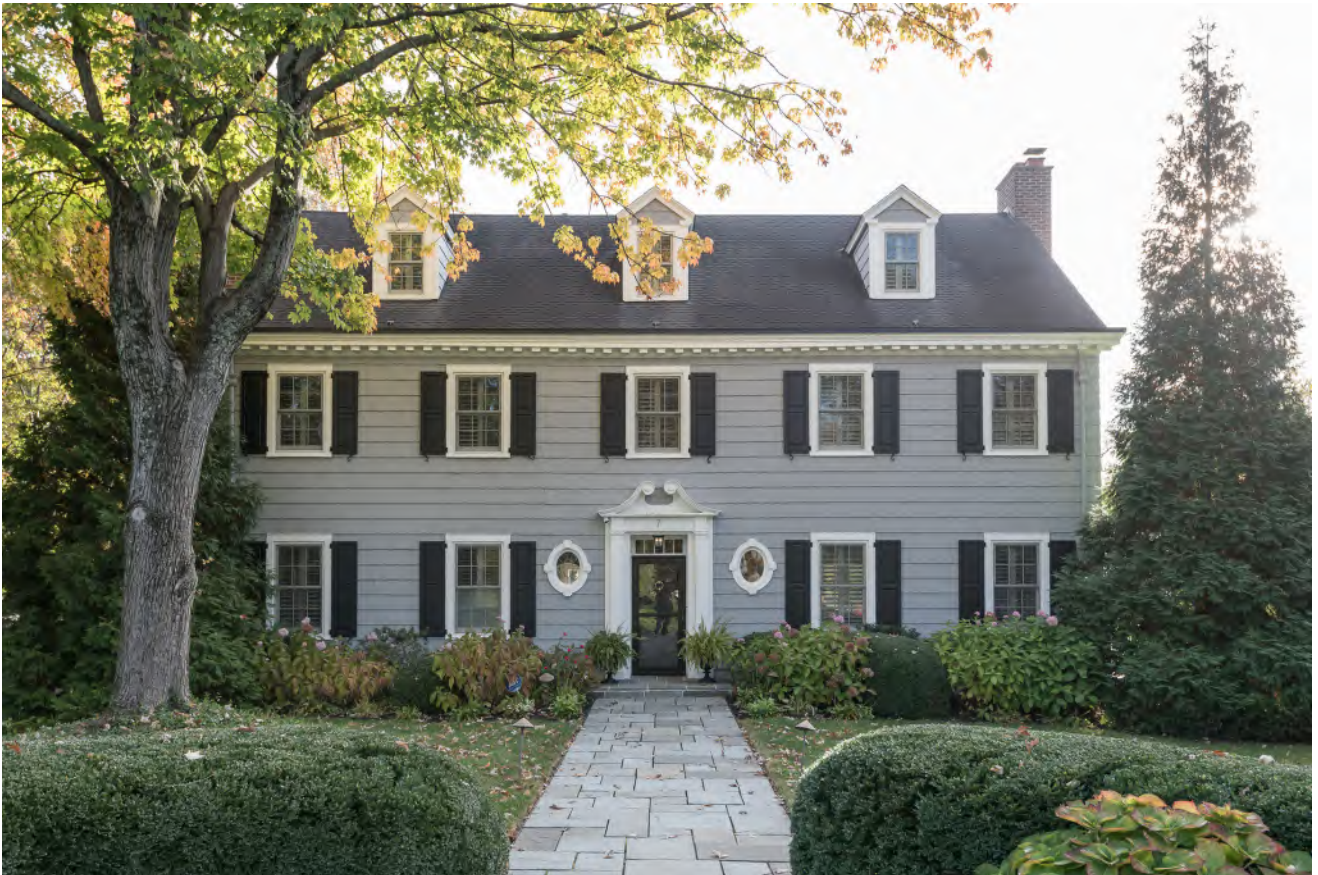
7 Annwood Ln, Front (West) Side Detail
