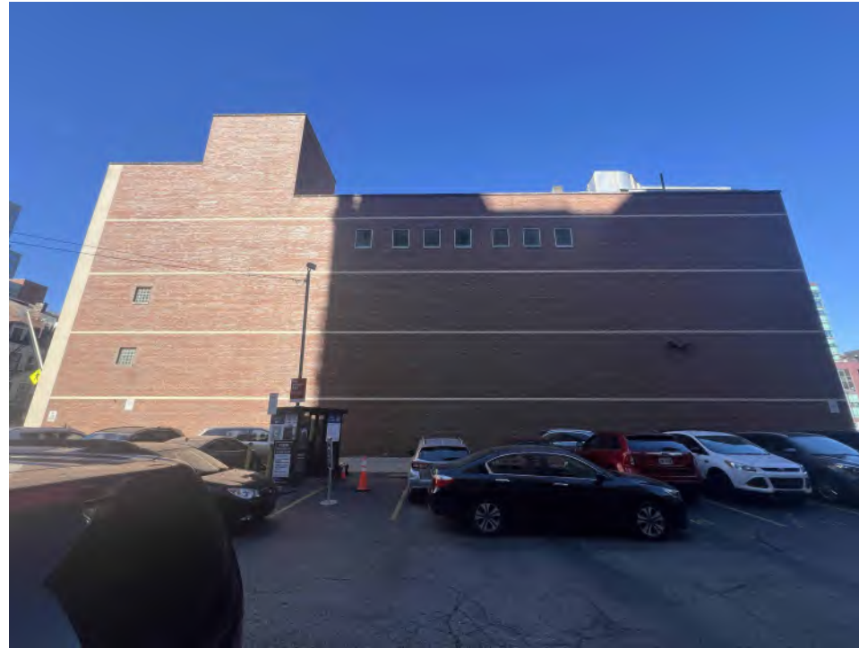
630 Main St (Looking north) Existing South Facade
