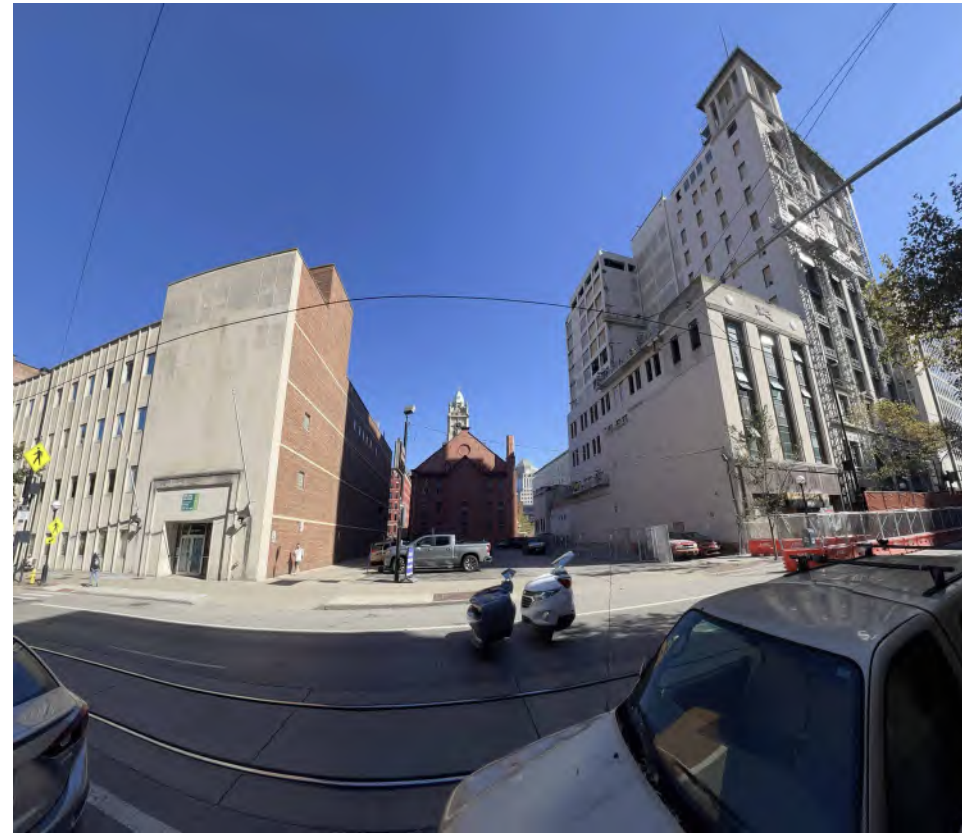
630 Main St + 602 Main St West Facade(s) (Looking east) West facade and South Wall of 630 Main St + West Facade and North Wall of 602 Main St
