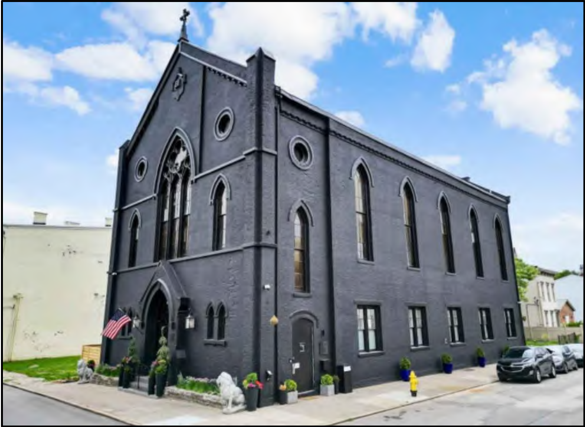
Figure 2. View of 1835 Baymiller Street. Image from applicant.
