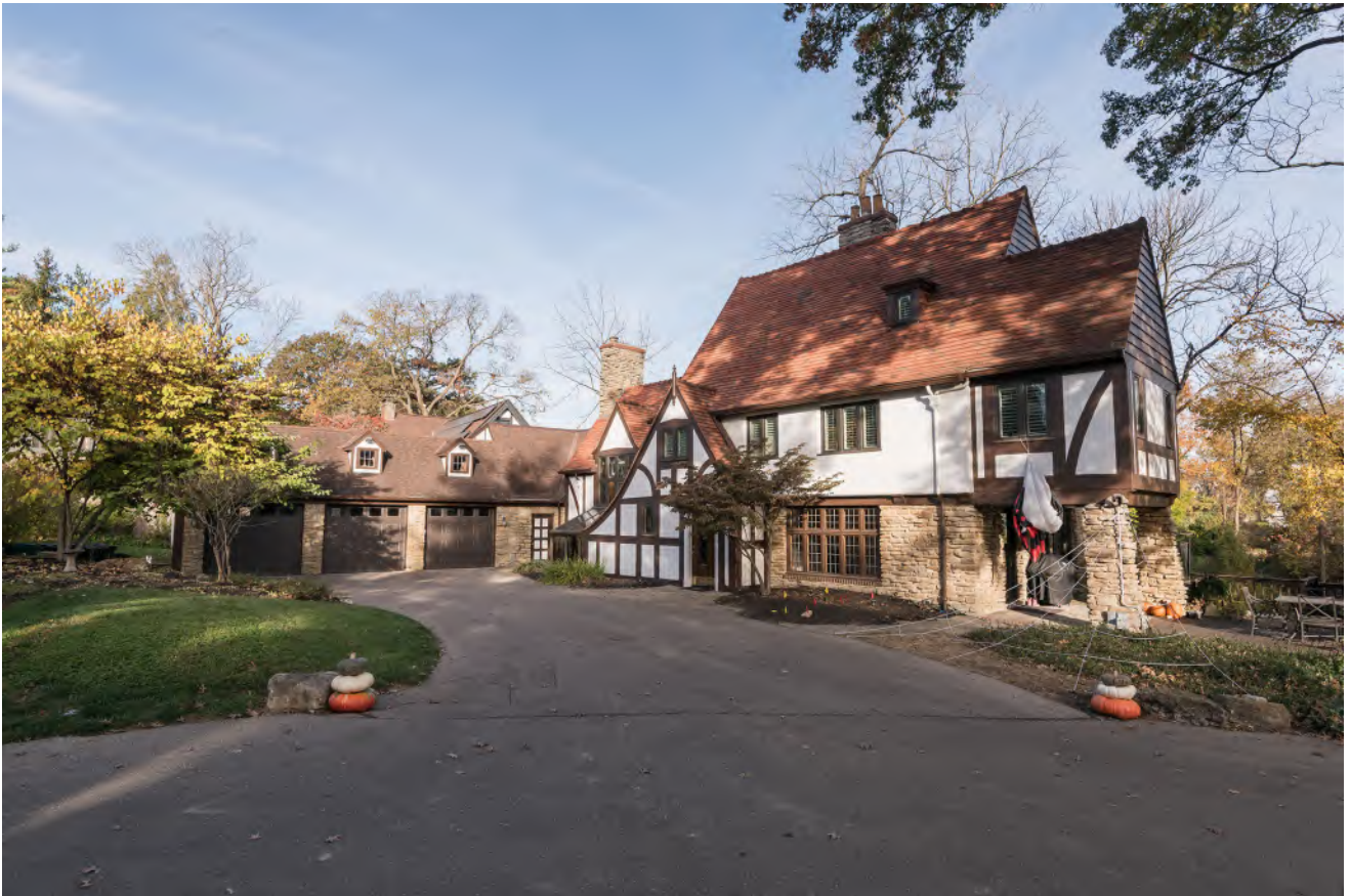
8 Annwood Ln, Front (Southeast) Side
