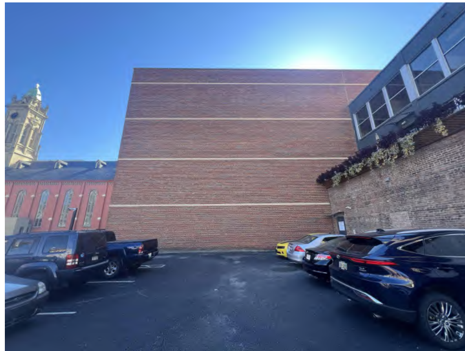
630 Main St (Looking south) Existing North Wall + Rear of 646 Main St
