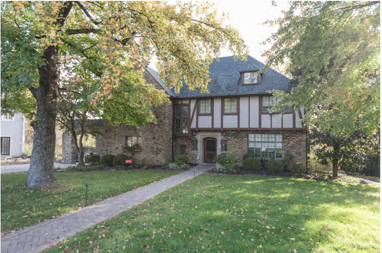
9 Annwood Ln, Front (West) Side
