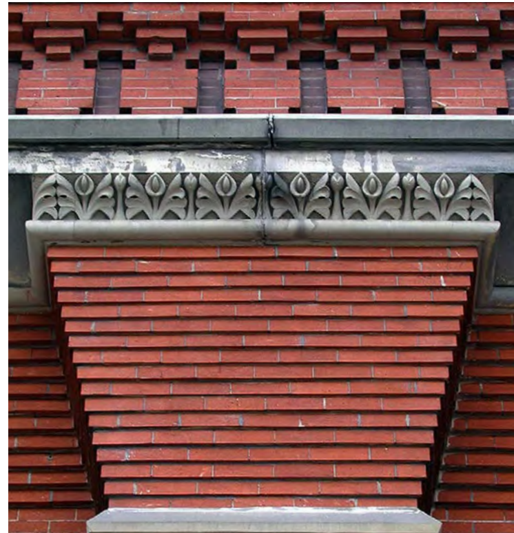
CORBEL DETAIL AT MUSIC HALL
