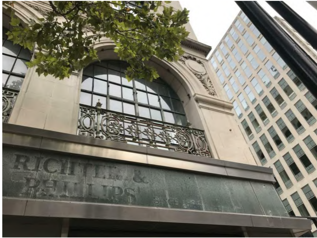
EXTERIOR VIEW OF WINDOW
