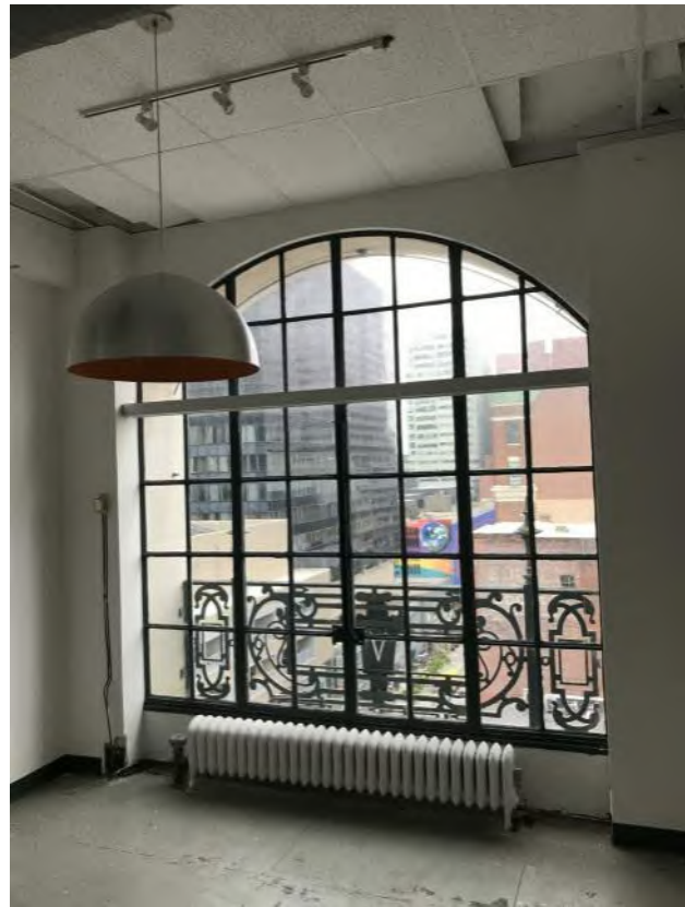
INTERIOR VIEW OF WINDOW
