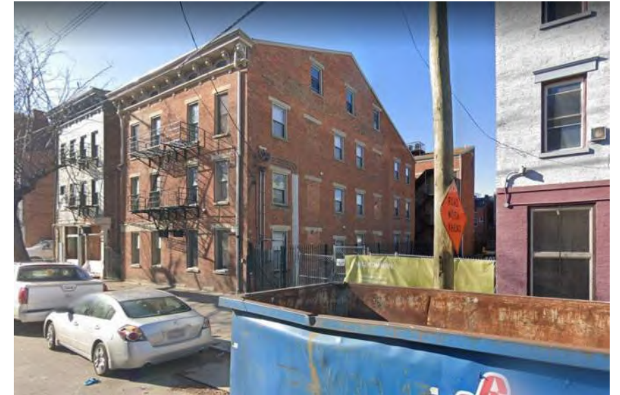
NORTH FACADE OF BUILDING TO THE SOUTH
