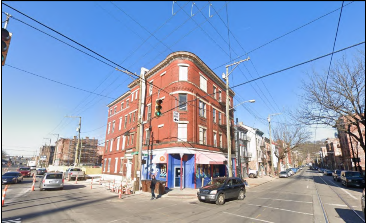
Figure 2. View of 1601 Race Street ca. November 2020. Image from Google.
