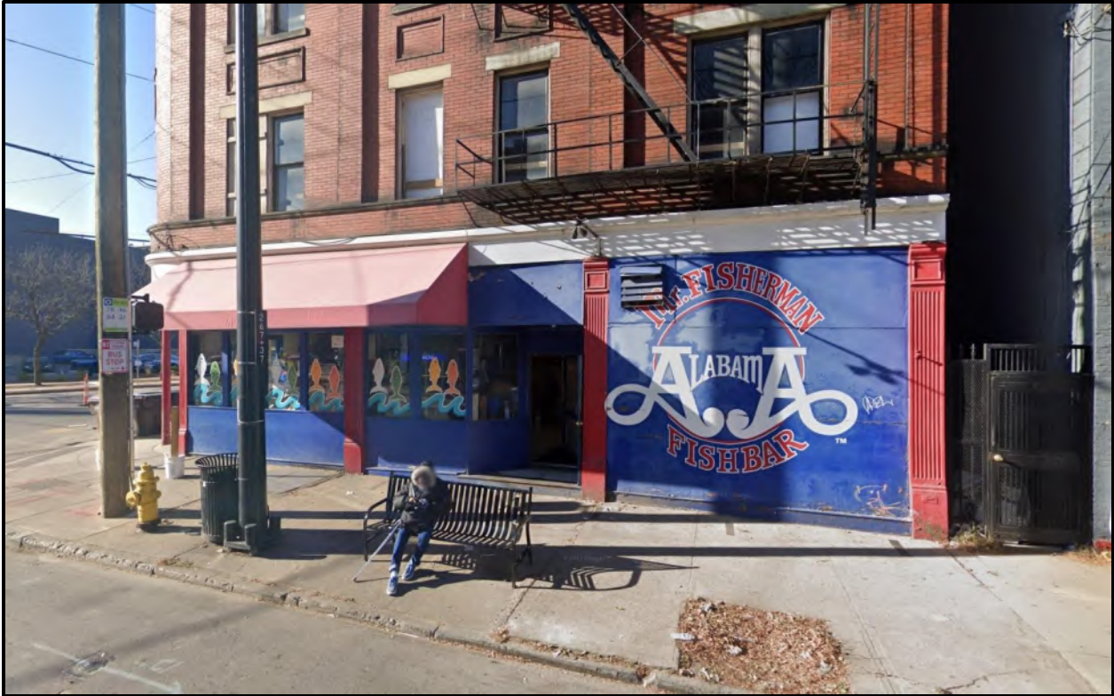
Figure 3. Detail of existing East Elevation. Image from Google.
