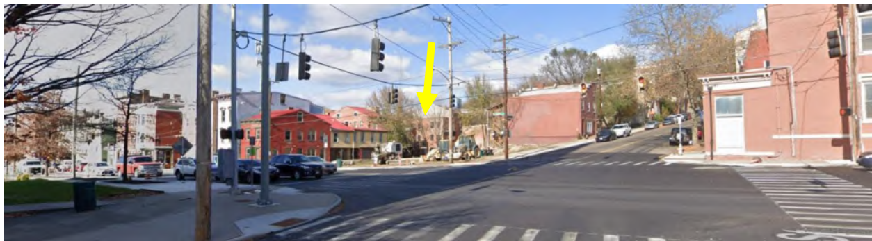
Figure 2: Street view of 228 E Liberty Street. The site is identified by the yellow arrow. Image provided by Google Street views.
