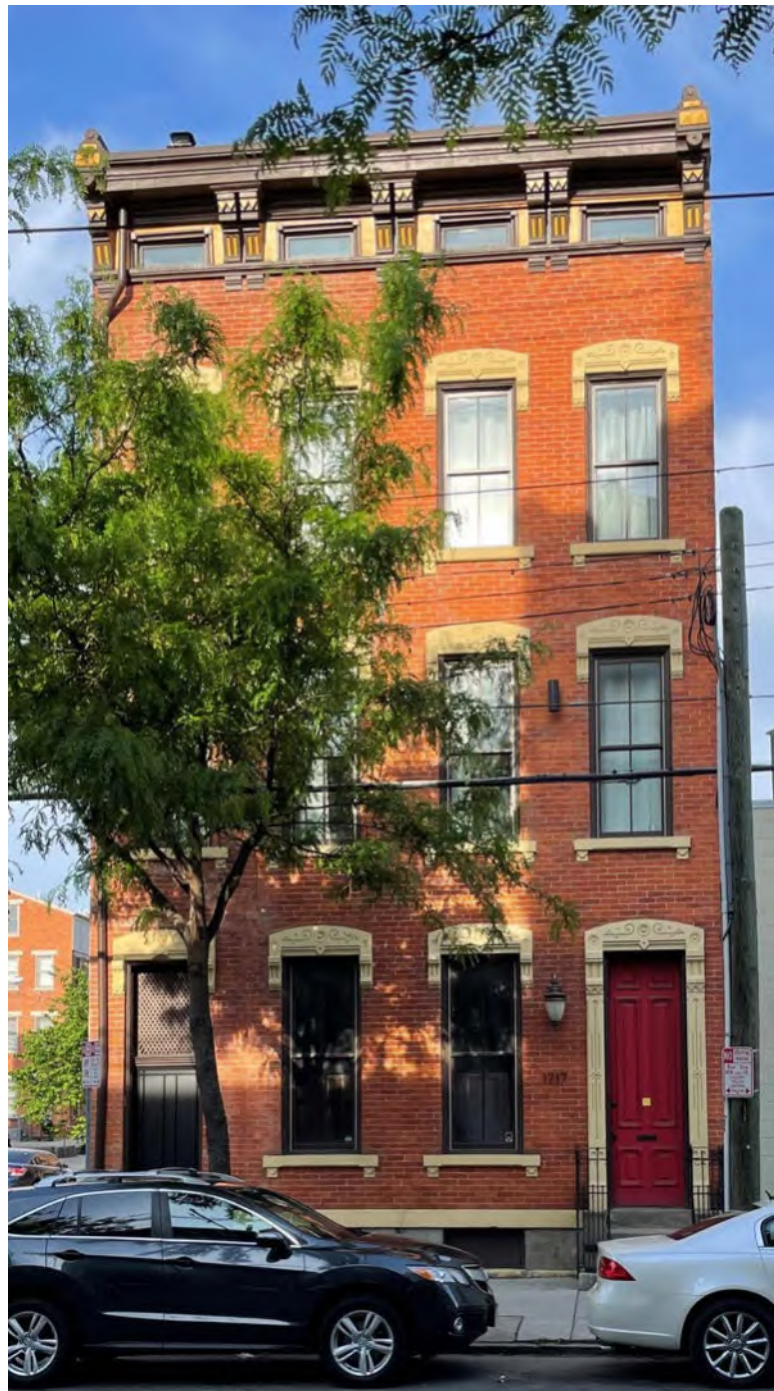
TYPICAL BUILDING IN OTR
