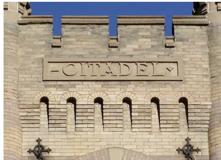
CORBEL DETAIL ON SALVATION ARMY BUILDING
