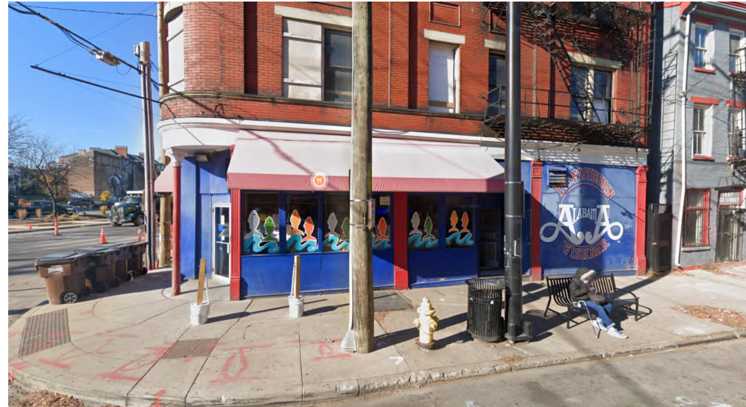
Existing East Facade (Primary)
