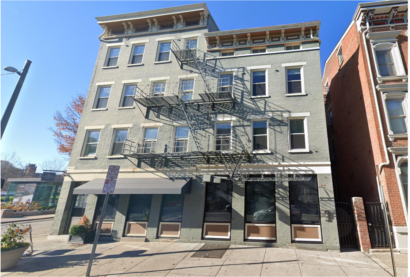
1401 Race St. - East (Front) Elevation (Google street view)
