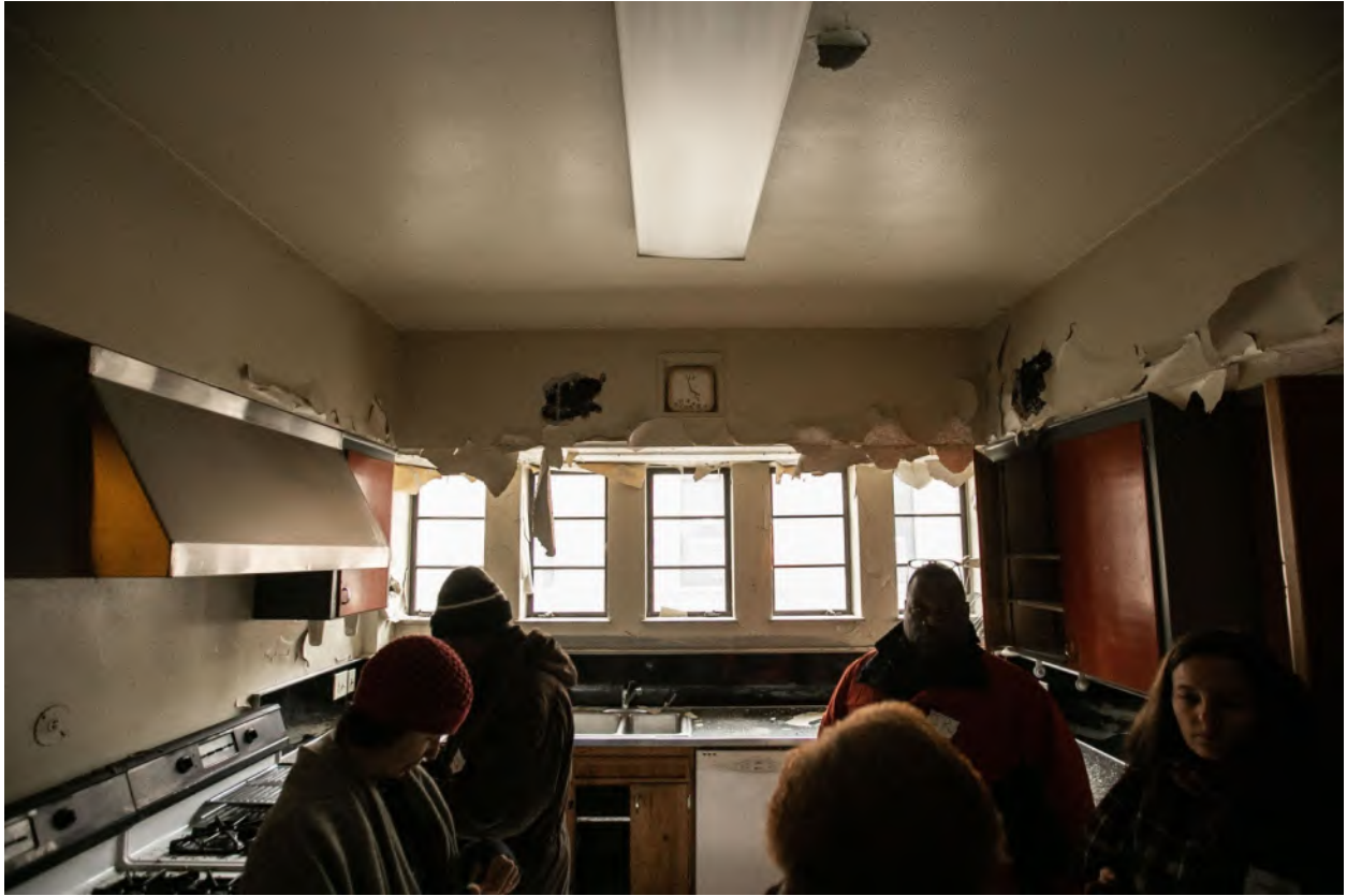
Figure 11 View of former kitchen with wood cabinets and awning windows.
