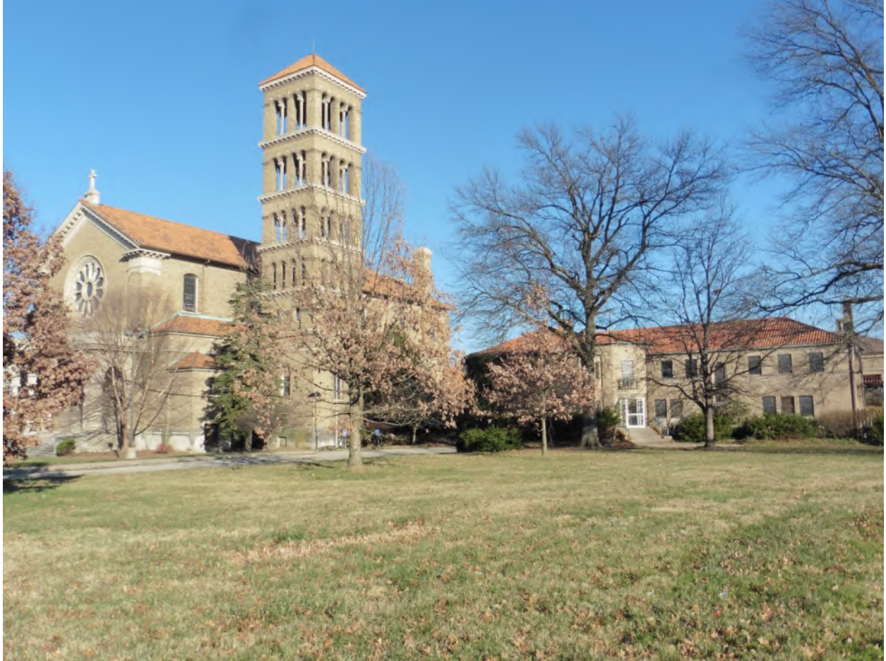
Figure 2 Overall view of St. Mark from Montgomery Road. View to the NE.
