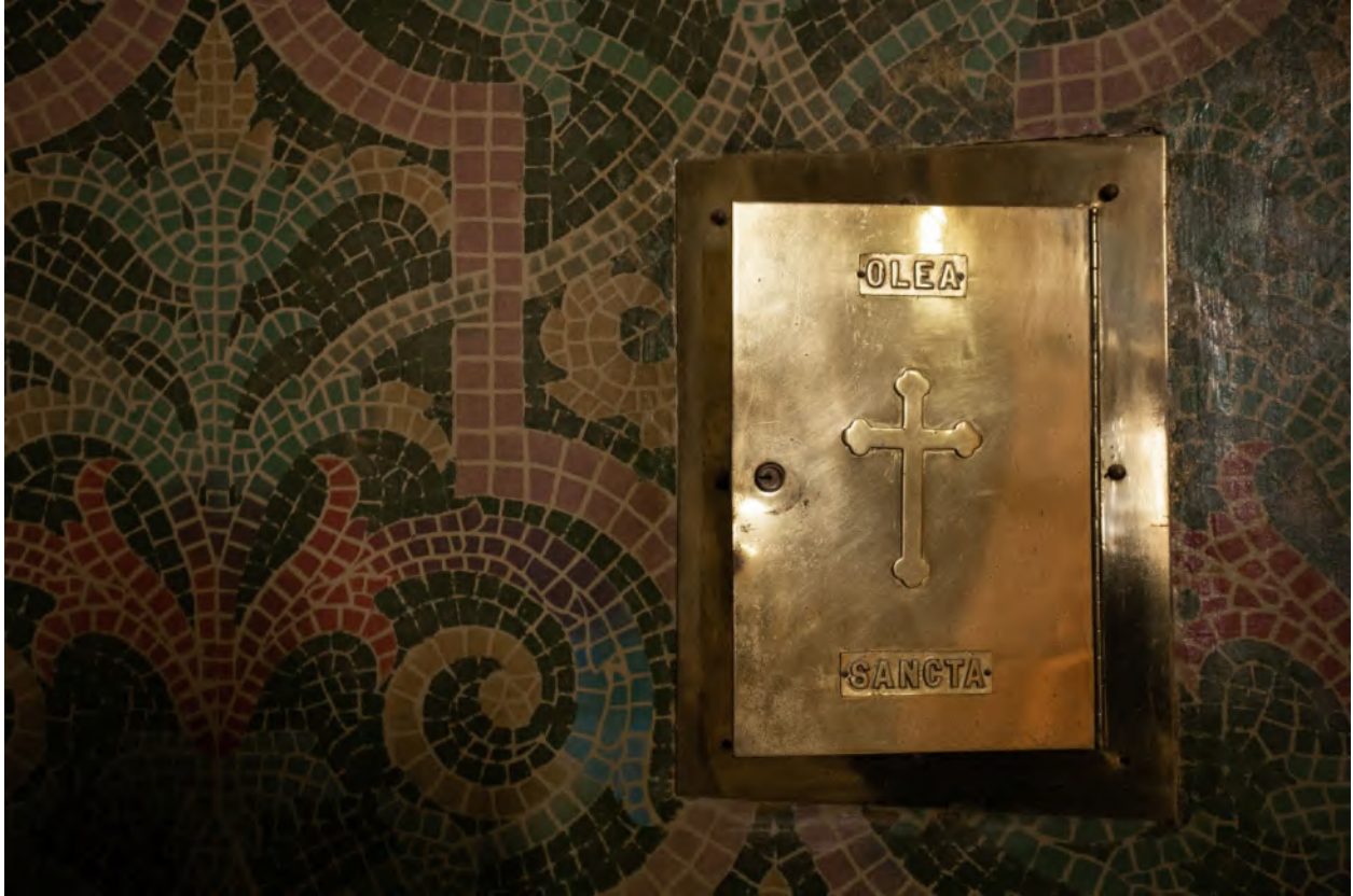
Figure 9 Detail view of mosaic wall treatment and brass cabinet for storage of holy oil.
