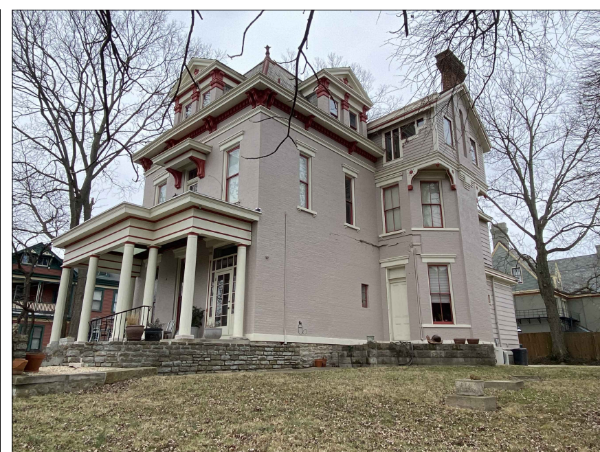
G. LOOKING NORTHEAST TOWARDS WEST/FRONT AND SOUTH/SIDE ELEVATIONS OF HOUSE
