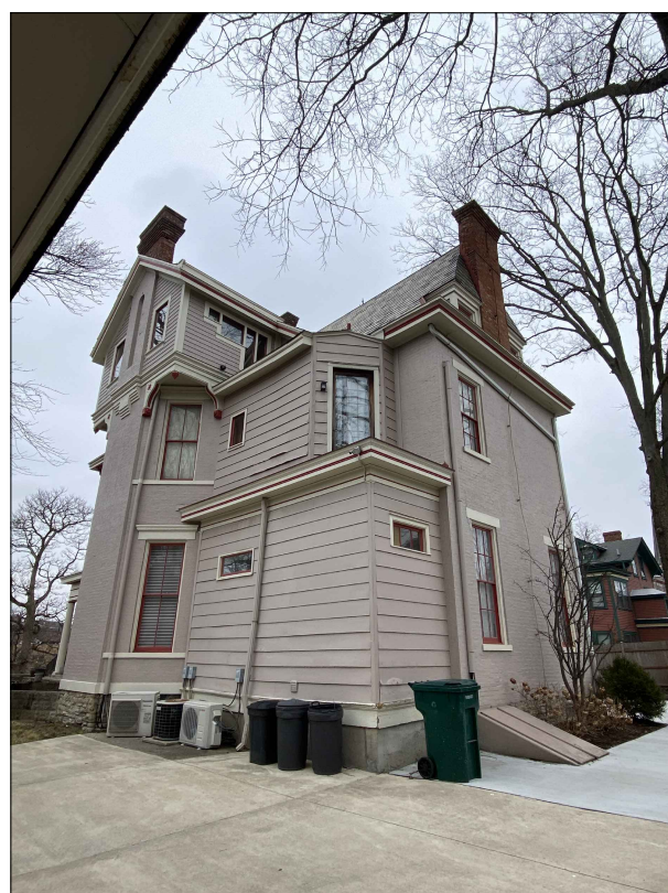
E. LOOKING NORTHWEST TOWARDS EAST/REAR ELEVATION OF HOUSE
