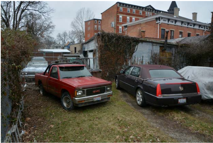
REAR/SIDE FROM PARKING LOT - LOOKING SOUTHWEST SCALE: NTS
