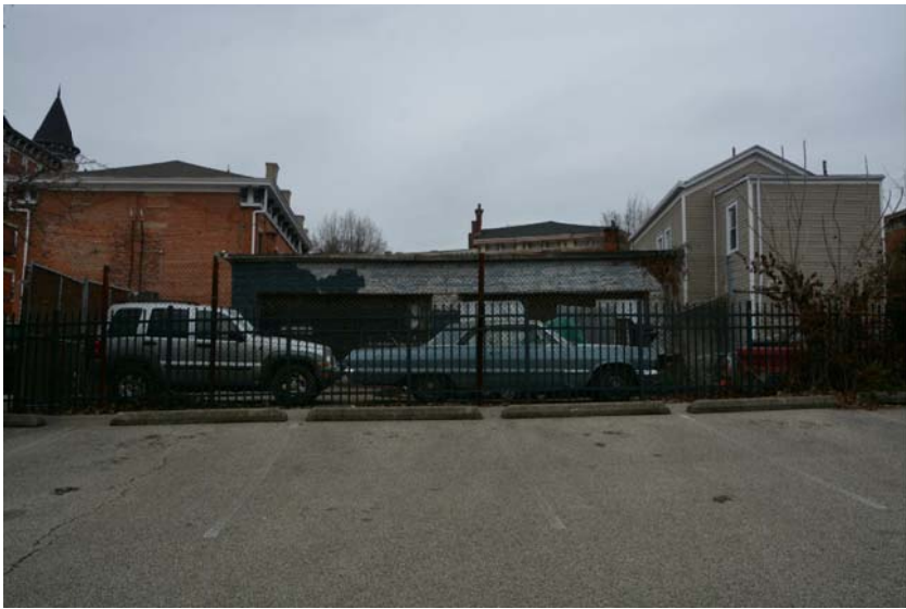
REAR FROM PARKING LOT - EAST SCALE: NTS
