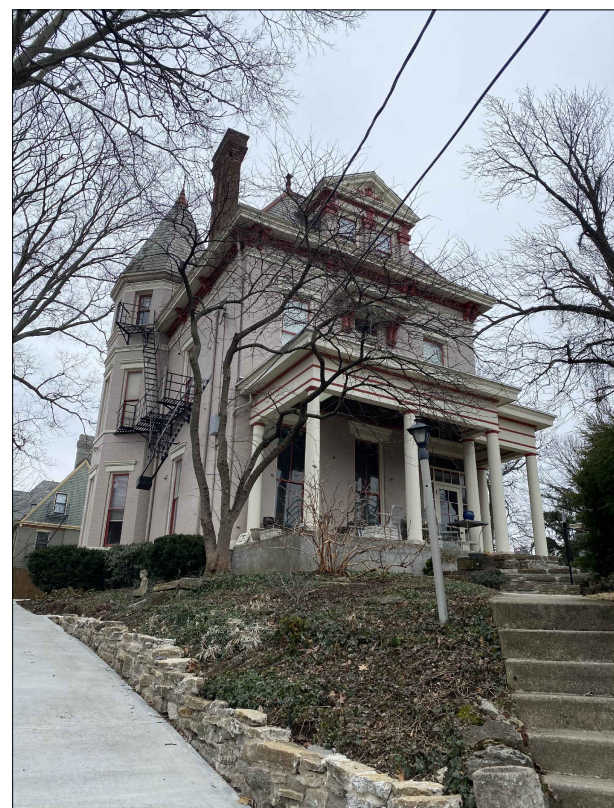
B. LOOKING SOUTHEAST TOWARDS WEST/FRONT ELEVATION OF HOUSE
