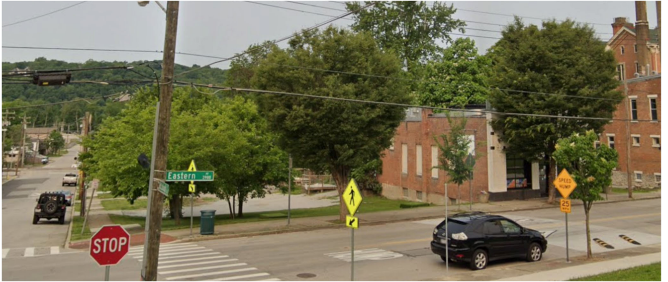
Google street view of the subject property from Eastern Ave.
