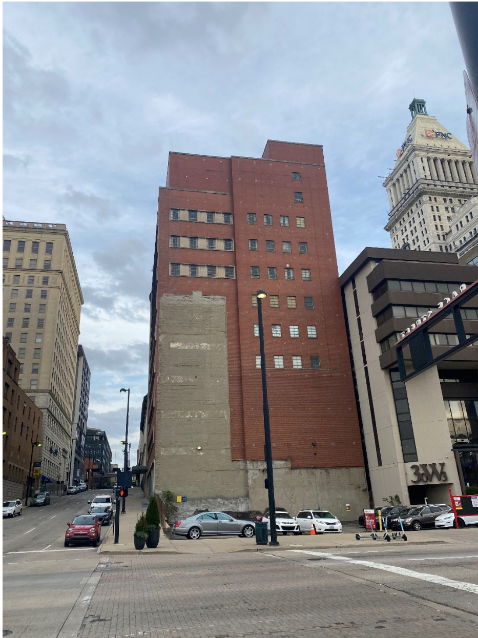
Photograph 8: South elevation looking north.
