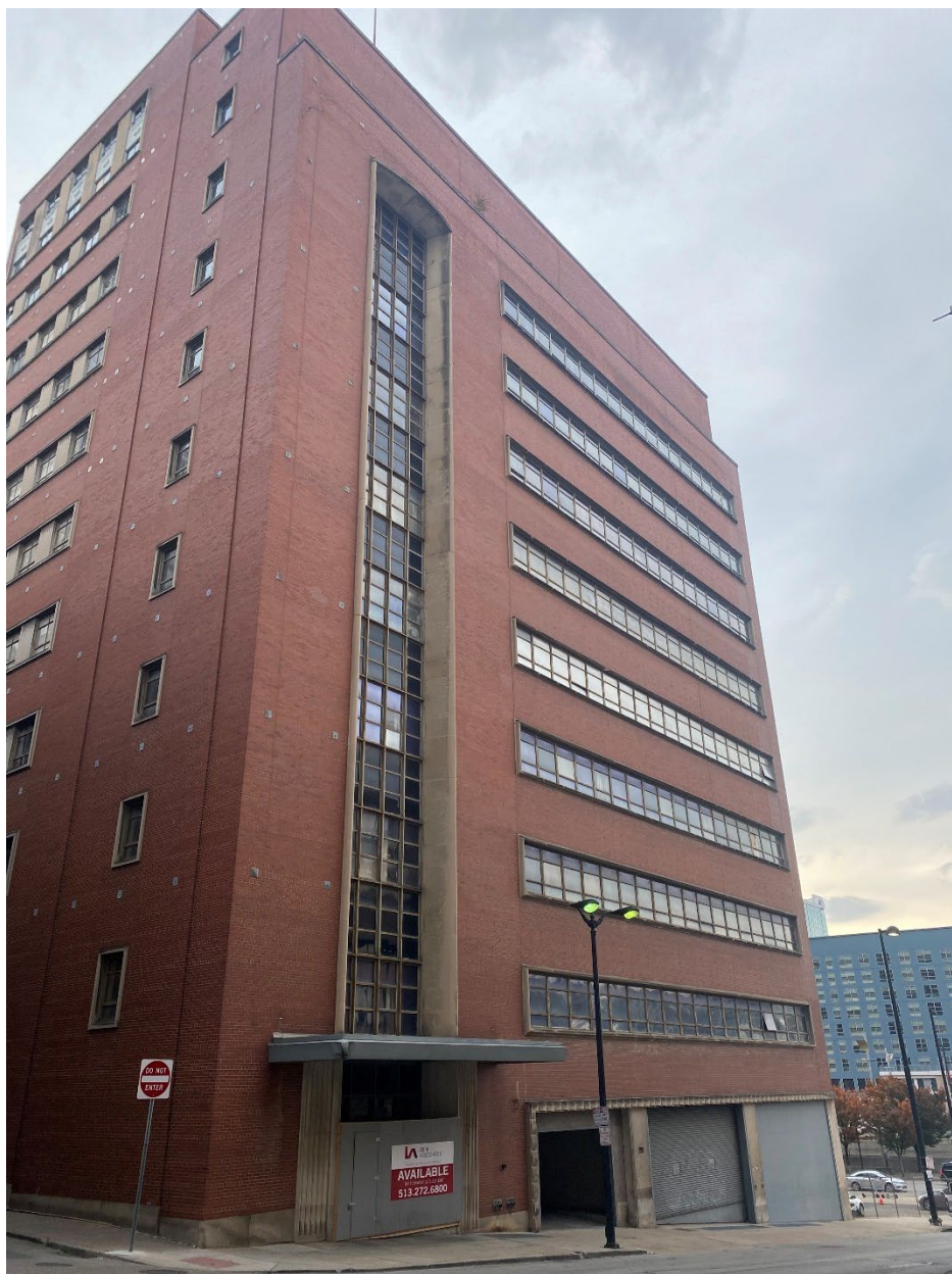
Photograph 2: Primary west elevation looking southeast.
