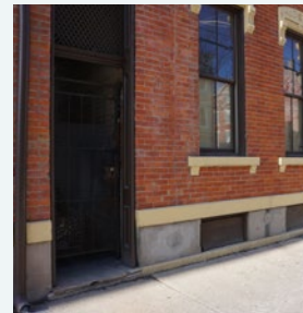
1708 Elm Street exhibits the characteristics of residential bases.
