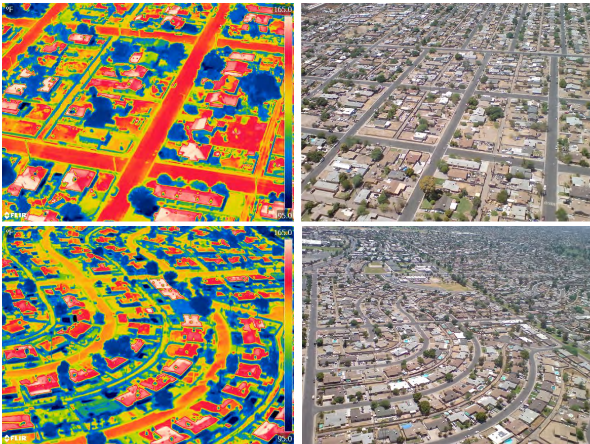
Figure 5: Conventional paving in Phoenix, taken on August 7, 2020 prior to any Cool Pavement installation. Top: District 4; Bottom: District 5. Images taken around 12–1pm, showing temperature comparisons between conventional asphalt concrete roadways, roofs, open lots, and lawns/trees.
