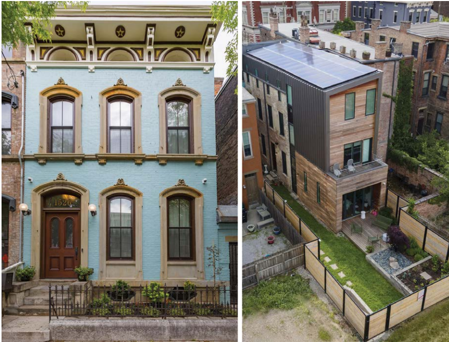
This 1870 home in Over the Rhine achieved a LEED Platinum designation by making high performance upgrades that honored the home's historic character. Photo courtesy of Sol design + consulting.
