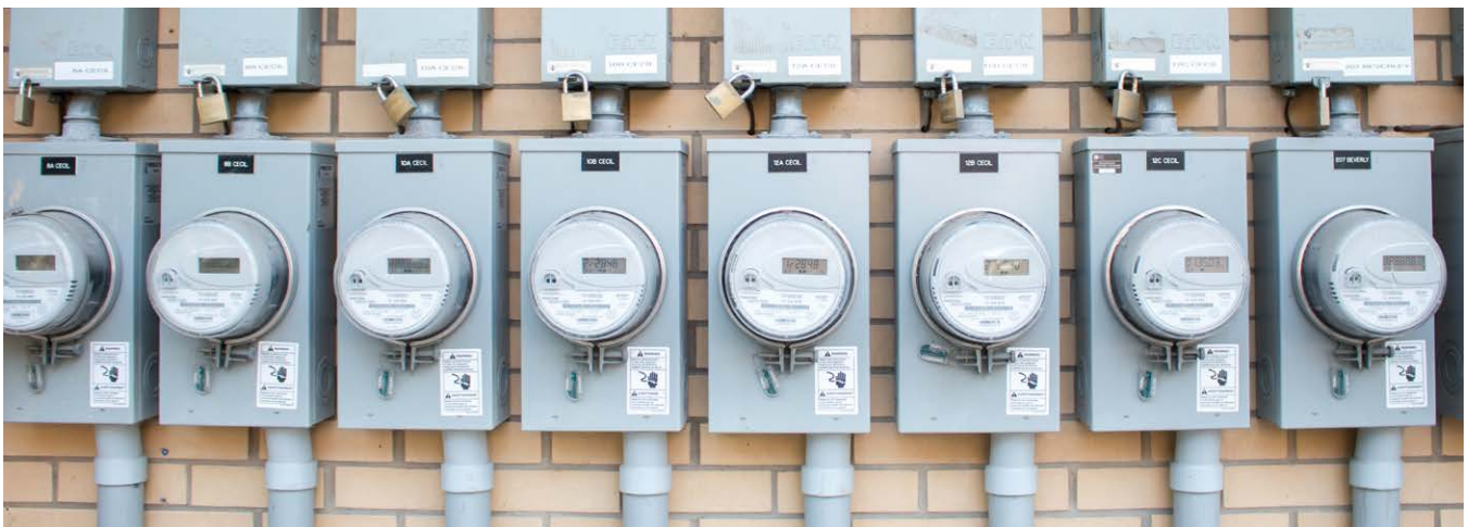
Multi-family buildings, like this 8-unit building, are often poorly insulated and energy inefficient, resulting in high energy rates and costs to residents.
