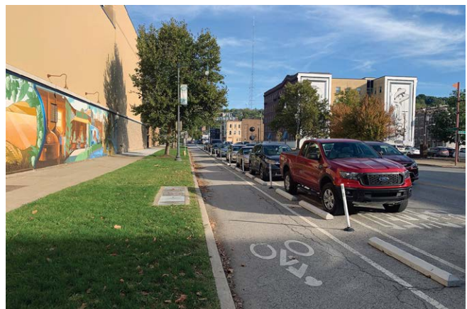
The bike lanes on Central Parkway separate cyclists from vehicles improving safety. Photo courtesy of Tri-state Trails.
