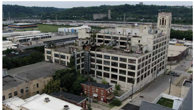
The historic Crosley building is an example of a brownfield site in Camp Washington. Clean-up of brownfield sites can revitalize neighborhoods and build healthier communities. Photo courtesy of Maddy Schmidt/WCPO.
