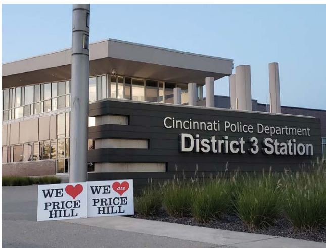
The Cincinnati District 3 Police Headquarters is Net Zero—producing all of the energy it needs to operate. Photo courtesy of Pete Witte.
