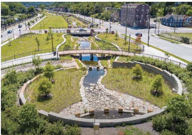
The Lick Run Greenway, completed in 2021 by Greater Cincinnati Metropolitan Sewer District, is an example of a large-scale green infrastructure project that reduces combined sewer overflows. Photo courtesy of MSD.
