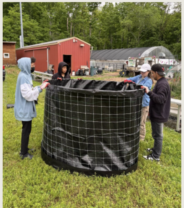
Figure 8A: Prepared outer ring – remesh wrapped in landscape fabric, secured with zip ties
