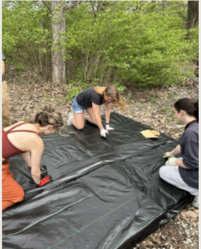
Figure 3A: Stapling fabric to pallet(s)
