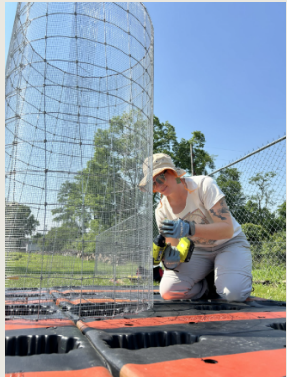
Figure 6A: Chimney remesh being wrapped in hardware cloth
