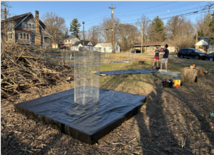
Figure 7A: Secured base by drilling 3-inch screws
