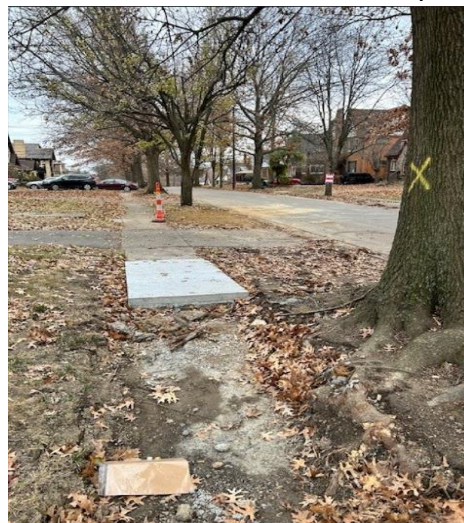
Figure 2: Sidewalk removed in Covedale, with a street tree marked for removal.
