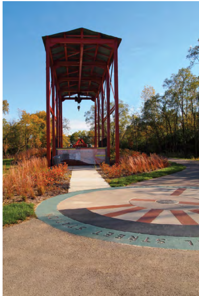
Carrel Street Station
