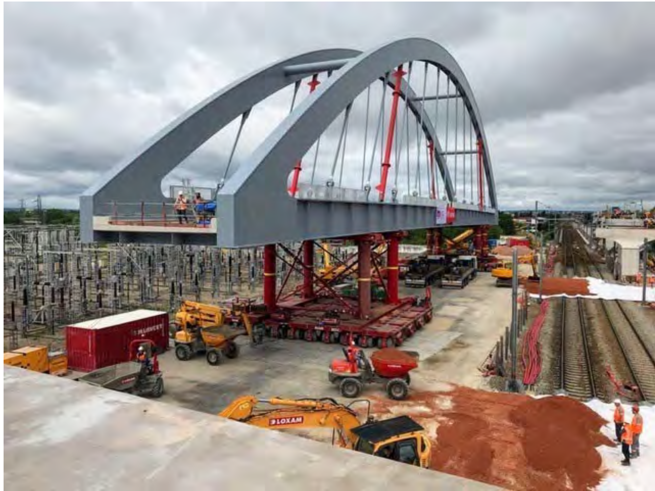
Figure 6: An Arch Bridge being transported over rail lines on SPMT's
