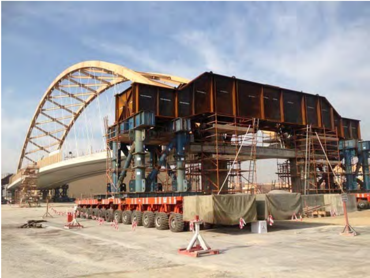
Figure 5: A Completed Arch Bridge being transported on SPMT's
