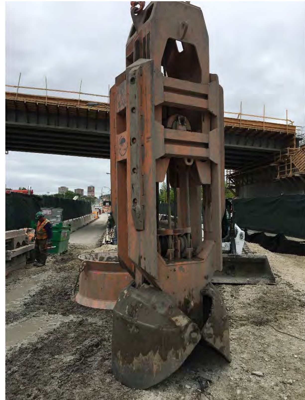
Figure 2: Clam Bucket for Excavating Caisson
