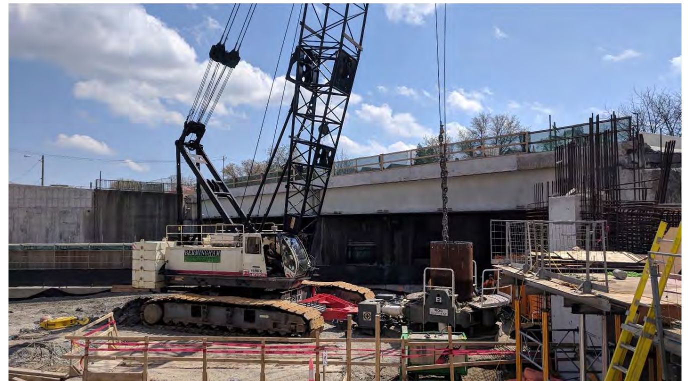
Figure 1: Close Quarters Caisson Drilling without Service Crane
