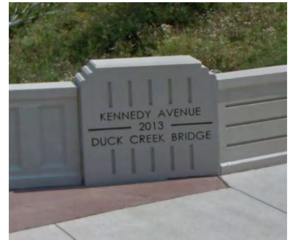
Kennedy Avenue – Duck Creek Bridge
