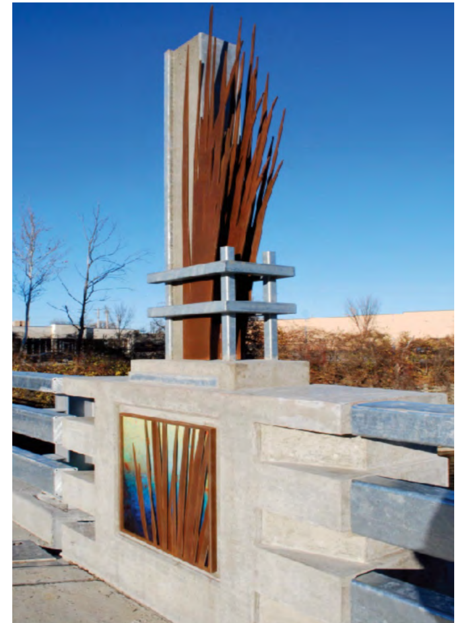
Clifton Avenue – Mill Creek Bridge
