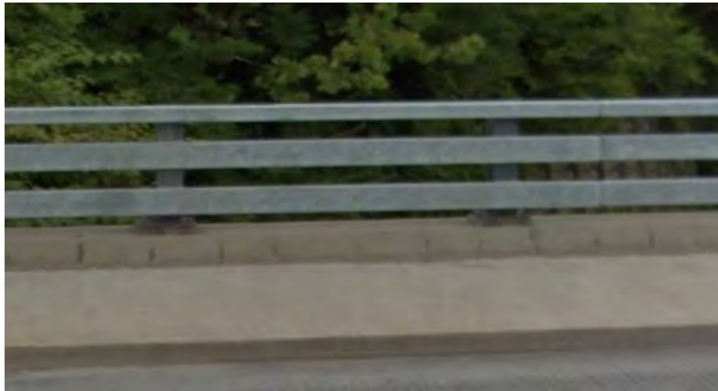
Hamilton Avenue – Hillside Railing
