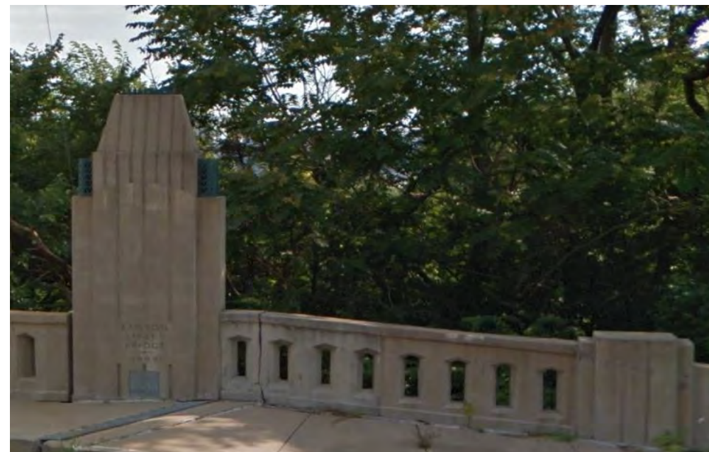
Kenton Street Bridge
