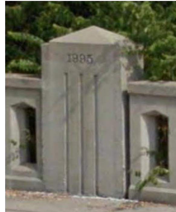
Beekman Street – West Fork Creek Bridge
