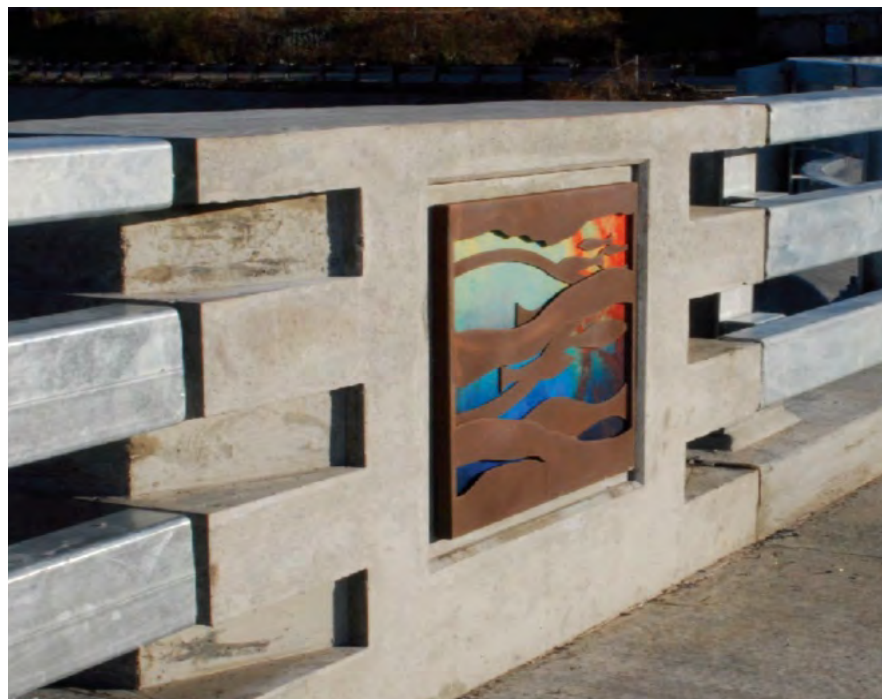
Clifton Avenue – Mill Creek Bridge
