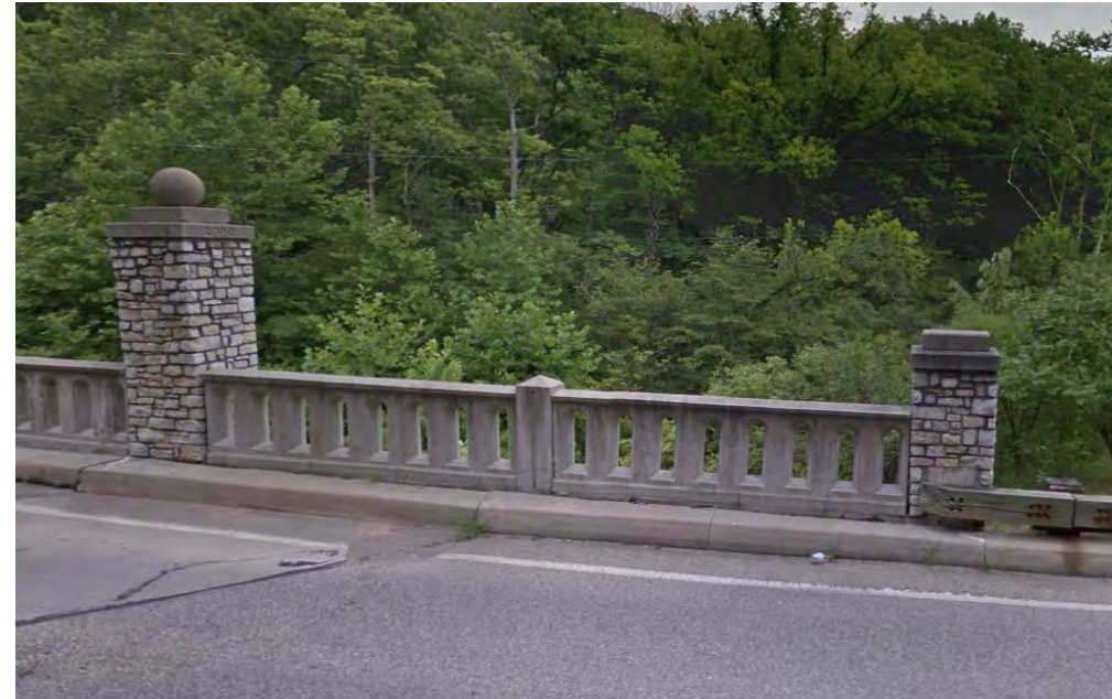
Mt. Airy – West Fork Creek Bridges
