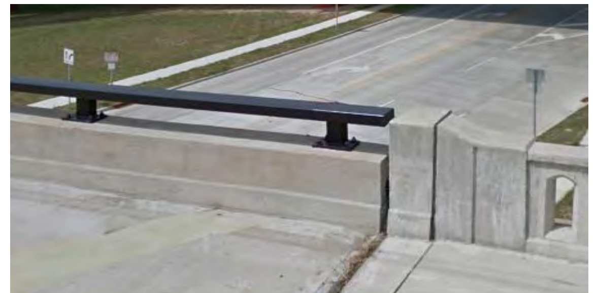
Waldvogel Gateway Ramp System Railing
