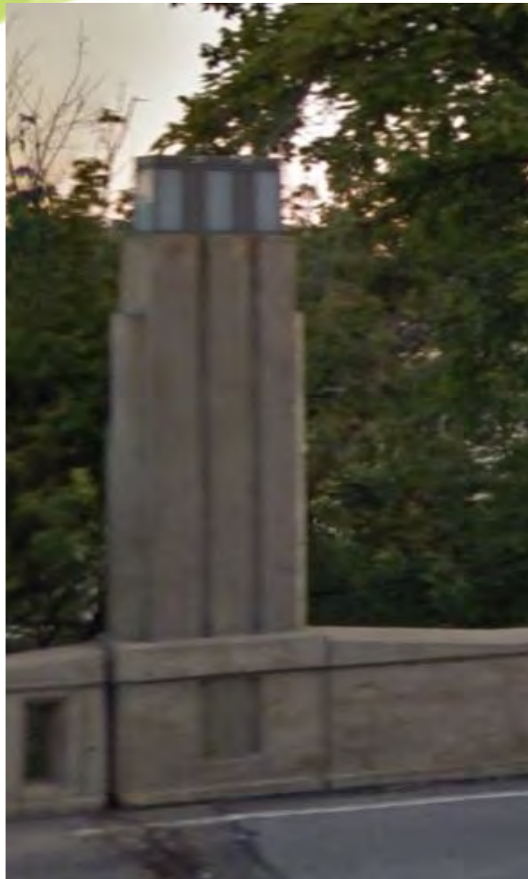
Columbia Parkway Bridges
