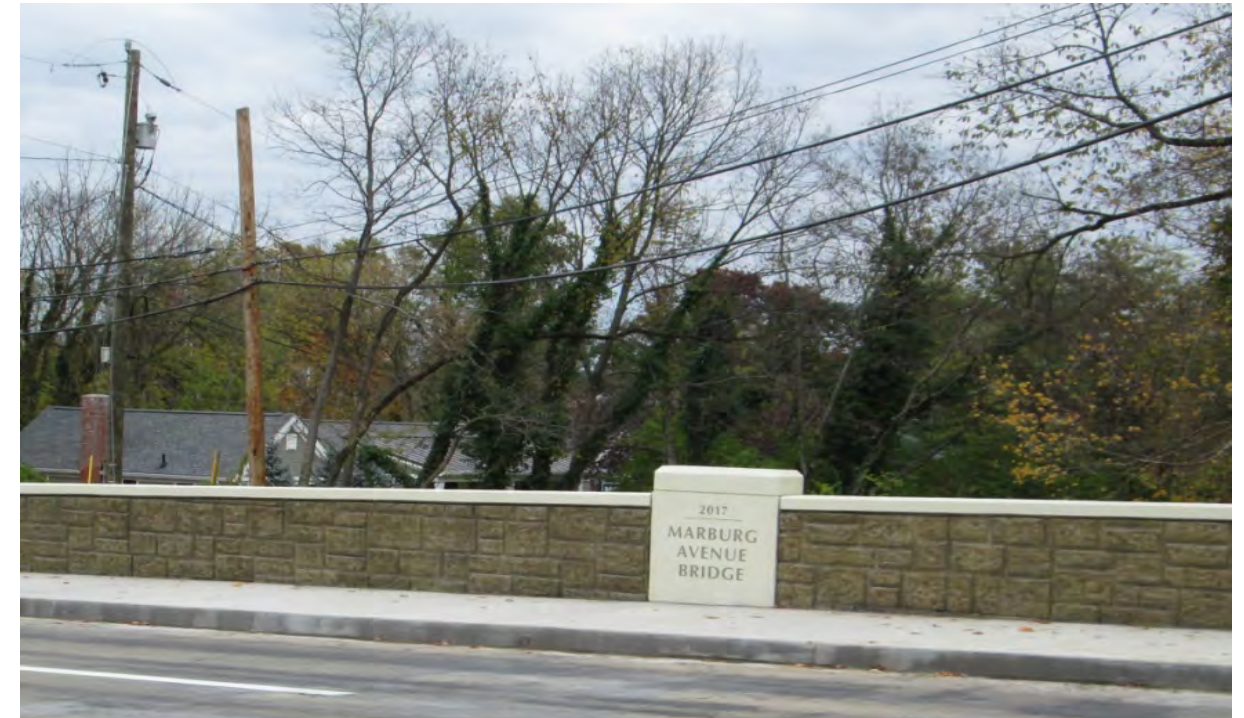
Marburg Avenue – Wasson Way Bridge Railing
