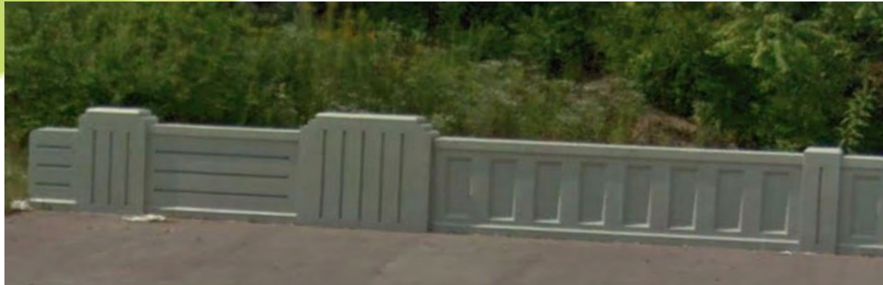
Kennedy Avenue – Duck Creek Bridge Railing
