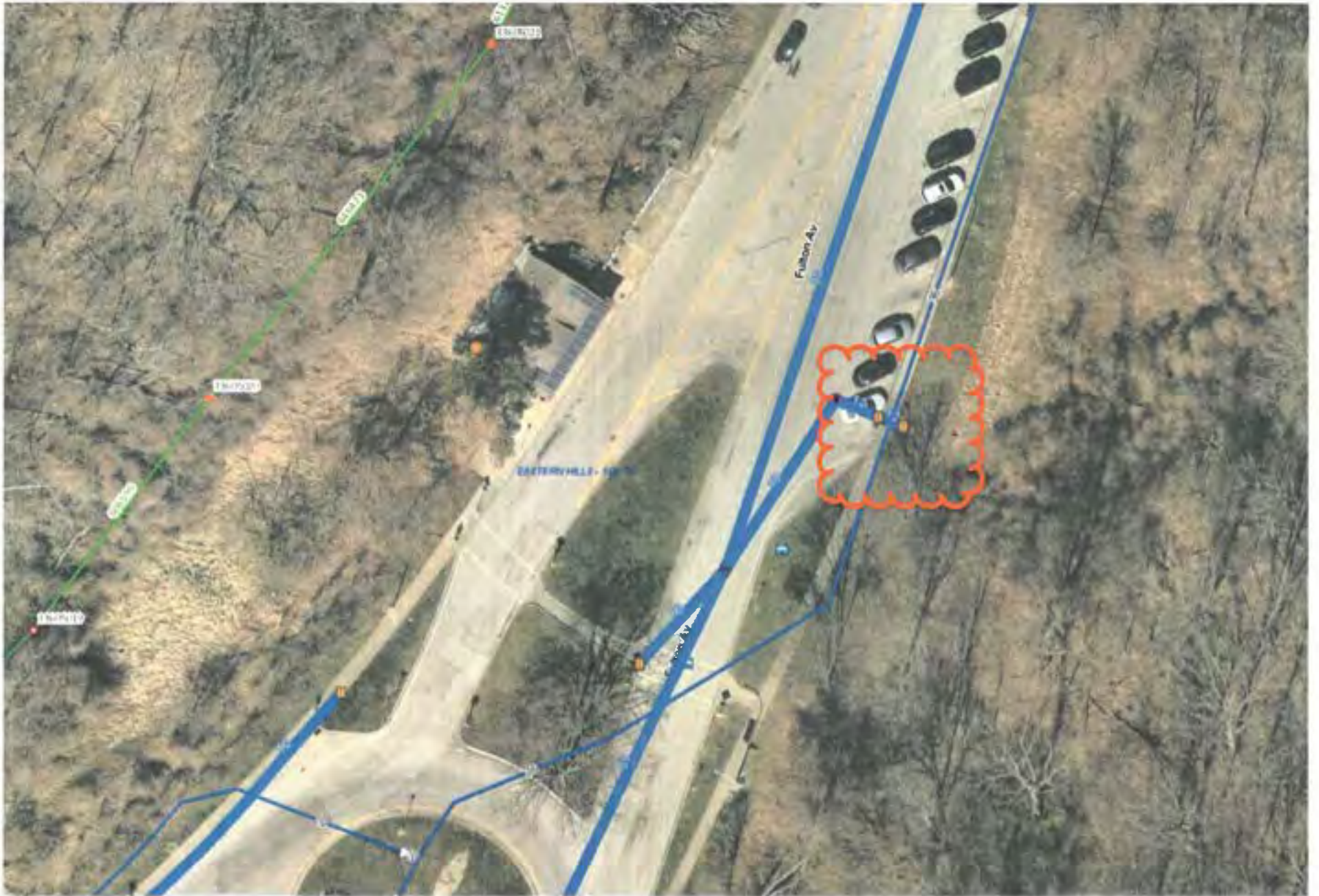
Eden Park - Fulton Comfort Station Parking Sink Hole
