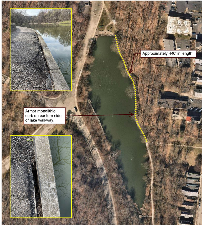
Concrete Repairs - Walkway Around Lake
