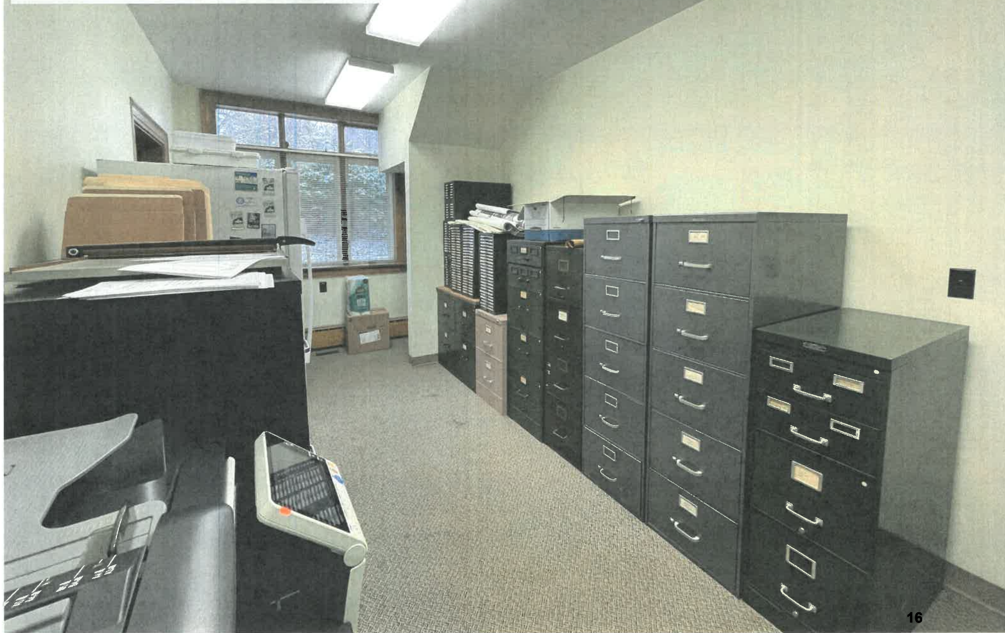
Hauck House - Original Kitchen - to be Renovated into Kitchenette / Team Break Room
