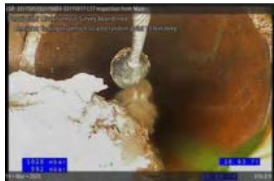
Miscellaneous Survey Abandoned at 010.0 ft | Ending inspection located random point 13 feet deep.
