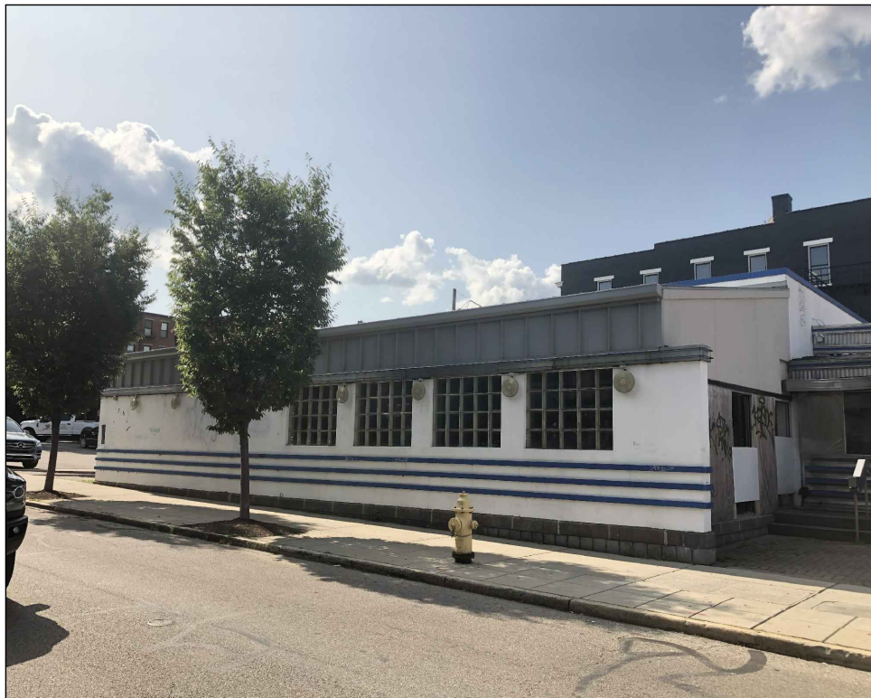
1203 SYCAMORE: SOUTH FACADE
