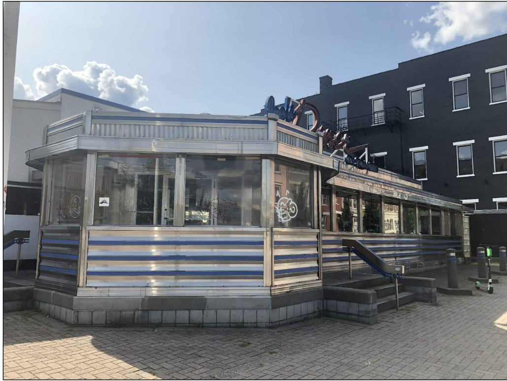
1203 SYCAMORE: ENTRY AND EAST FACADE
