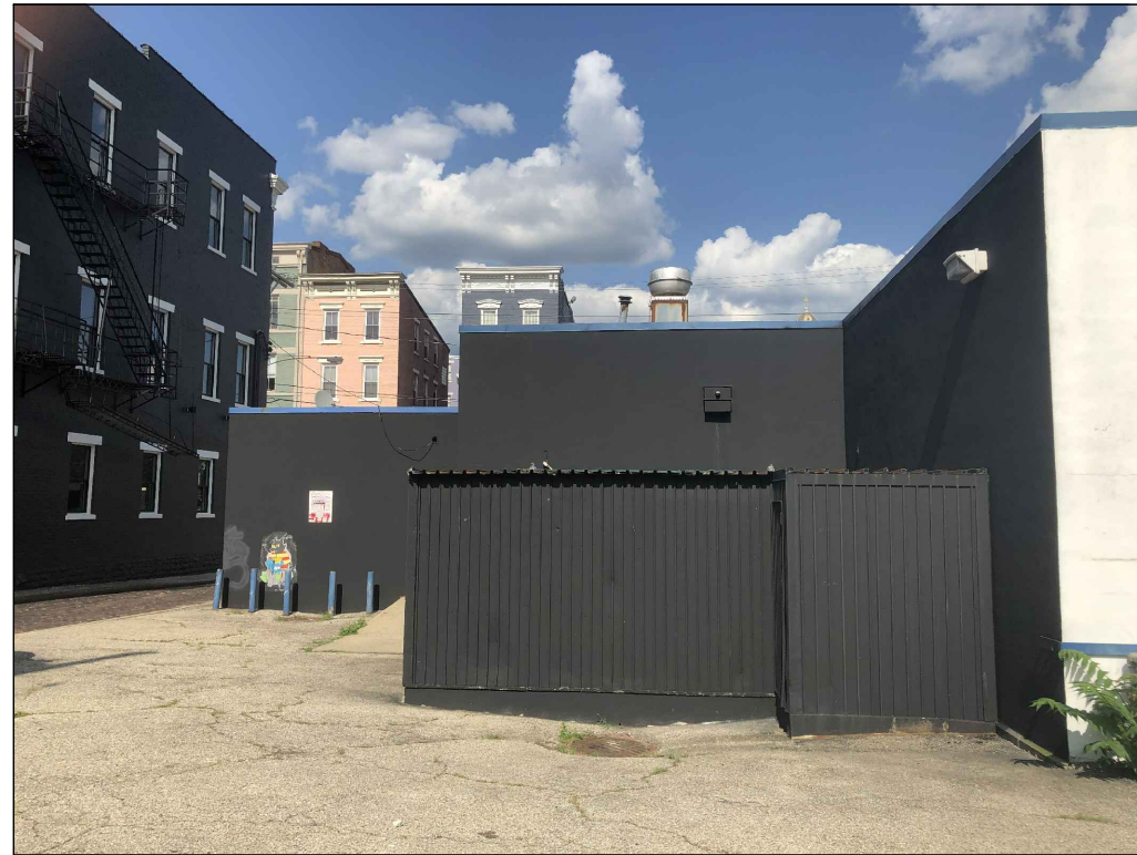
1203 SYCAMORE: NORTHWEST CORNER
