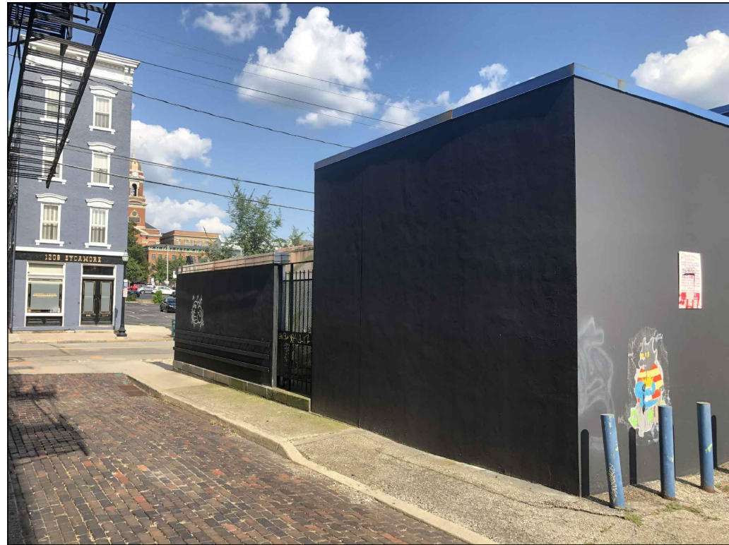
1203 SYCAMORE: NORTH FACADE & GREAR ALLEY
