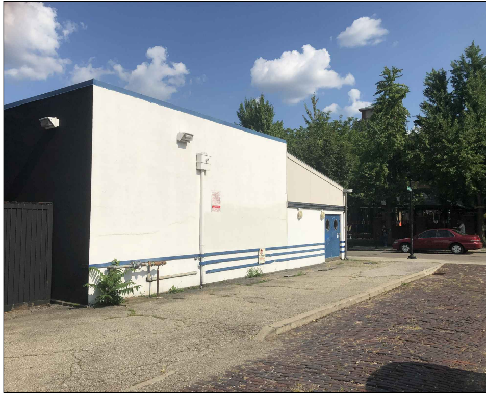
1203 SYCAMORE: WEST FACADE (FUTURE PATIO) & COGSWELL ALLEY
