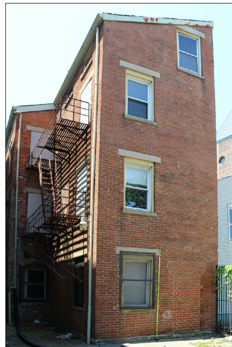
D: CLYMER ALLEY EXISTING FACADE
