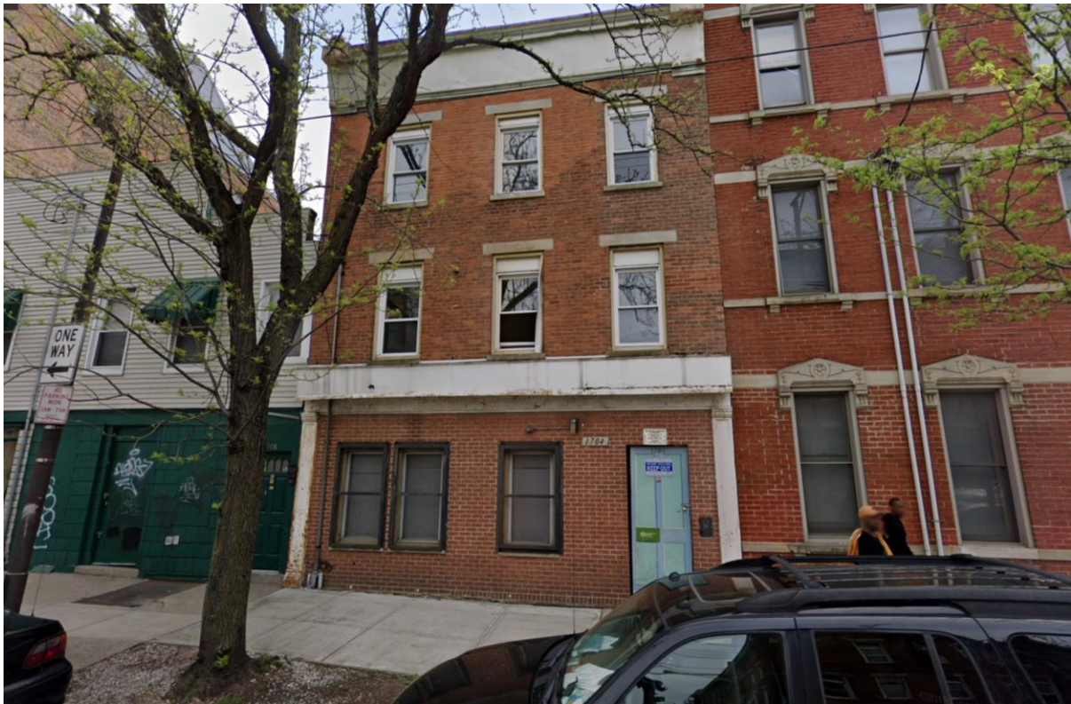
Figure 2. Image of 1704 Elm Street. Image from Google.
