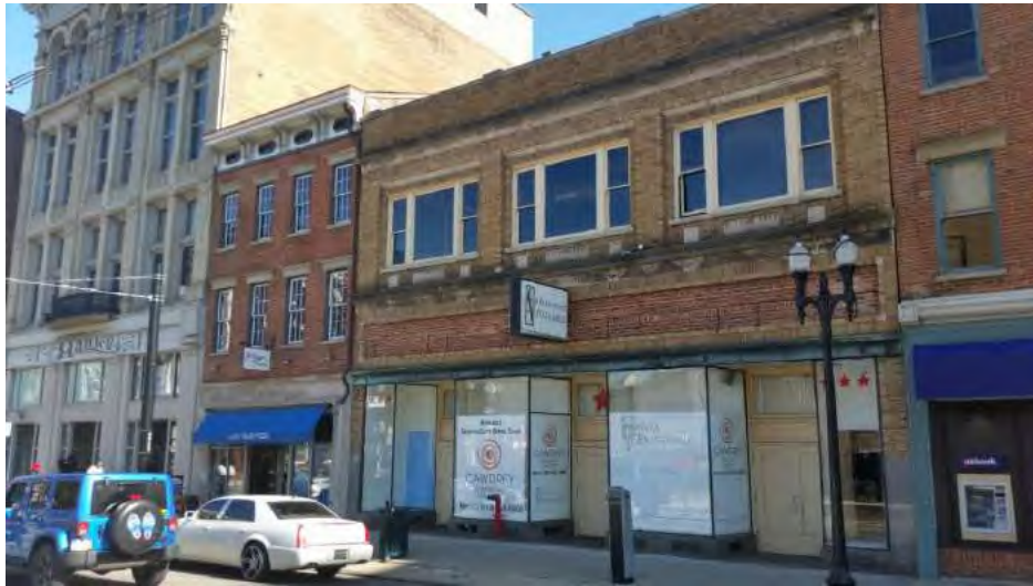
Figure 2: Picture of 1120 Main Street from the street provided by the applicant.
