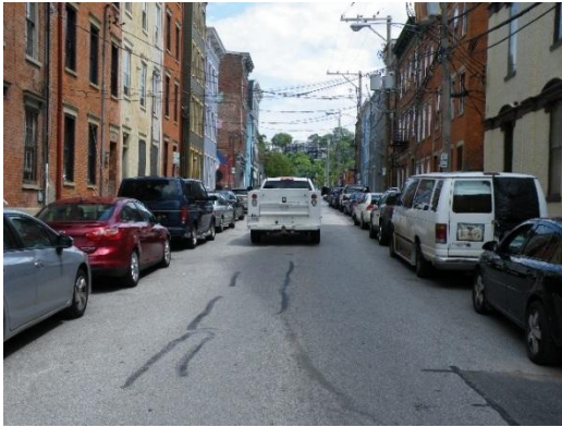
12 th St. narrow one lane for traffic
