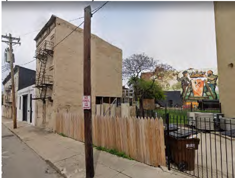
Figure 1: 112 Corwine St. Image from google street views.
