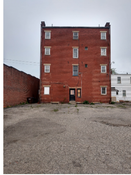
3 EAST - REAR FACADE
