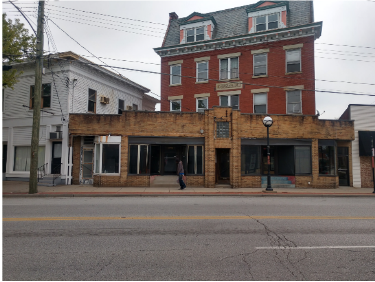
1 WEST - FRONT FACADE
