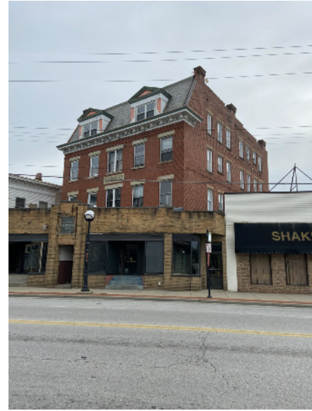
2 SOUTH - SIDE FACADE
