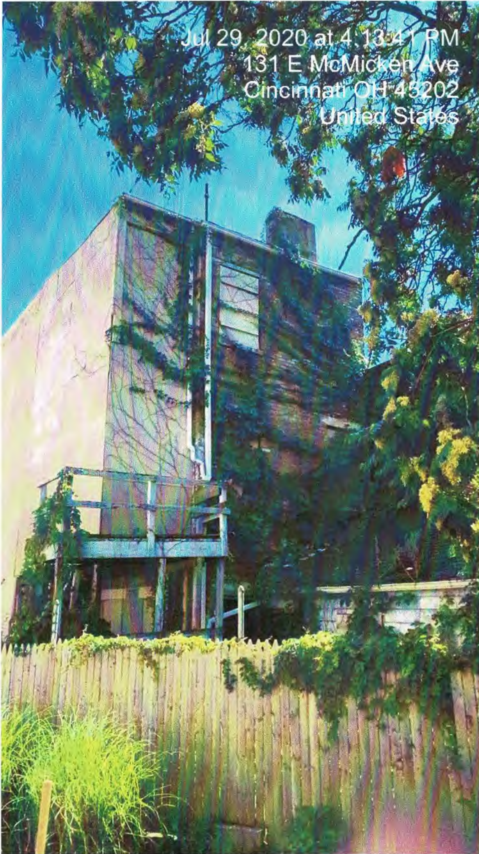
112 Corwine ( Rear View : South )
