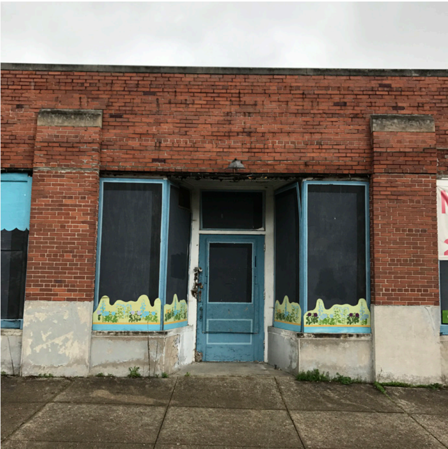
Existing front Entry w/ painted plywood "windows"
