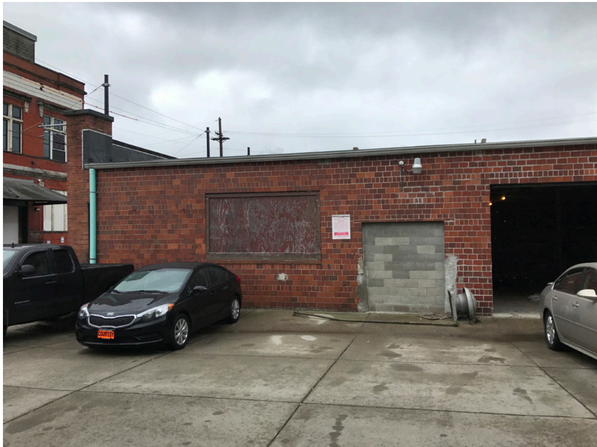
Rear of Building (East Elevation) - side closest to Henry Street
