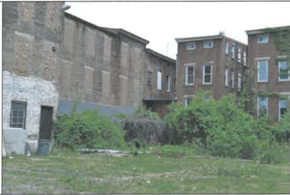
SOUTH FACADE FROM OPEN LOT
