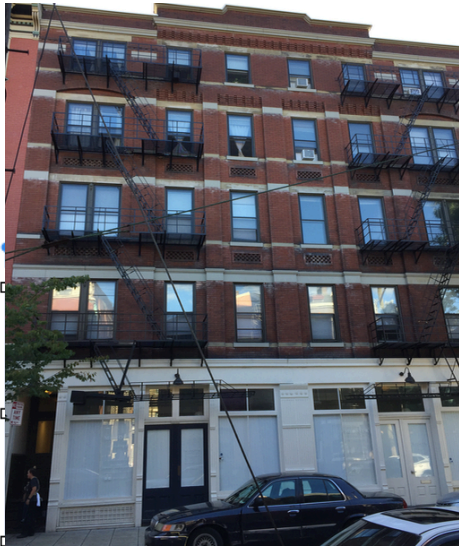
OTR Community Housing - built in 1897, all incomes are for people below 50% of median local income
