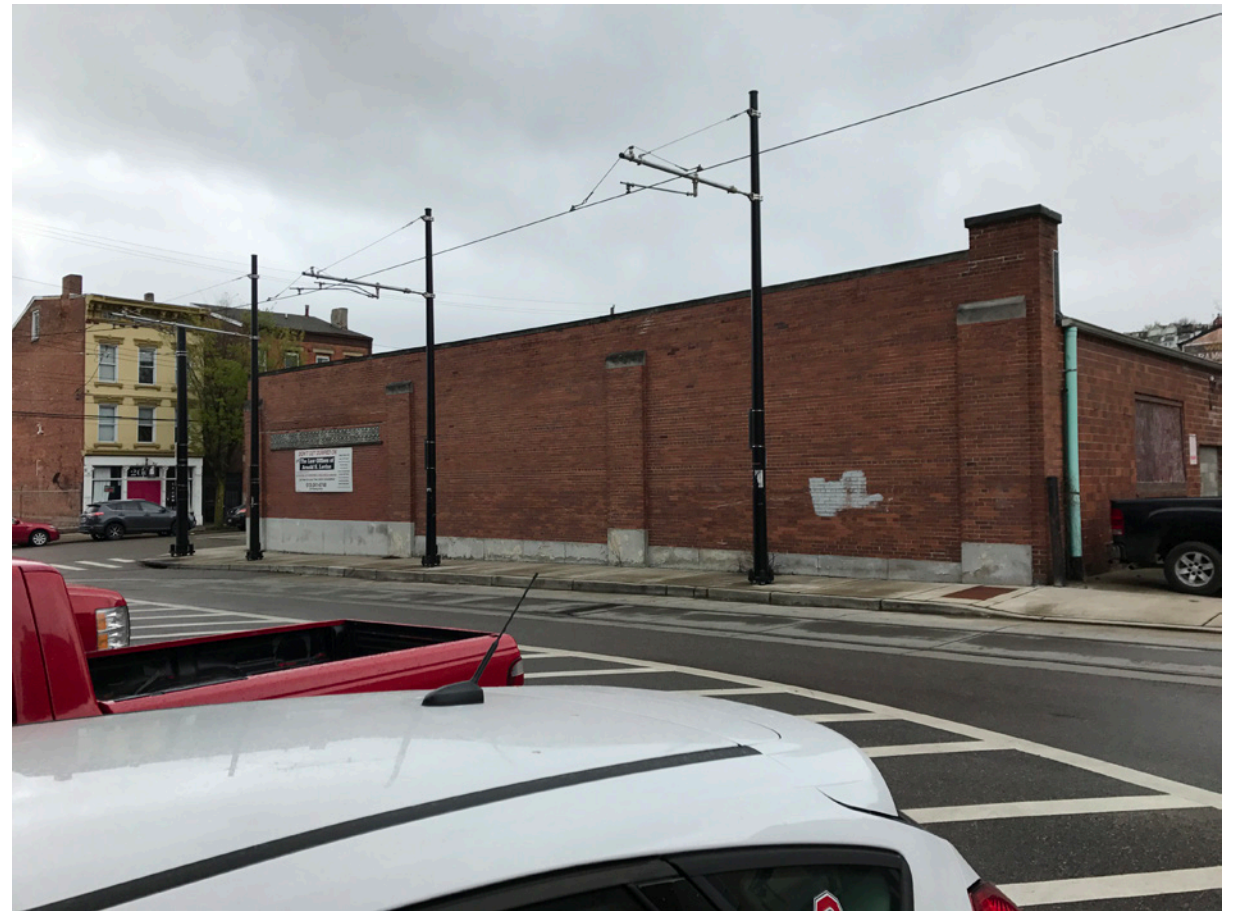
Side of Building along Henry Street (South Elevation) - view from SE
