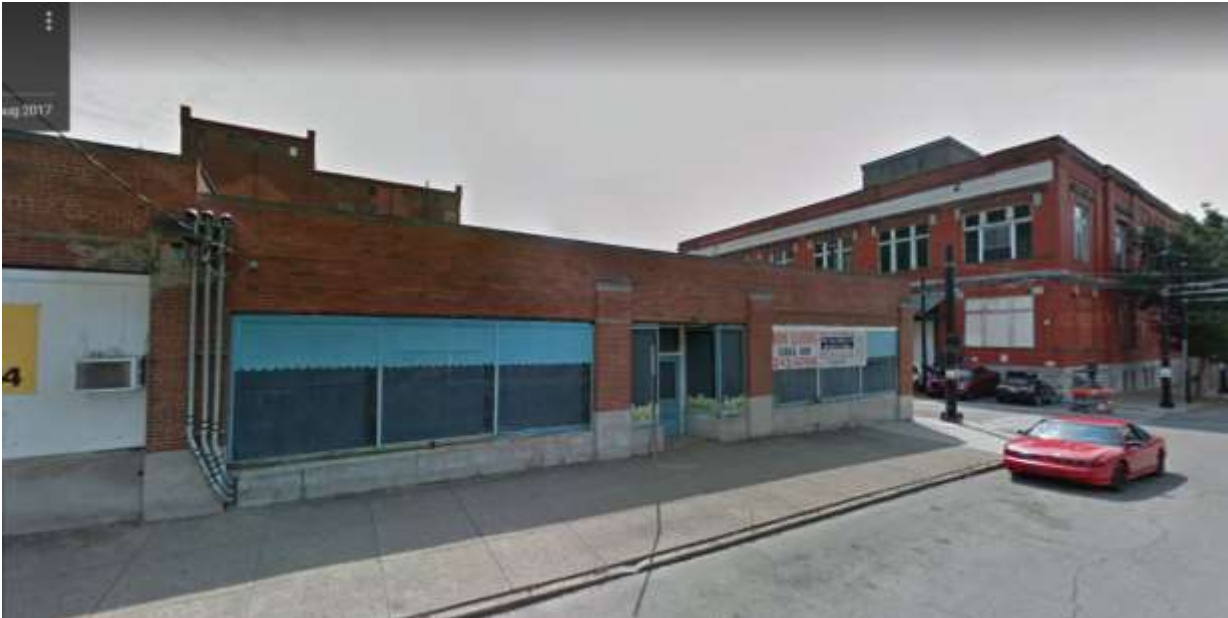
Figure 2: Front facade of existing 2010 Elm Street
