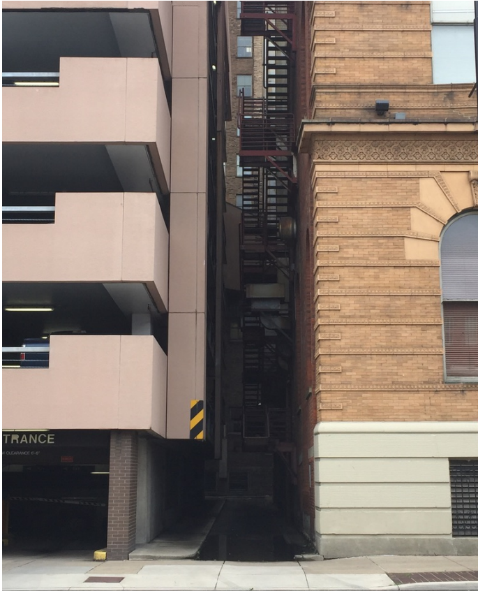
BALDWIN ALLEY FROM 9TH TO 8TH WITH MULTI-STORY CAR PARK
