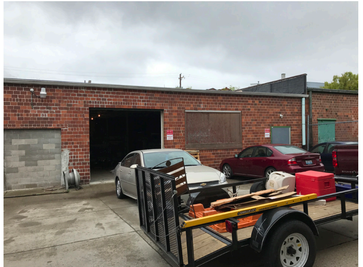
Rear of Building (East Elevation) - side closest to adjacent building
