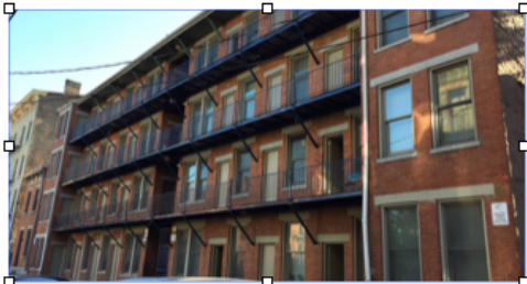
Section 8 low-income housing subsidized by HUD, built in 1883
