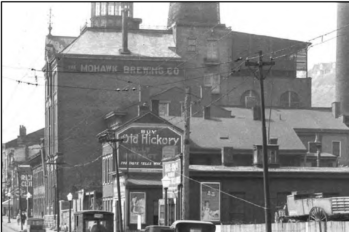
Figure 4. Image of subject property ca. 1927 showing rooftop appurtenances. Photo provided by applicant.
