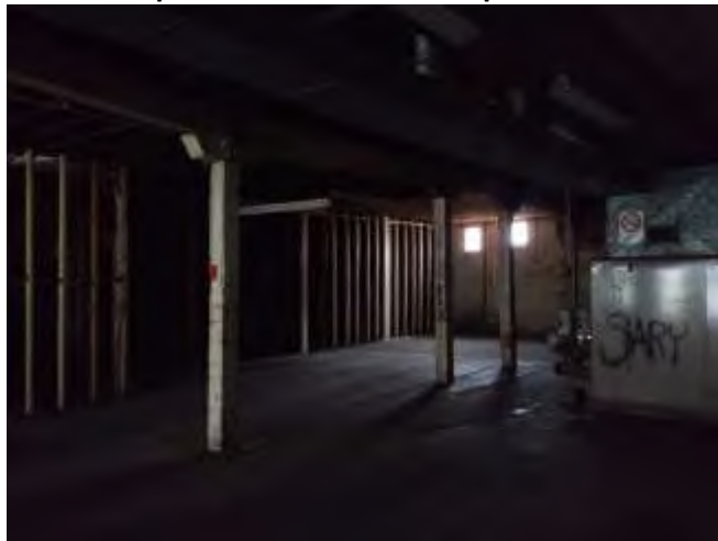
E - Interior photos of 1902 Colerain post stabilization (December 2017)
