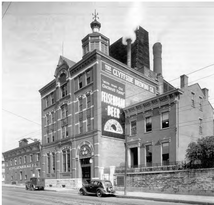
Figure 5. View of 244 W. McMicken Avenue, Showing 1845 Brewery Building (left) and Brew House (middle), c. 1935
