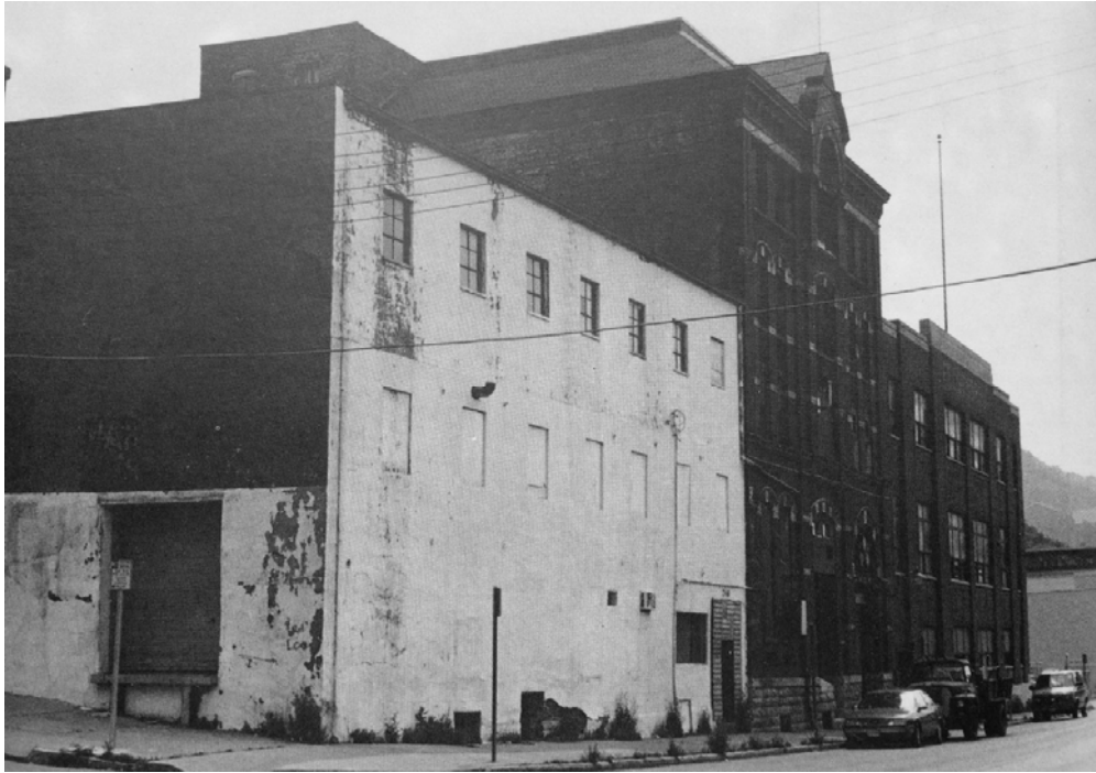
Figure 8. View of 244 W. McMicken Avenue, Showing Altered 1845 Sohn Brewery Building (left) and Wash House (right) c. 1989
