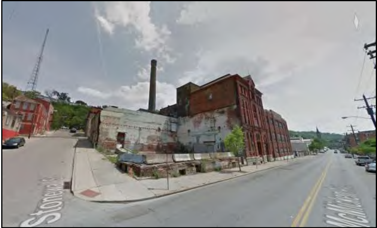
Figure 2. Condition of 244-246 W. McMicken Ave ca. May 2018. Image courtesy of Google.
