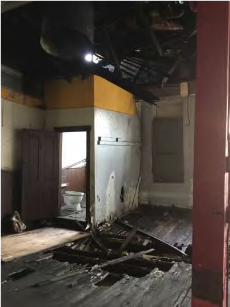
F - Interior photo of 1902 Colerain pre stabilization
