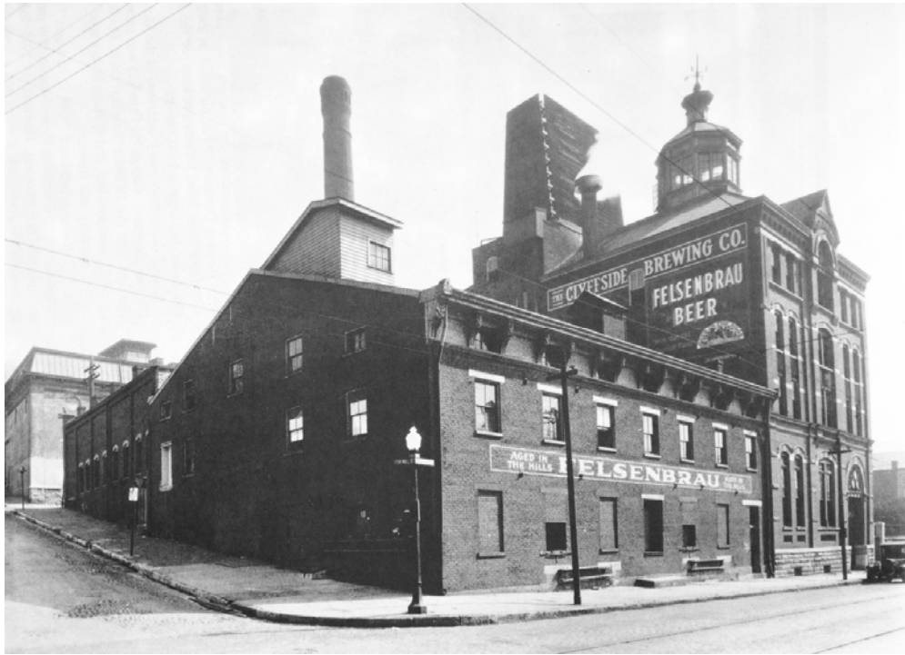
Figure 4. View of 244 W. McMicken Avenue, Showing Wash House, 1845 Brewery Building and Brew House (left to right), c. 1935
