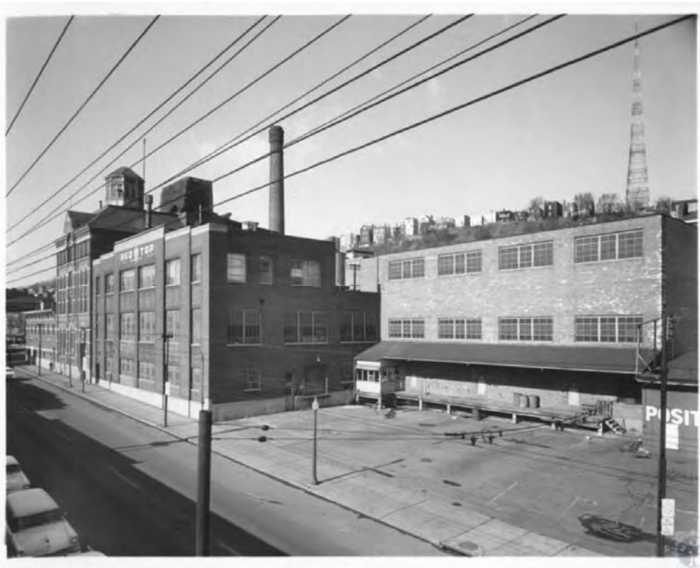
Figure 7. View of 244 W. McMicken Avenue, post 1956
