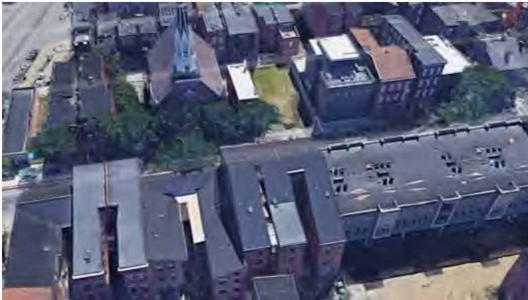
Figure 1: Street view of 1518 Race Street. Pictures provided by Google Street Views.
