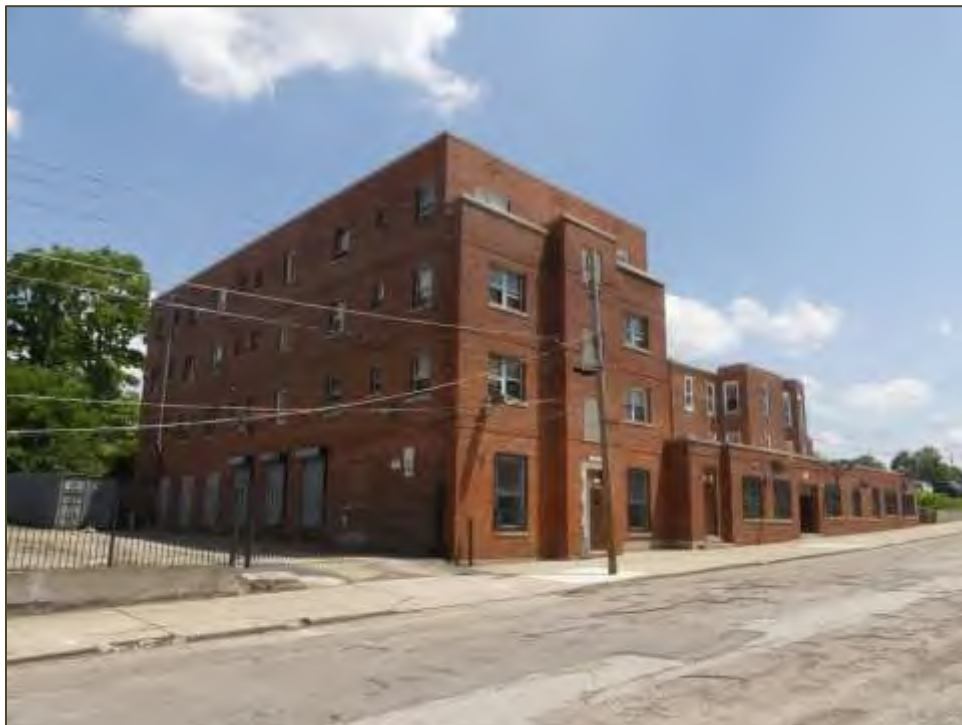
Manse Hotel, north and west elevations.
