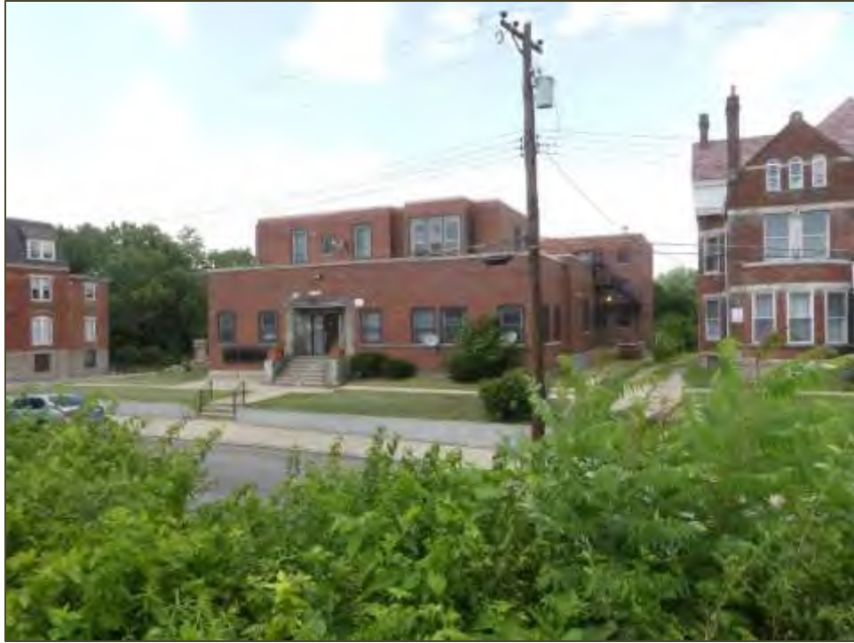
Manse Hotel, east and south elevations.
