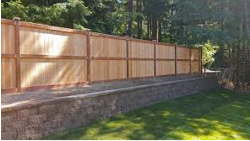
Privacy fence above retaining wall
