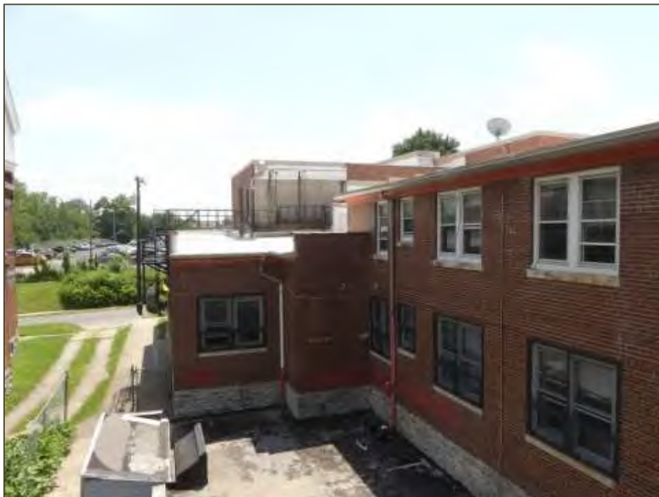
Manse Hotel, east elevation, looking south
