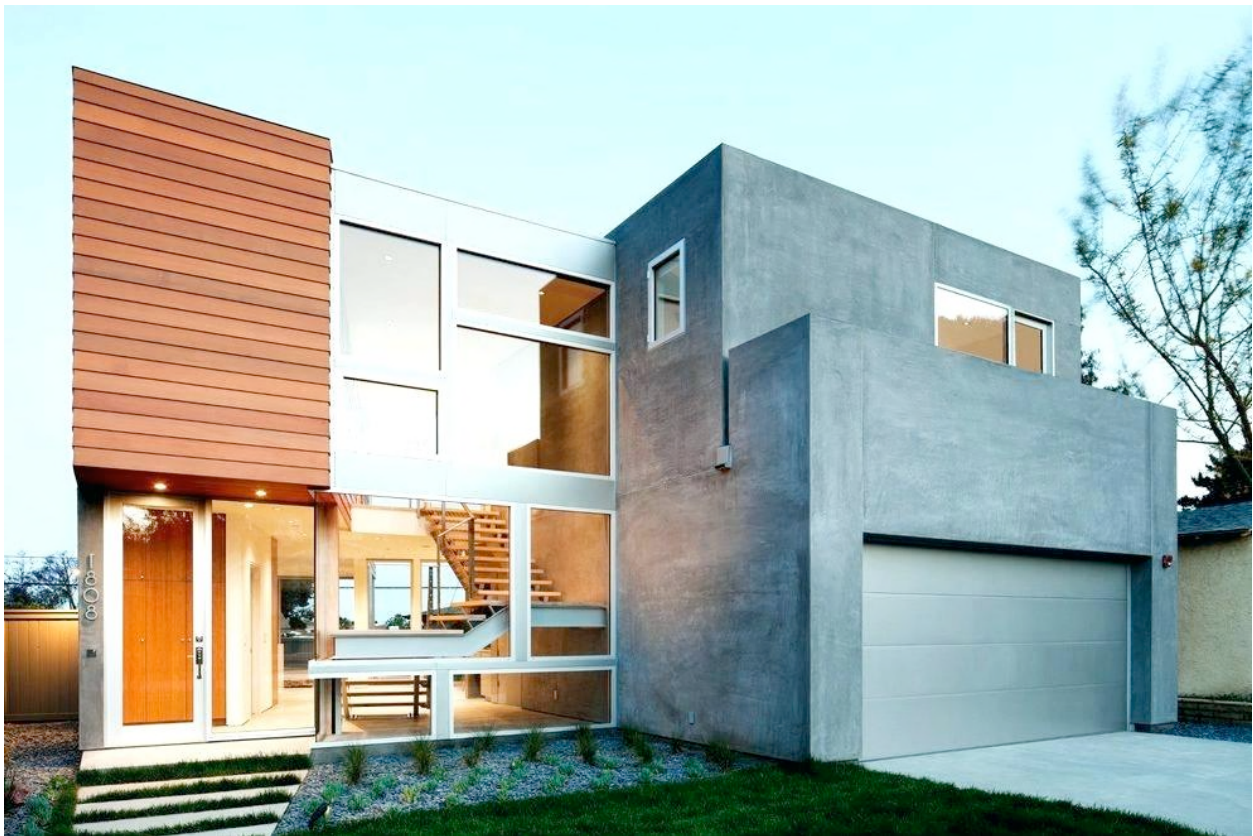
smooth stucco over CMU
