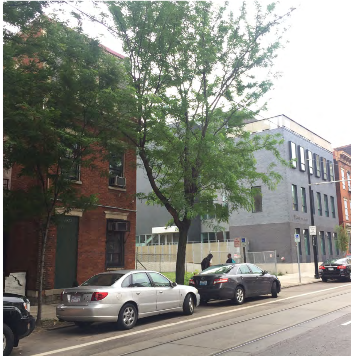
FRONT-OF-SITE PHOTO - Looking SE
