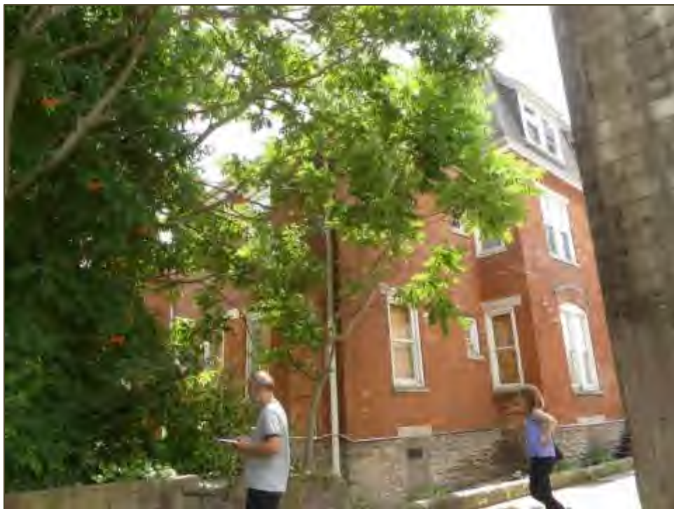
Manse Hotel Annex, west and north elevations.
