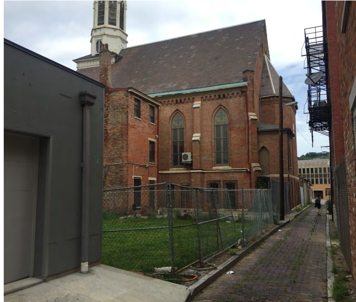
REAR-OF-SITE PHOTO - Looking NW
