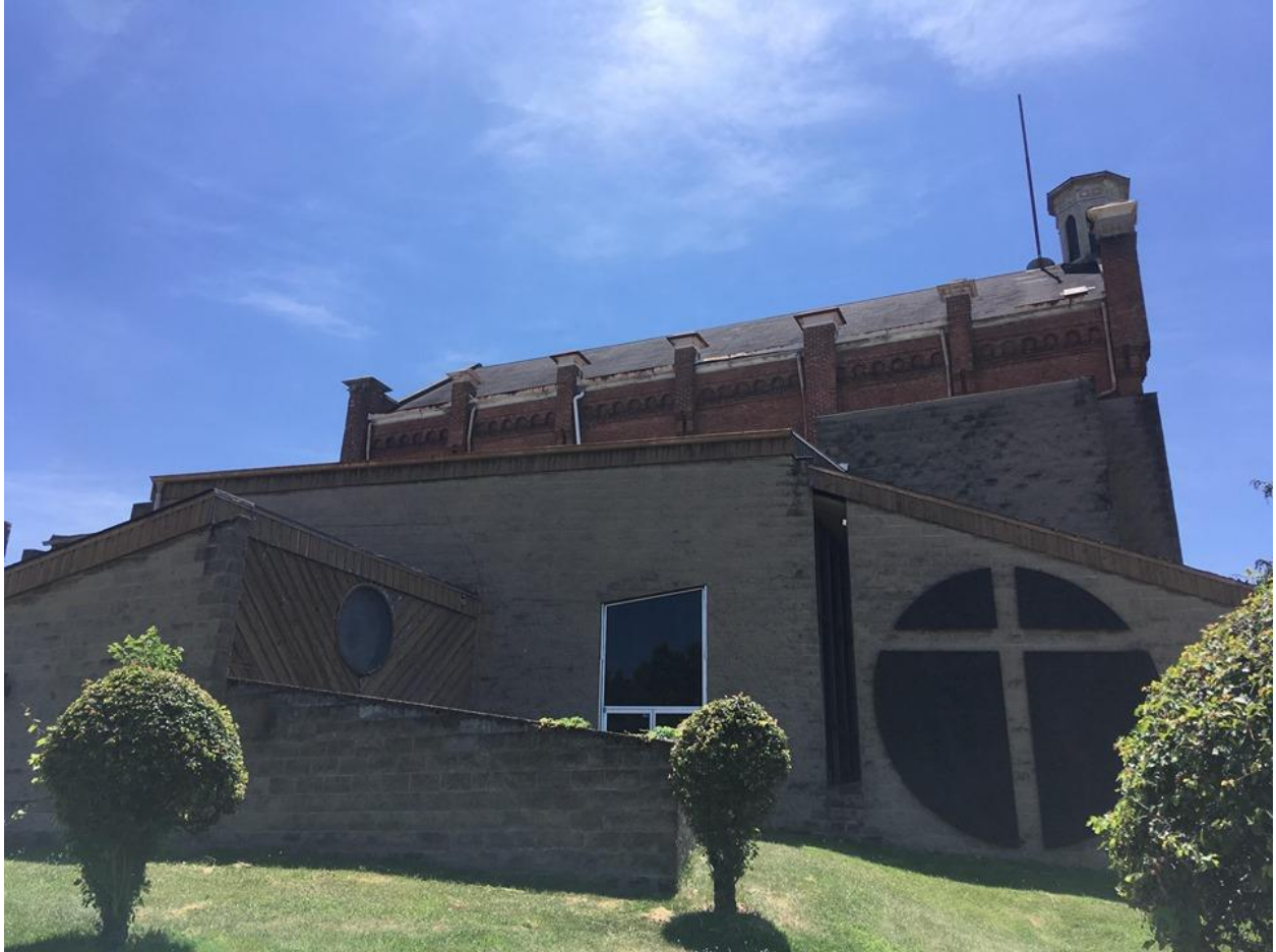
Figure L: Liberty Street (north) façade
