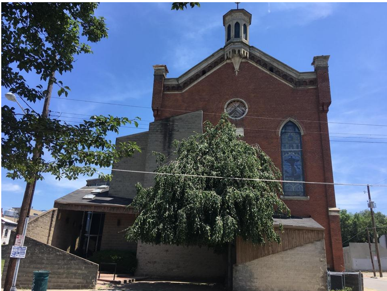
Figure 1: John Street (west) facade
