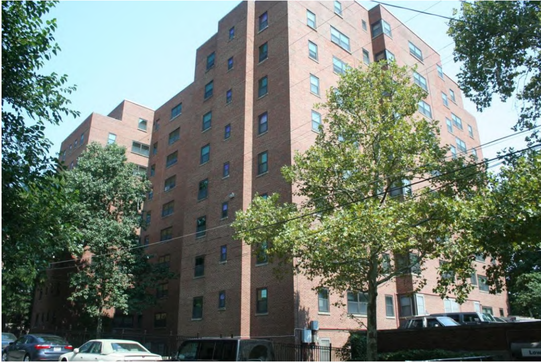
3700 Reading Road, South and Rear (East) elevations
