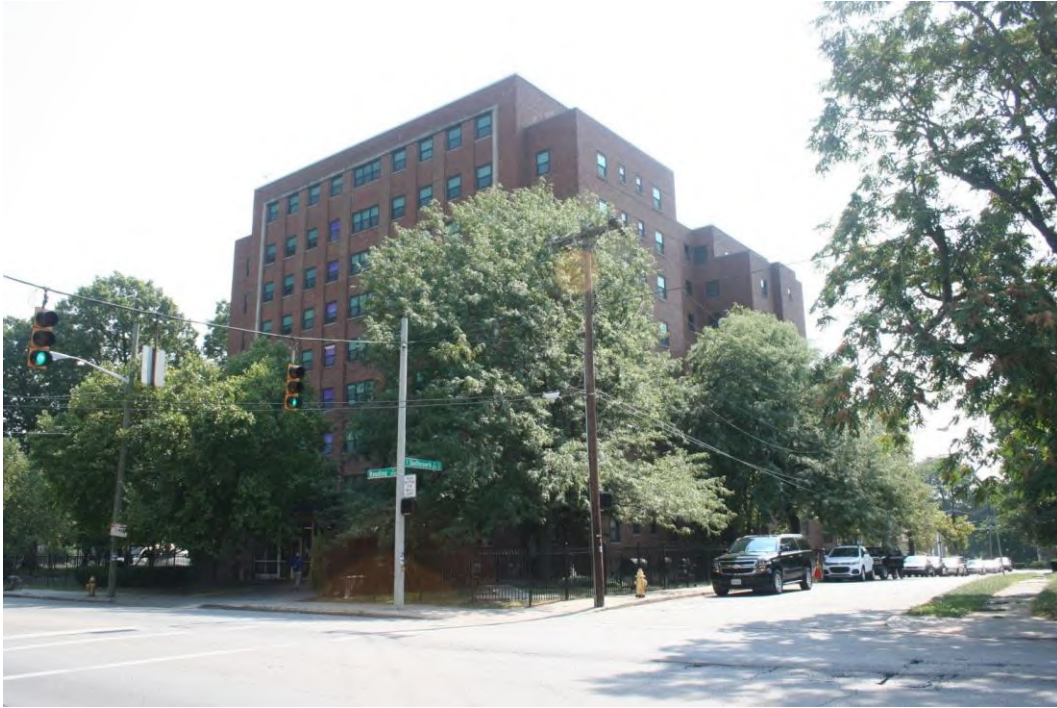
3700 Reading Road, Front (West) and South elevations
