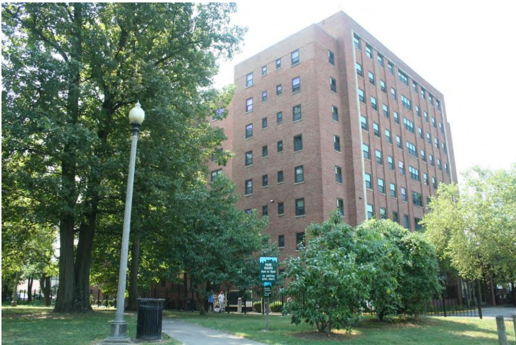
3700 Reading Road, North and East (Front) elevations
