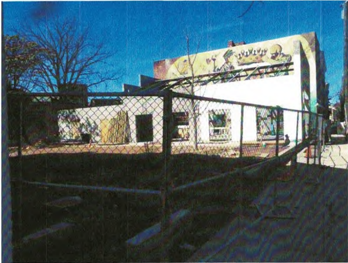
Figure 1. Existing Site : Southeast Corner
