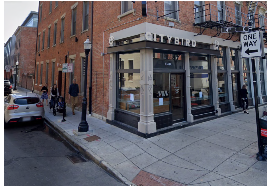
Corner of Vine & 14th (deep set storefront, returns one bay with wrapping awning)
