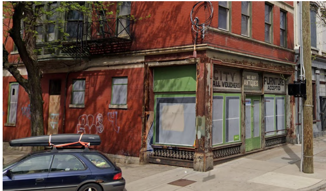
Corner of Race and Green (deep set storefront with cast iron frame, returns one bay)
