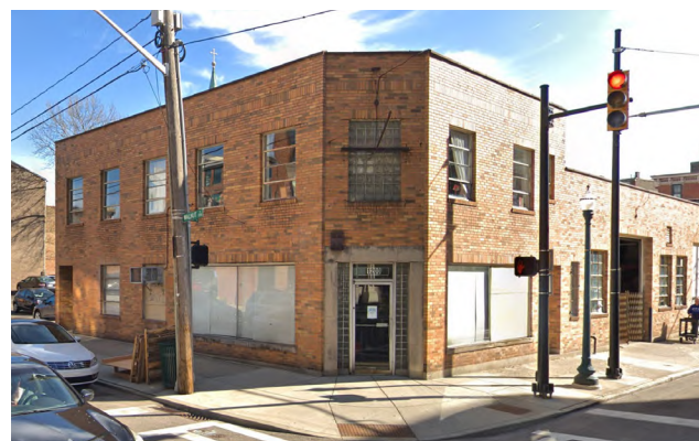
2 story at corner of 12th and Walnut
