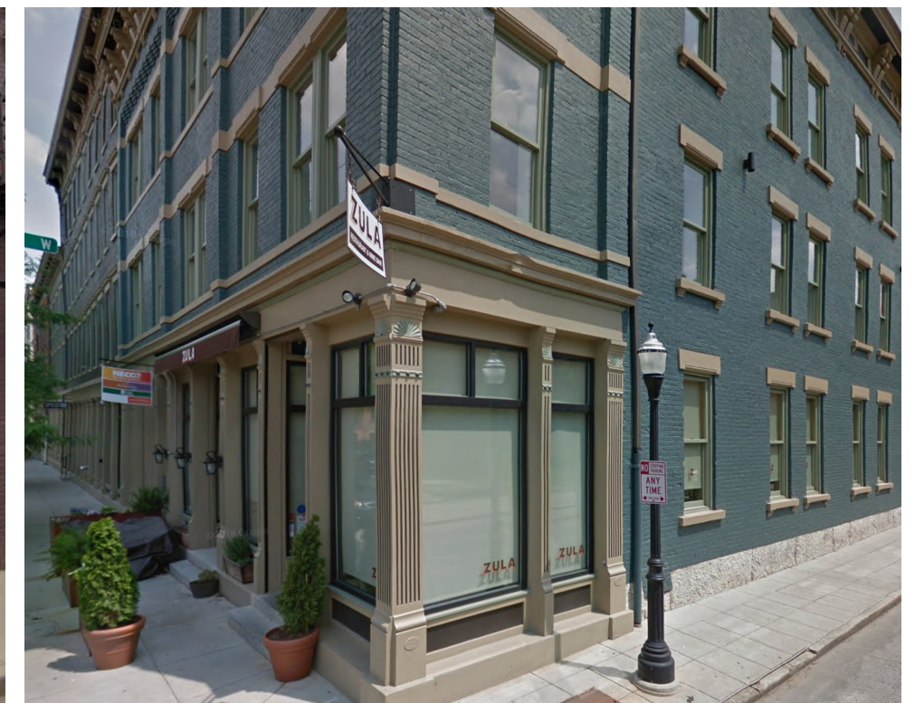
Corner of 14th & Race (deep set storefront with cast iron piers, returns two bays)
