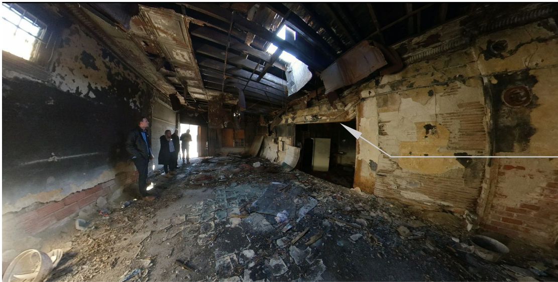
FORMER DRY CLEANERS (NORTHERN MOST BAY) LOOKING EAST
