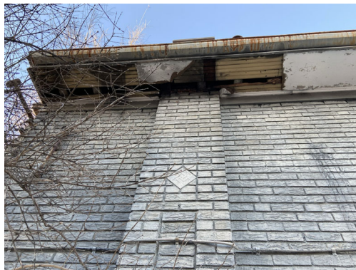
EAVE AND GUTTER - SOUTHWEST CORNER
