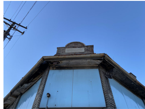
EAVE AND GUTTER - SOUTHEAST CORNER
