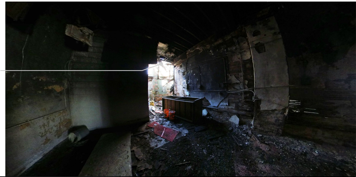
ENTIRE SECTION OF ROOF AND STRUCTURE COLLAPSED LEAVING REAR EXTERIOR WALL COMPLETELY EXPOSED
