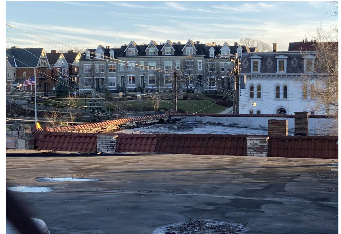
VIEW OF ROOF CONDITION FROM ESTELLE STREET
