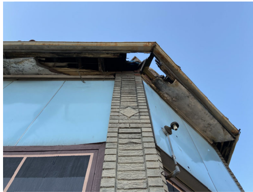
EAVE AND GUTTER - SOUTHEAST CORNER
