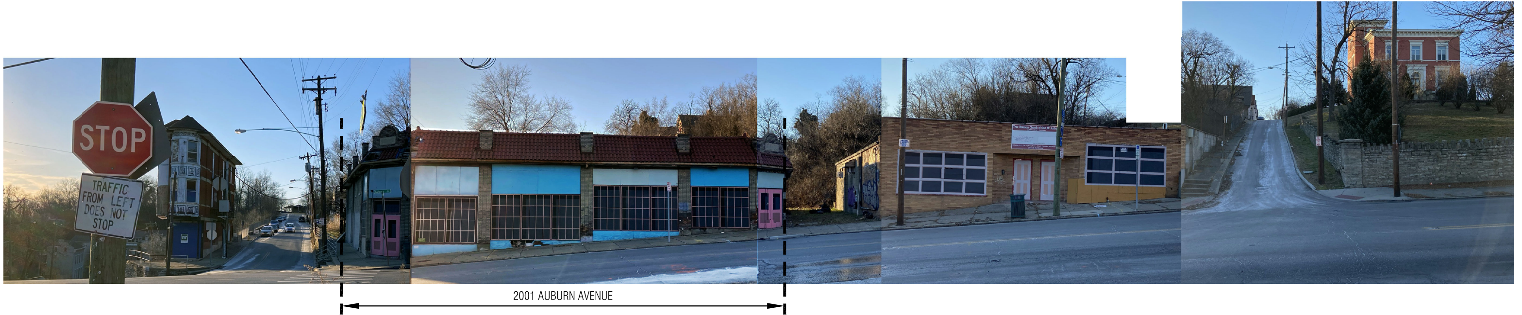
EXISTING PHOTOS ALONG AUBURN AVENUE LOOKING WEST
