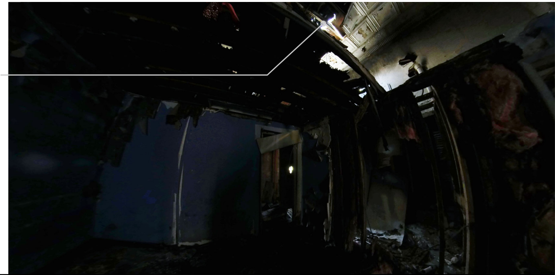
LARGE AREAS OF ROOF COLLAPSE BEYOND CEILING THIS ROOM LEAVING STRUCTURE OPEN AND DETERIORATING
