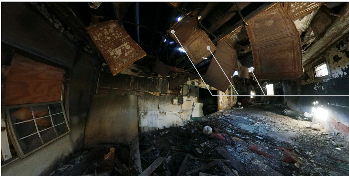
FORMER DRY CLEANERS (NORTHERN MOST BAY) LOOKING WEST
