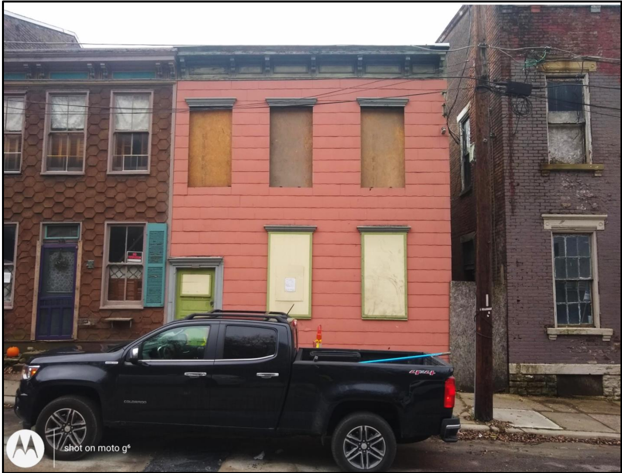
Figure 3: Current conditions of subject property, facing south. Image from applicant.
