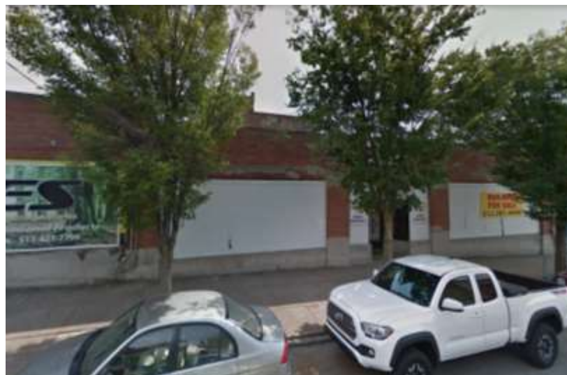
Figure 2: Front facade of existing 2014 Elm Street
