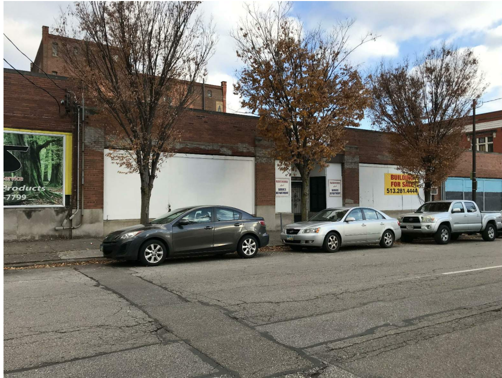
1. FRONT VIEW - NW
