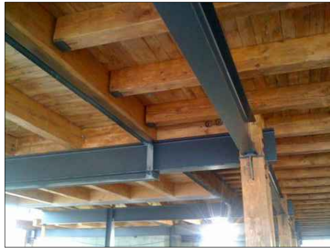
2 WOOD DECKING AND STEEL FRAMING
