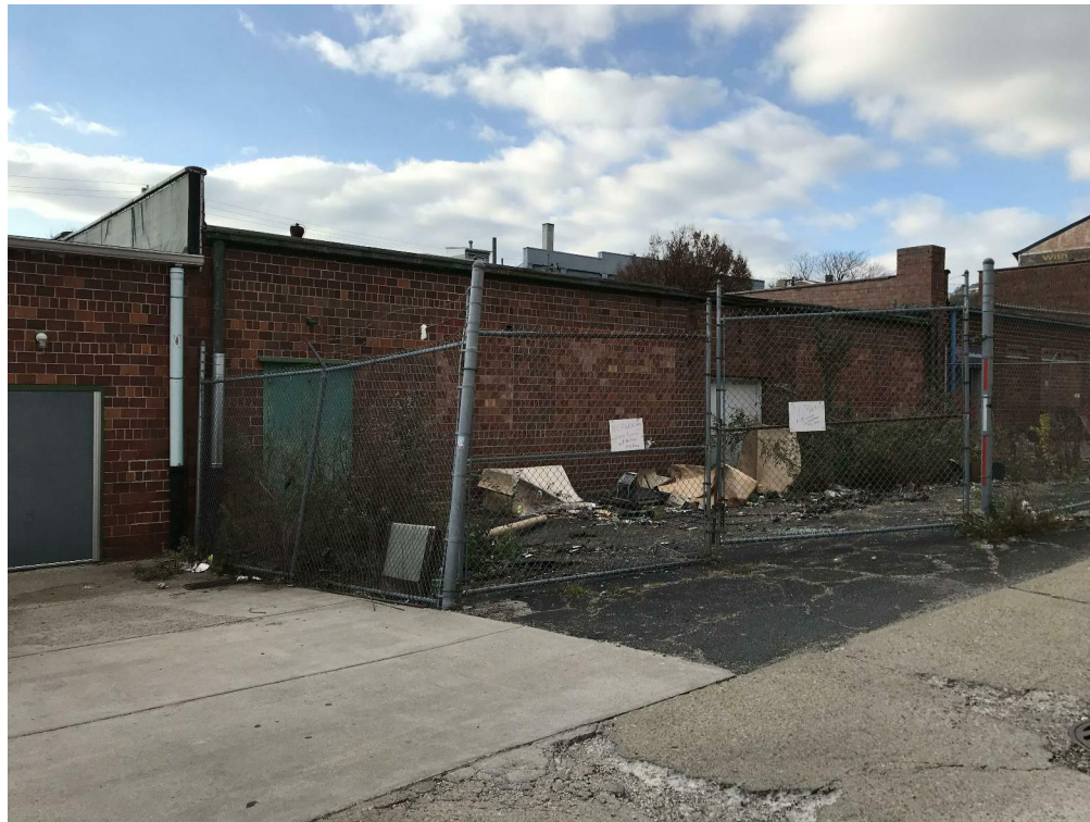
3. REAR VIEW - SE
