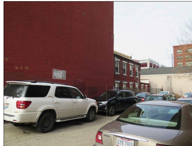
EXISTING CONDITIONS VIEW FROM COURT STREET
