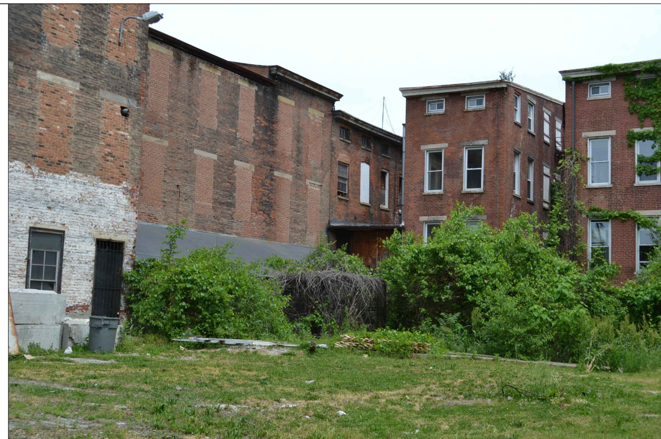
SOUTH FACADE FROM OPEN LOT
